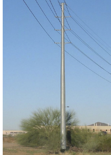
Typical 69kV double-circuit pole (left) and typical 69kV double-circuit pole with 12kV underbuild (right)
