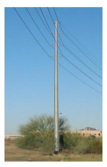
Typical 69kV double-circuit pole
