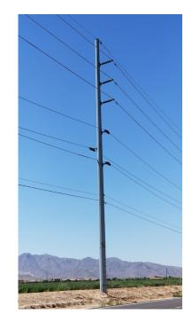
Single-circuit 69kV pole with 12kV underbuild
