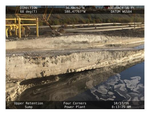
Undermining beneath the concrete ramp in the northwest corner of the Upper Retention Sump.
