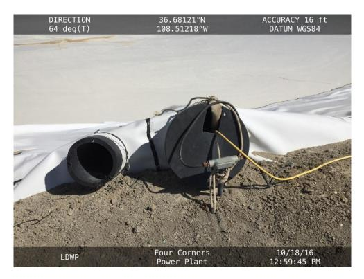
The interstitial geomembrane leak detection and evacuation pump.
