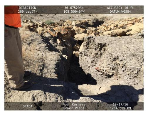
**20161017 – IMG\_1637** Erosion at the diversion channel outlet. The erosion is approximately 5 feet deep.
