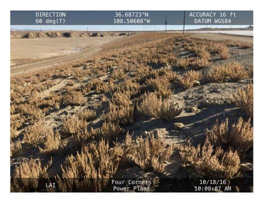
The Northwest Embankment of the LAI, facing east. The slope was regraded and drill-seeded as part of the adjacent Ash Pond 6 (left side of photo) closure.
