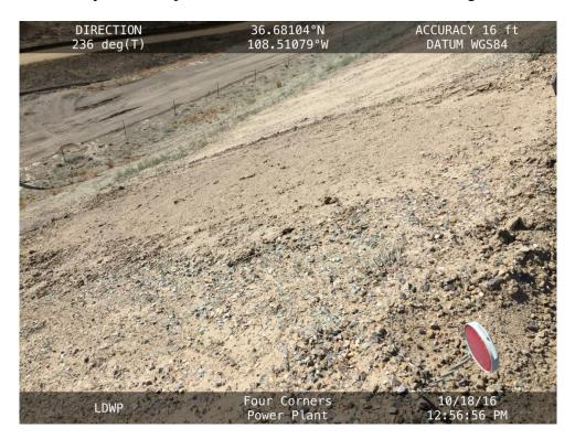
**20161018 – IMG\_1883** Area of repaired erosion along the South Embankment.
