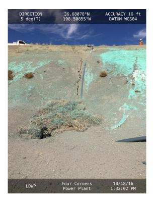
Erosion adjacent to a buried pipe for the Dead Pool Sump in the southeast corner of the LDWP.
