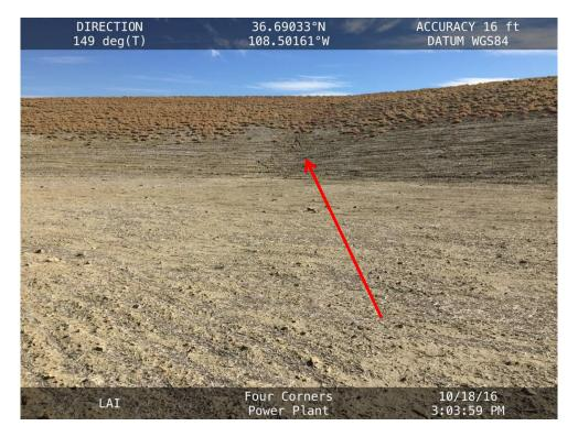
**20161018 – IMG\_1946** Erosion in the groin of the Northwest Embankment, facing south.
