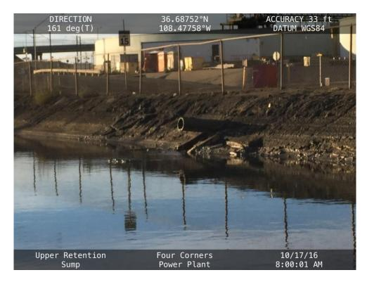
An inlet pipe along the west side of the Upper Retention Sump turned upward at a slight angle.
