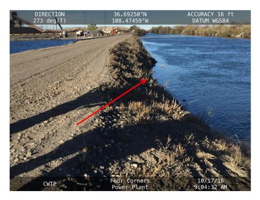
The downstream slope of the CWTP, facing west. The arrow is pointing to an oversteepened portion.
