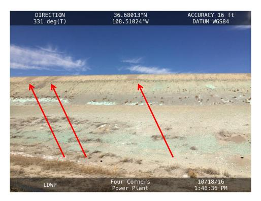
The South Embankment of the LDWP, facing north from the toe. The arrows point to locations where erosion has been repaired.
