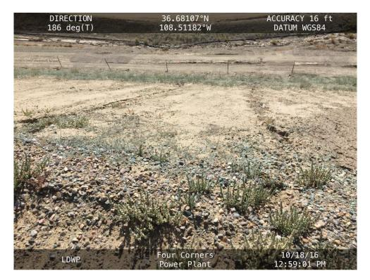
**20161018 – IMG\_1889** Areas of newer erosion rills along the LDWP South Embankment.
