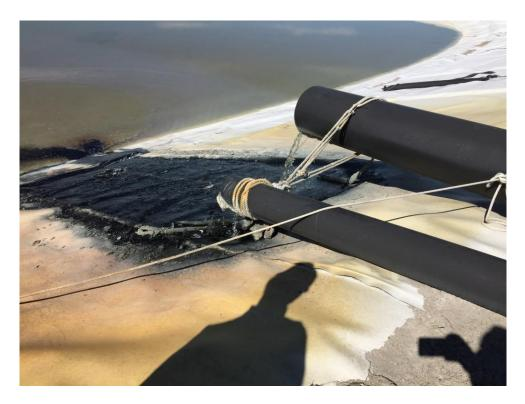
The 8-inch and 16-inch HDPE outlet pipes conveying decant water from the LAI.
