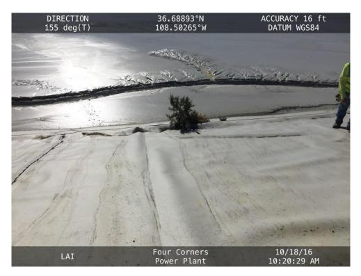
**20161018 – IMG\_1813** Vegetation growing in a liner tear along the Northwest Embankment.
