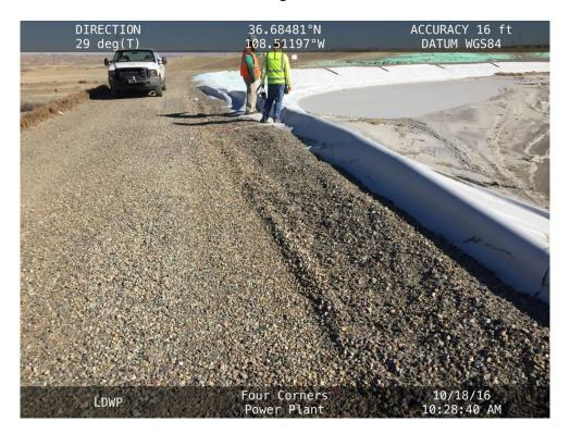
**20161018 – IMG\_1815** Anchor trench, liner pulling up in the northwest corner of the LDWP.
