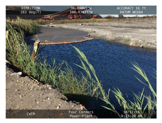
**20161017 – IMG\_1532** A decant cell in the CWTP partially filled with solids.
