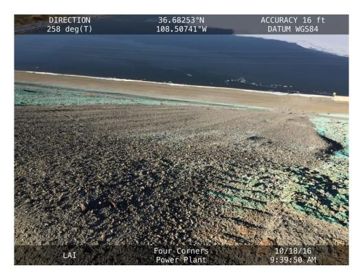
Area of erosion repair along the downstream slope of the West Embankment, facing west from the crest toward the toe and the LDWP.
