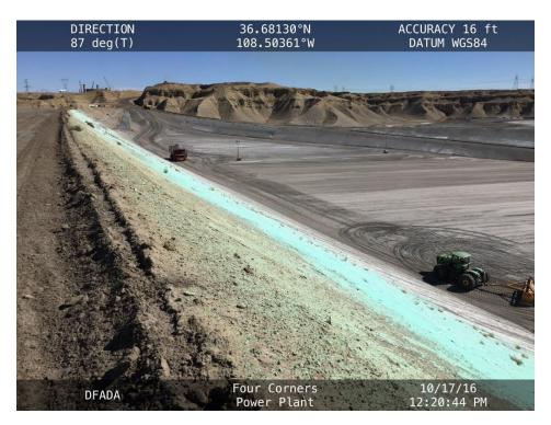
**20161017 – IMG\_1612** Ongoing CCR, ash placement in Cell 3, facing east from the South Embankment of the LAI.
