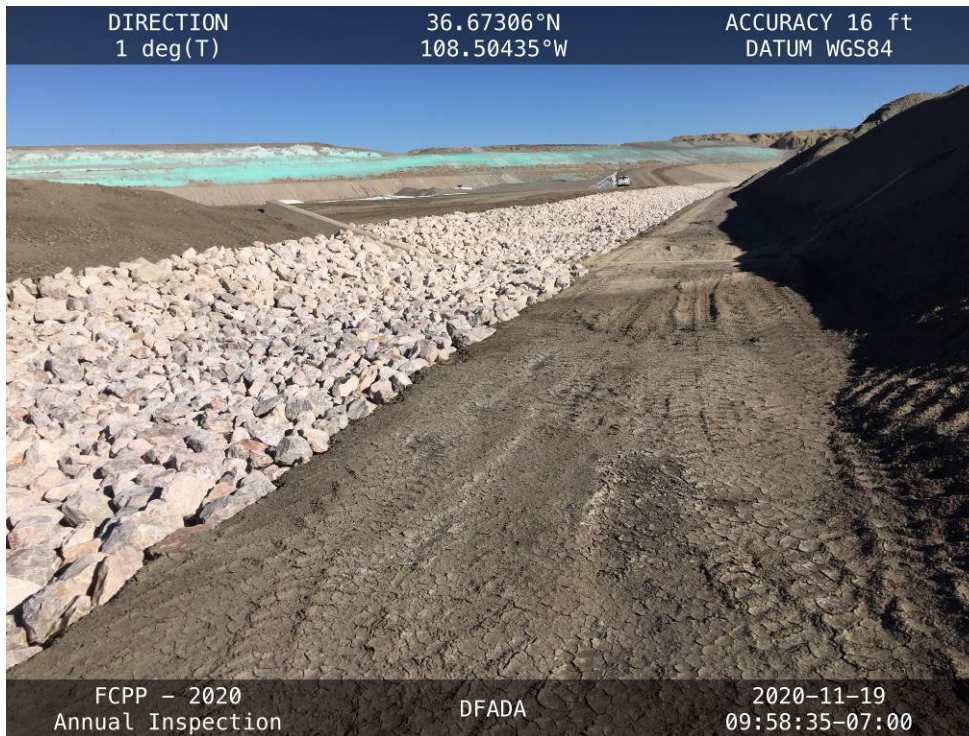
The new Stormwater Diversion Channel outlet constructed for Cell 4.
