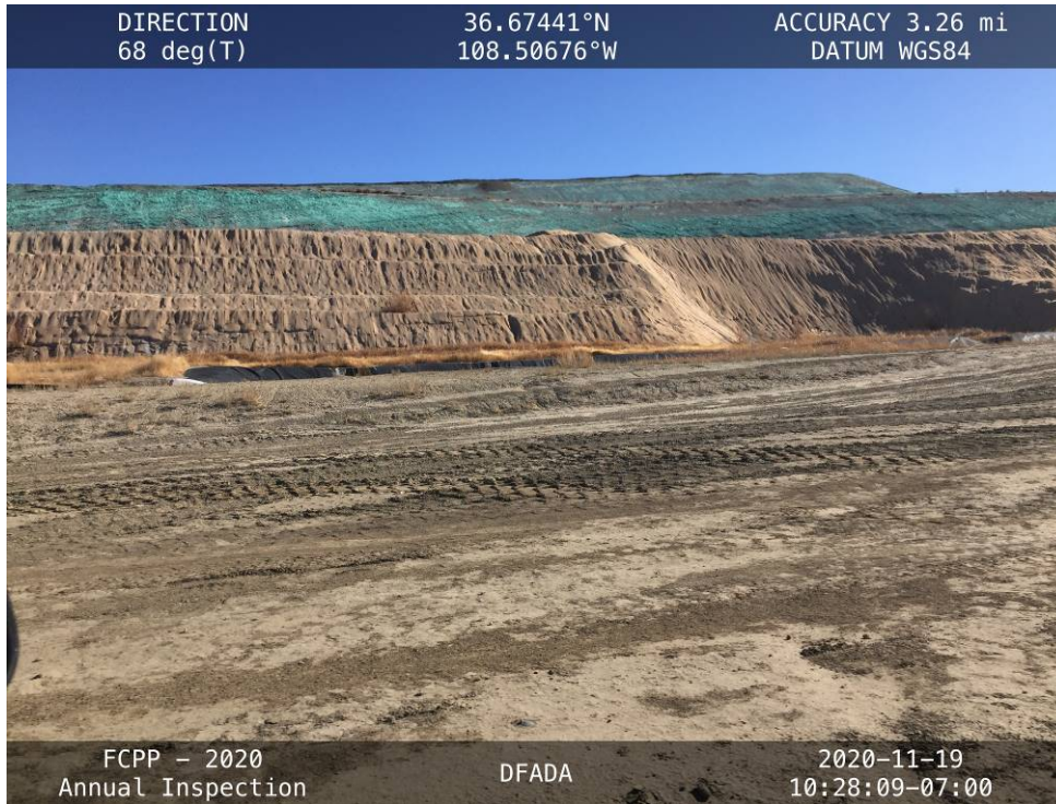
20201119 – IMG_3599 The western slope of Cell 1, facing east.
