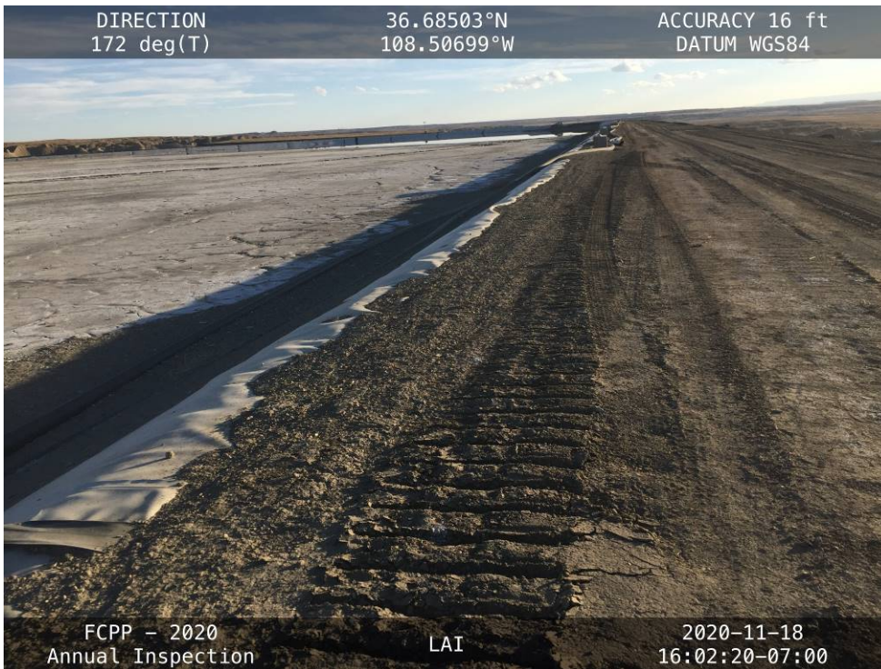
20201118 – IMG_3482 The crest of the West Embankment, facing south.
