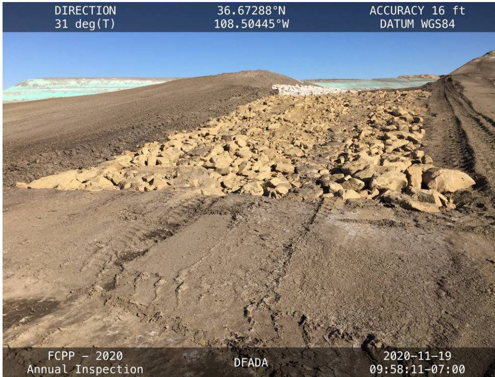
The new Stormwater Diversion Channel outlet constructed for Cell 4.
