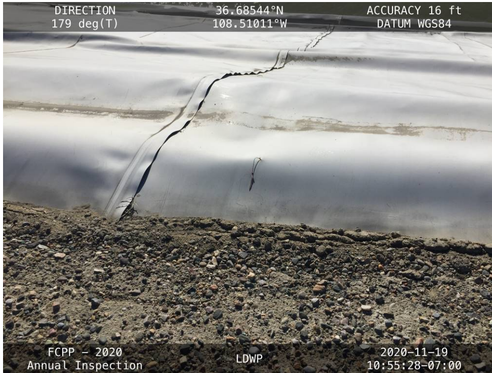
A hole in the liner along the North Embankment marked with a pin flag.
