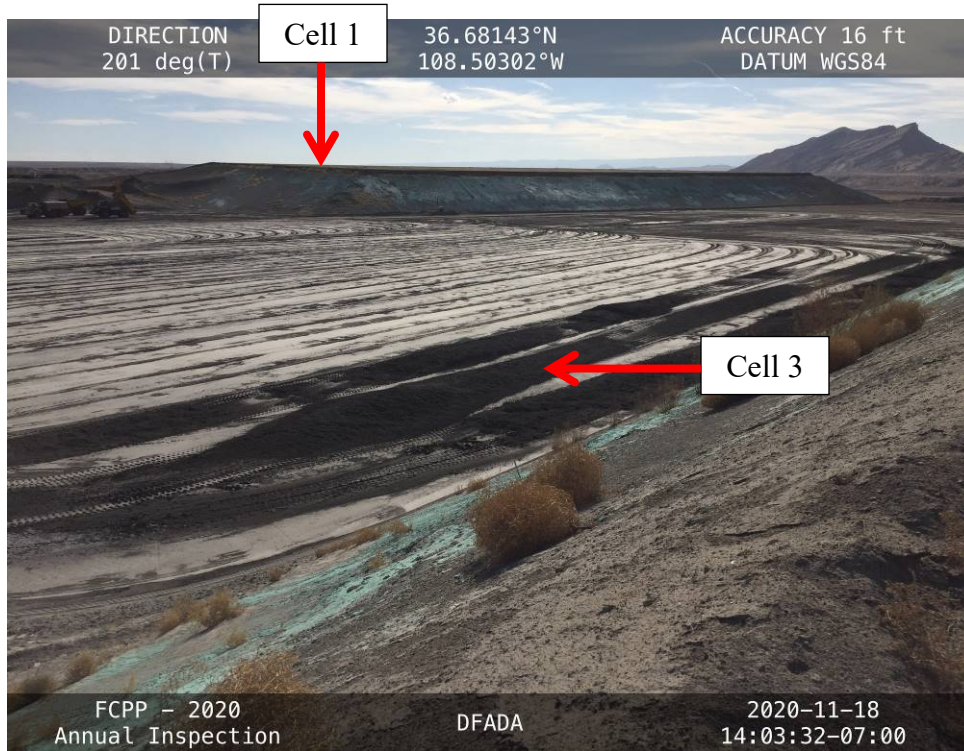
20201118 – IMG_3367 DFADA Cell 1 and the central portion of Cell 3, facing southwest.
