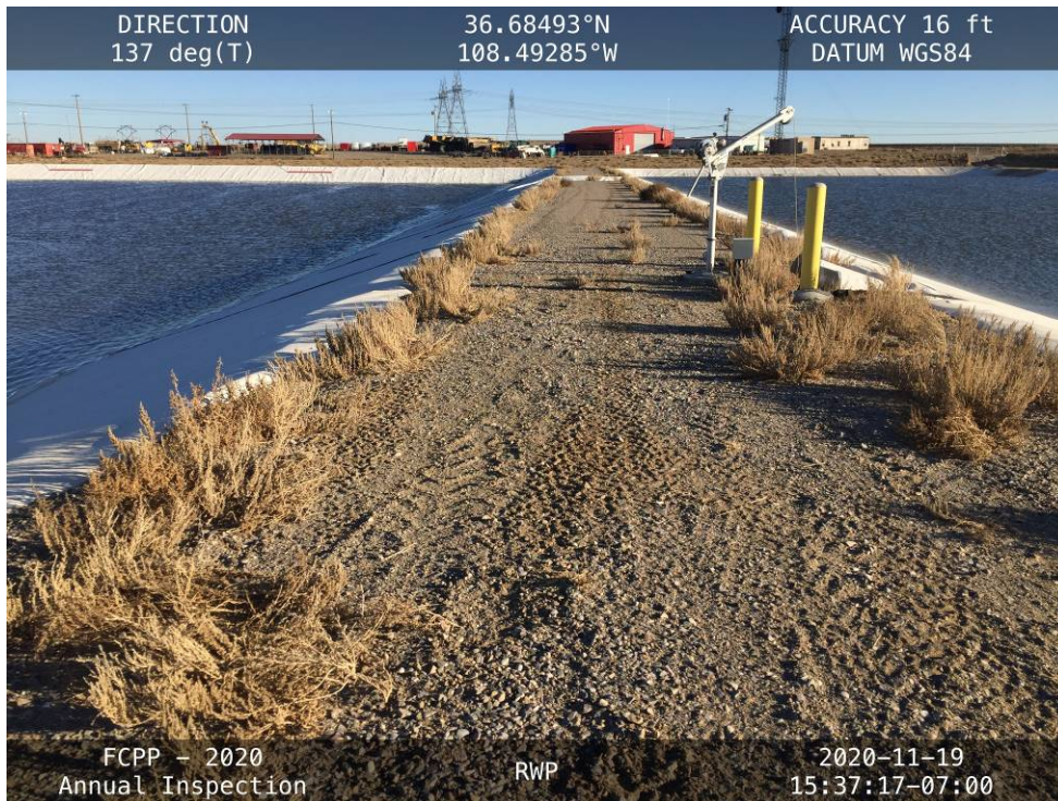
20201119 – IMG_3897 The crest of the Internal Embankment, facing southeast.
