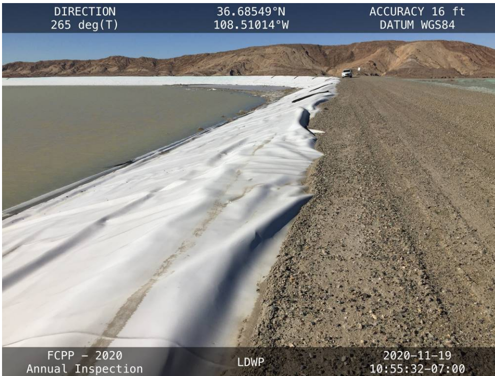
A hole in the liner along the North Embankment marked with a pin flag.
