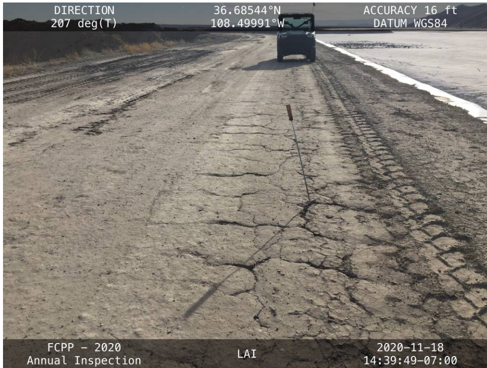
Mud cracks on the upstream side of the East Embankment crest, facing south.
