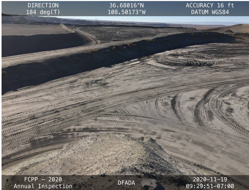
20201119 – IMG_3523 The western side DFADA Cell 2, facing south from Cell 1.
