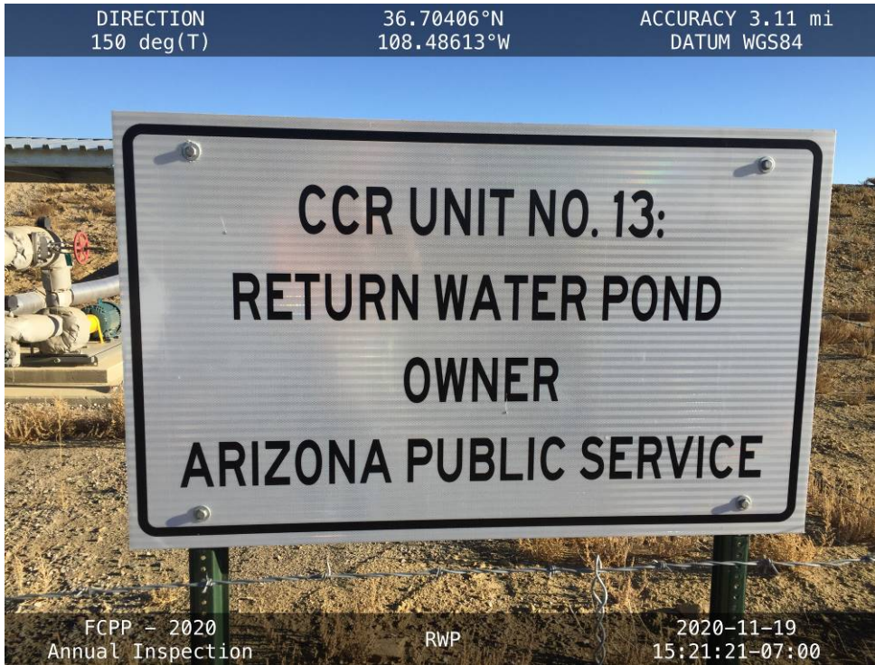
20201119 – IMG_3849 The permanent identification marker for the RWP.
