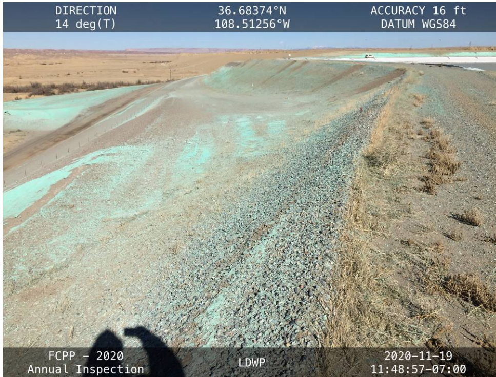
20201119 – IMG_3705 The downstream slope of the West Embankment, facing north.
