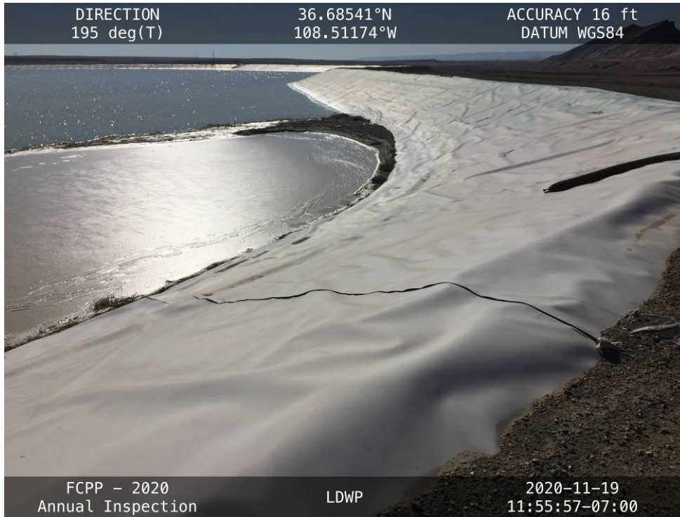
20201119 – IMG_3719 The upstream slope of the West Embankment, facing south.
