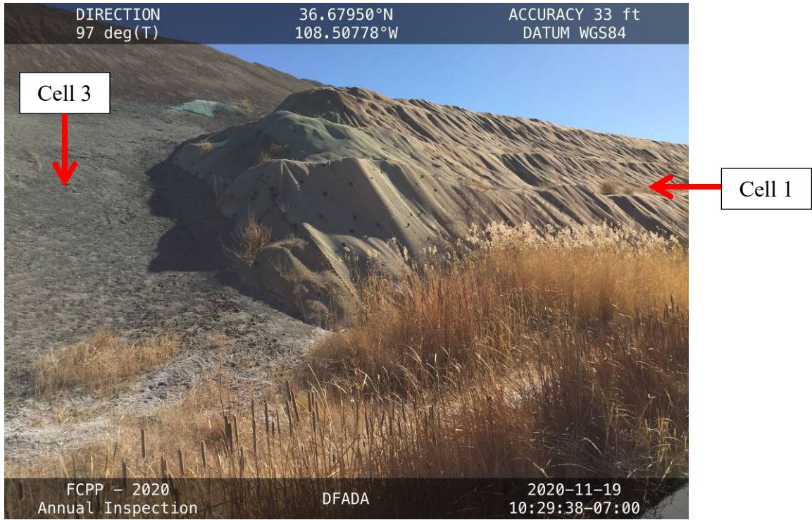
20201119 – IMG_3604 The Cell 3/Cell 1 intersection, facing east from the toe.
