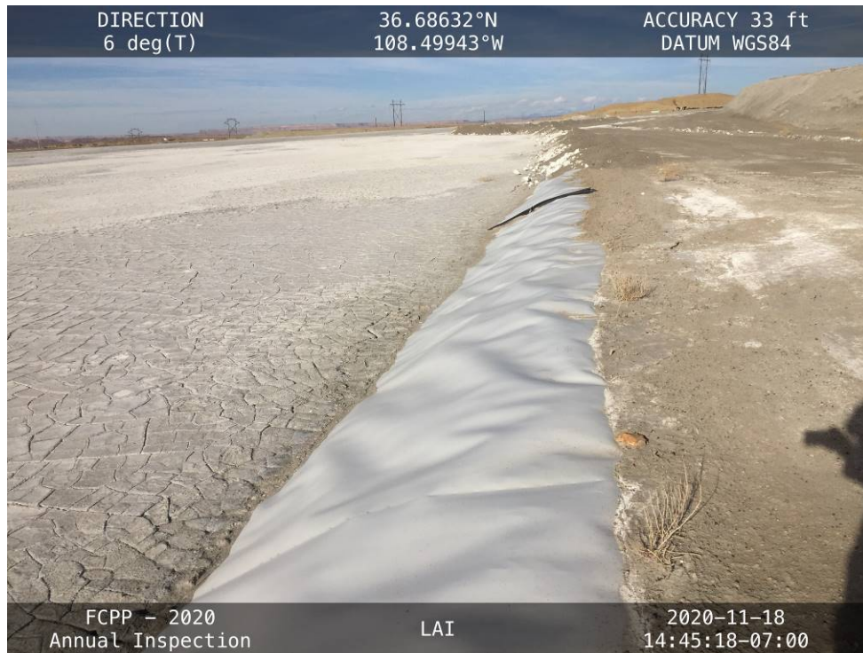
Mud cracks on the upstream side of the East Embankment crest, facing south.
