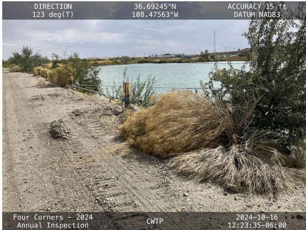
20241016 – IMG_7082 Vegetation to be removed from the upstream slope.
