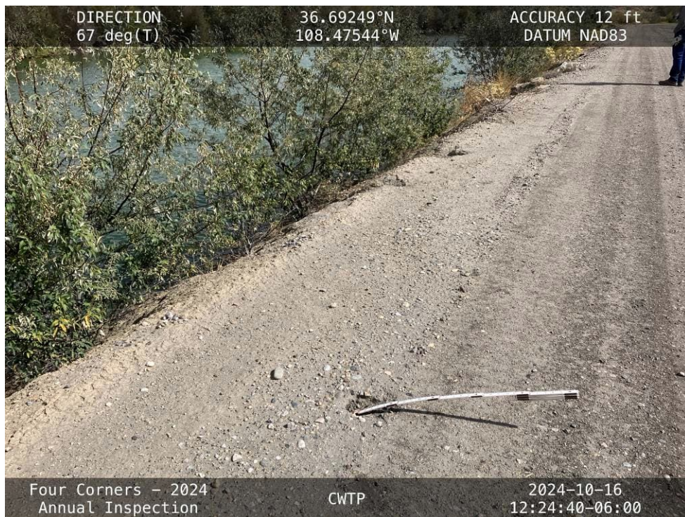
20241016 – IMG_7085 A 1-foot deep hole in the North Embankment crest.
