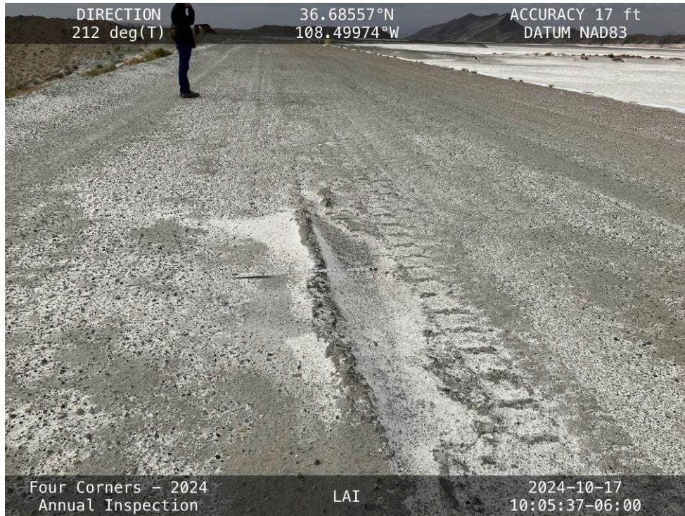
20241017 – IMG_7309 A 6-inch deep rut in the East Embankment crest.
