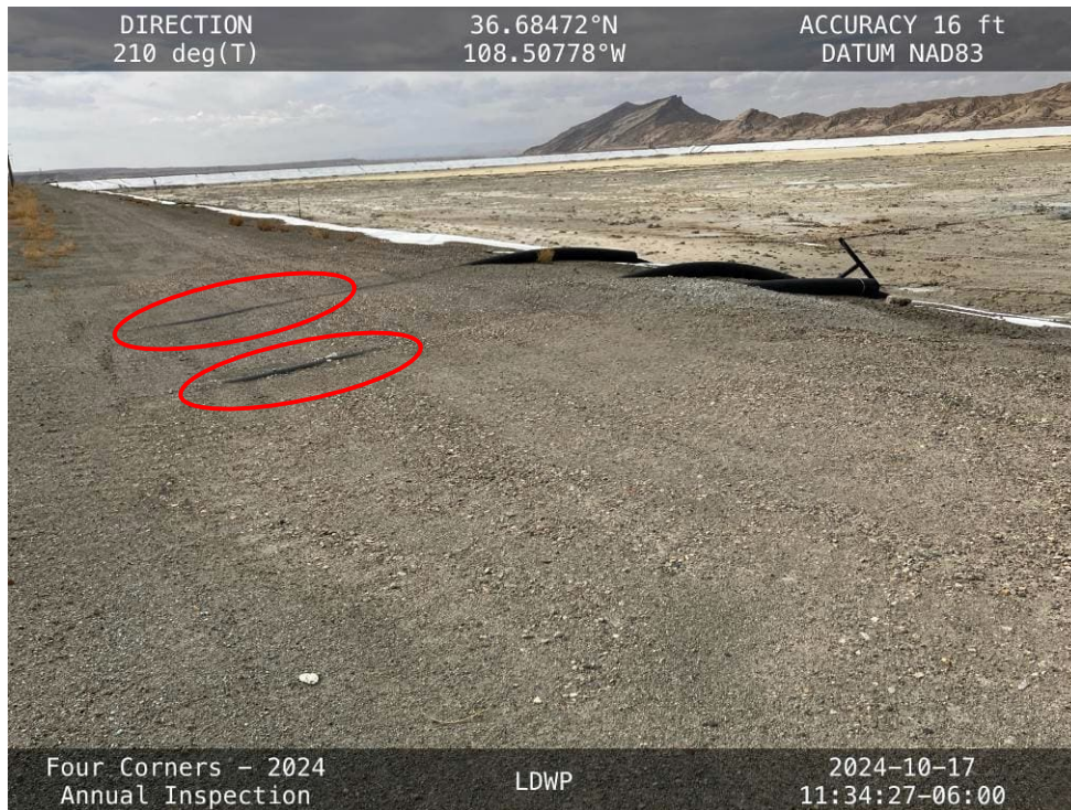
20241017 – IMG_7460 Portions of the outer pipes for the suction intake lines exposed across the East Embankment crest.
