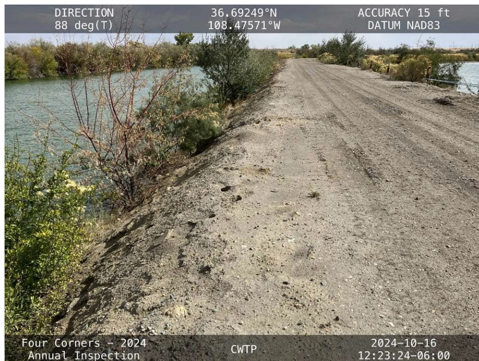
20241016 – IMG_7081 Shallow holes on the downstream shoulder of the North Embankment where depressions have been previously observed.
