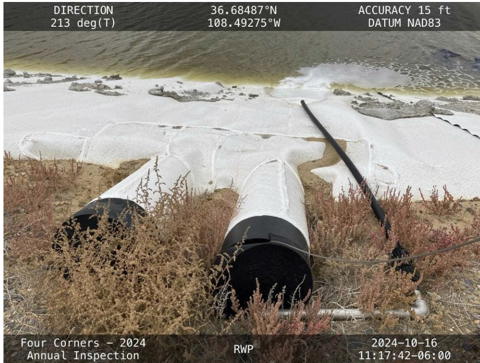
20241016 – IMG_7038 The 1.25-inch LCRS discharge pipe in the FGD cell flowing.
