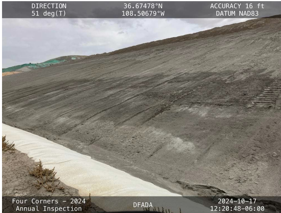
20241017 – IMG_7533 Moisture along the lower portion of the Cell 4 western slope.
