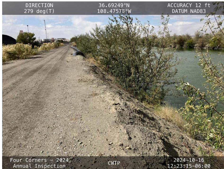
20241016 – IMG_7080 Vegetation to be removed from the downstream slope.
