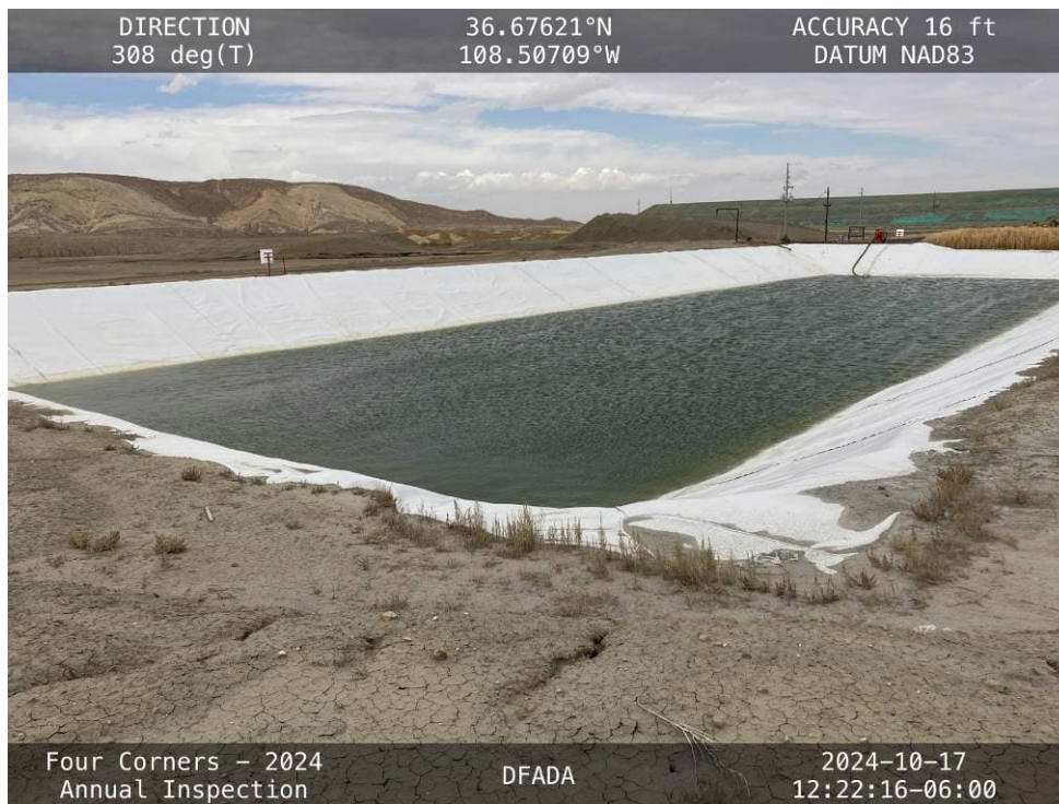
20241017 – IMG_7538 The DFADA Cell 2 leachate collection pond, facing north from its southeast corner.
