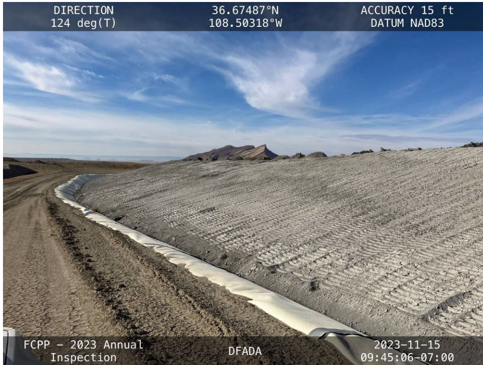
20231115 – IMG_2534 The downstream slope of Cell 4, facing southwest.
