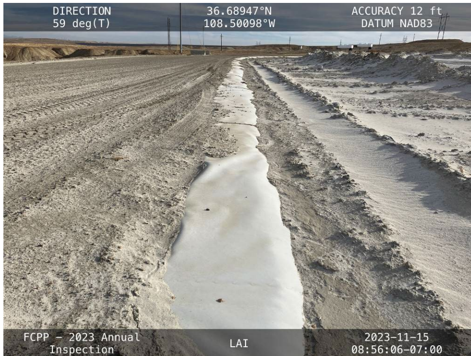
Shallow rutting and tire tracks at the Northwest Embankment access ramp.
