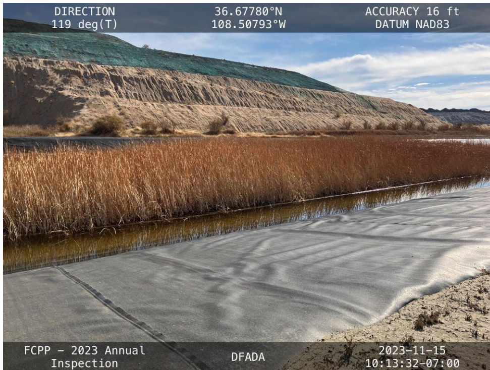
The Cell 1 leachate collection pond and middle of the western slope.
