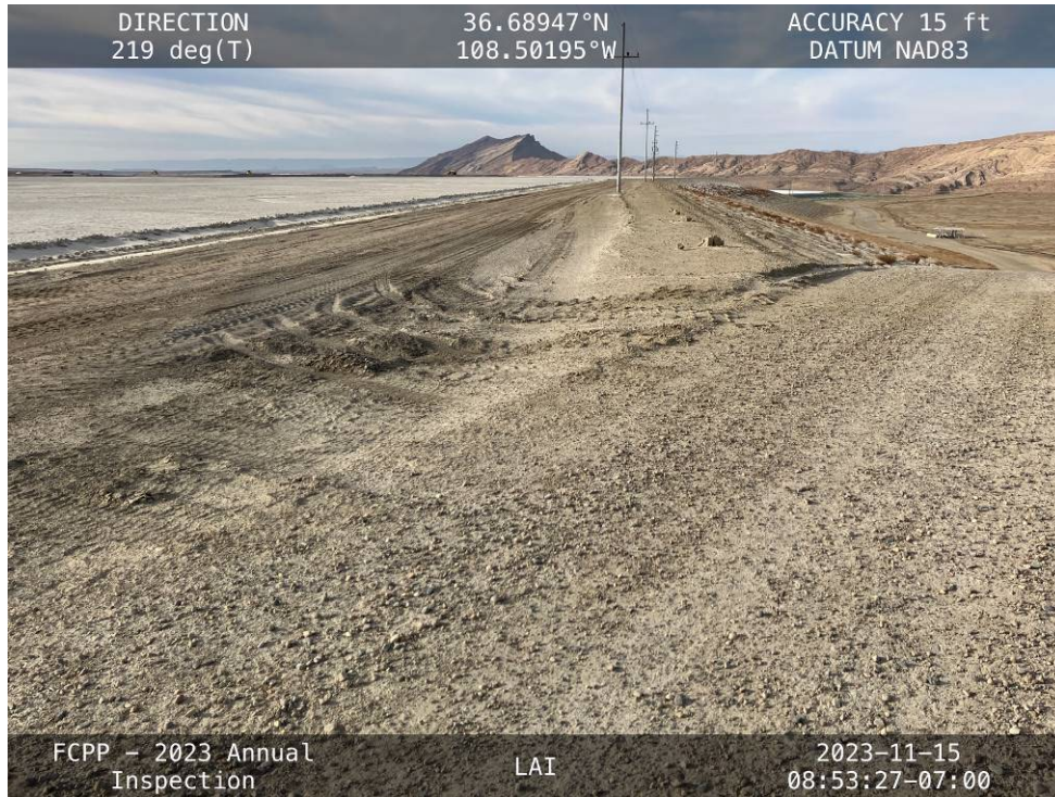
Shallow rutting and tire tracks at the Northwest Embankment access ramp.
