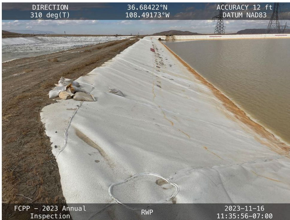
20231116 – IMG_3123 The upstream slope of the RWP Internal Embankment, facing northwest.
