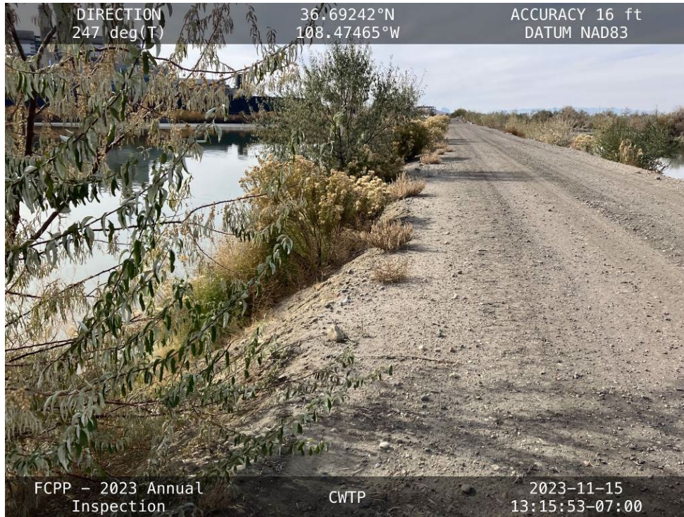
20231115 – IMG_2831 The upstream slope along the North Embankment, facing west.
