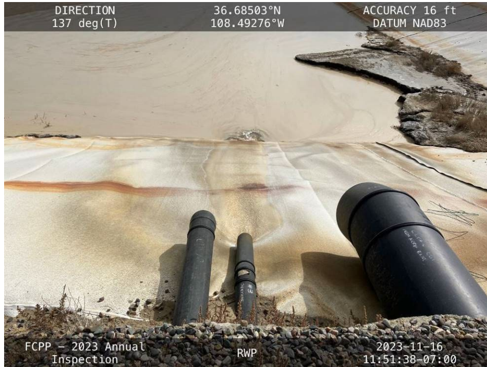
20231116 – IMG_3189 RWP cell inlet pipes.
