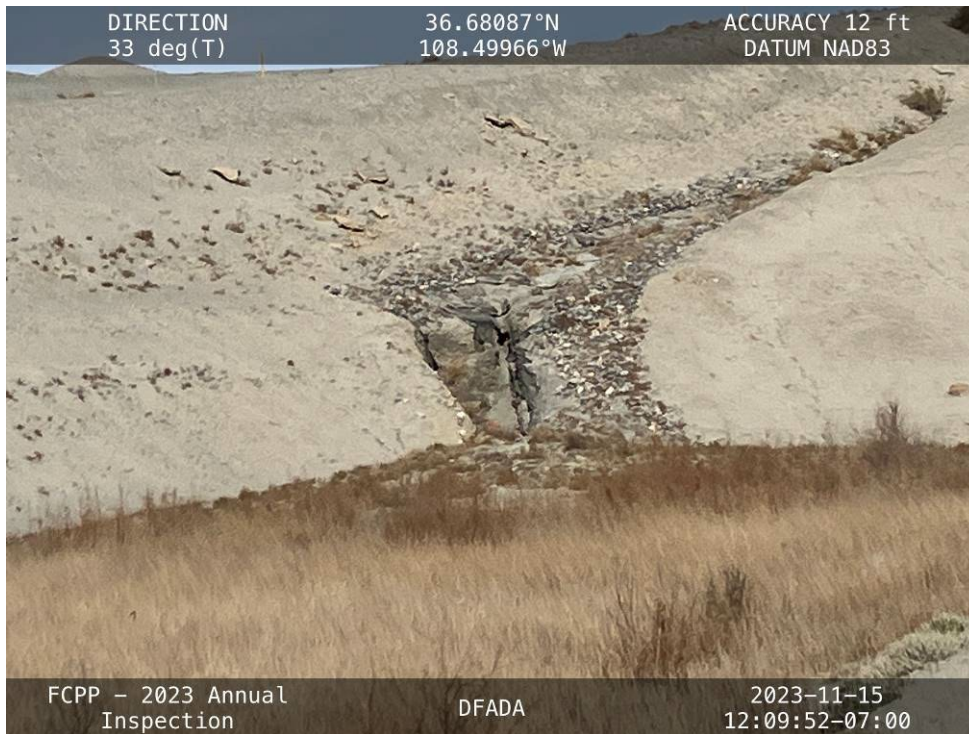
Erosion around the new outlet for the Stormwater Diversion Channel.
