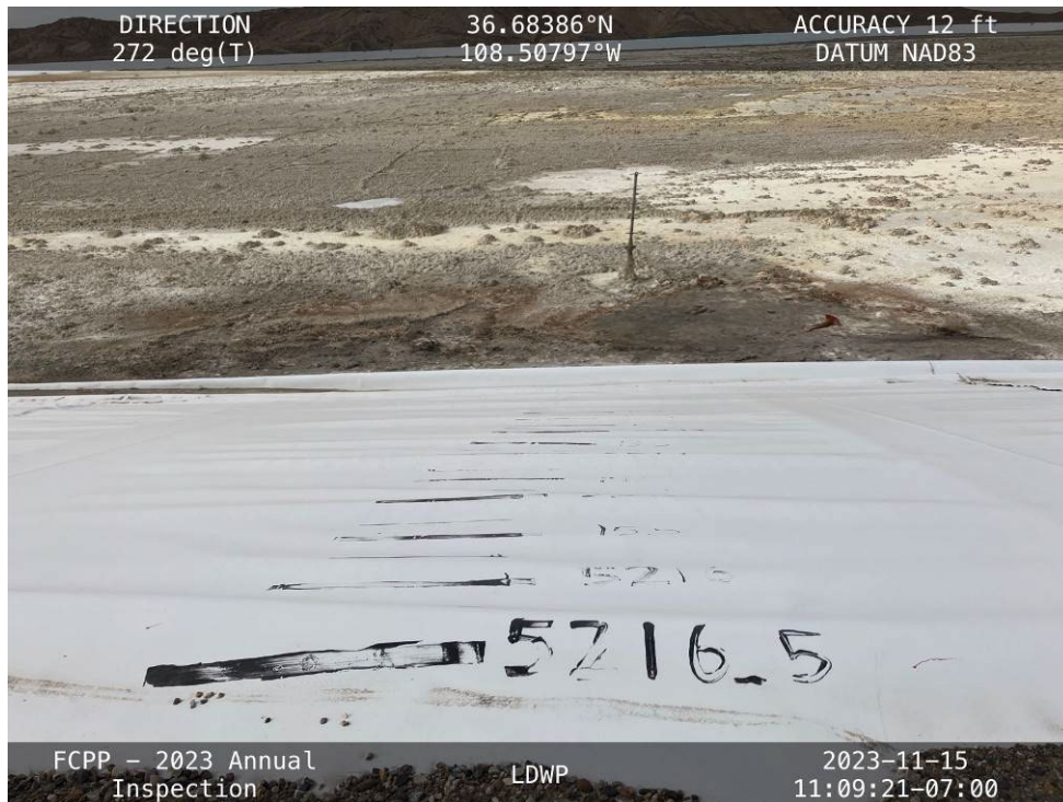
The crest of the East Embankment with ash from erosion off the LAI West Embankment, facing south.
