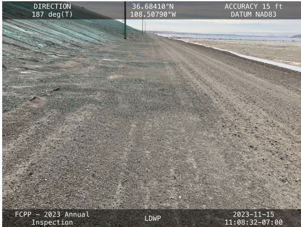
The crest of the East Embankment with ash from erosion off the LAI West Embankment, facing south.
