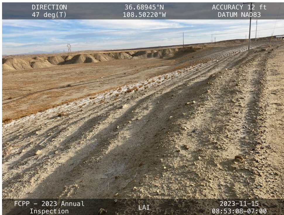
20231115 – IMG_2428 The downstream slope of the Northwest Embankment, facing northeast.
