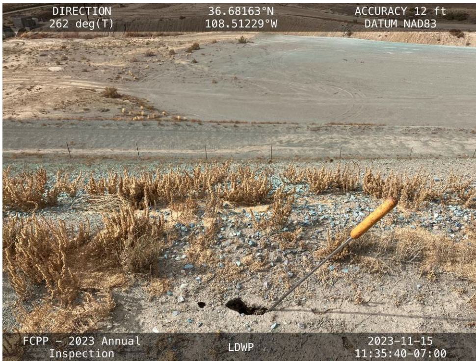
An 11-inch-deep erosion rill on downstream slope of the West Embankment.
