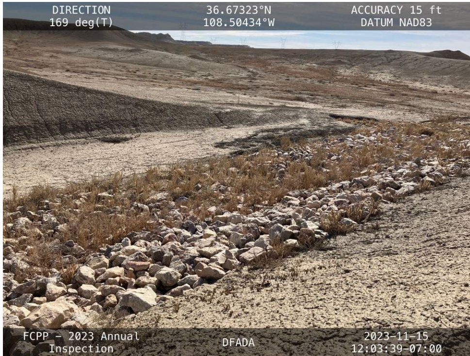
20231115 – IMG_2778 The end of the Stormwater Diversion Channel, facing south.
