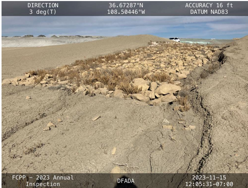
Erosion around the new outlet for the Stormwater Diversion Channel.
