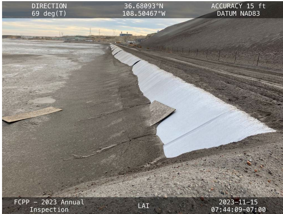
20231115 – IMG_2303 A piece of plywood along the liner, separated by a thin layer of ash.
