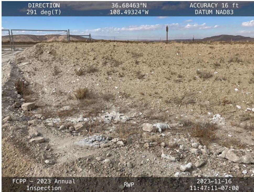
20231116 – IMG_3163 FGD spilled outside the FGD Pond during recent removal activities.
