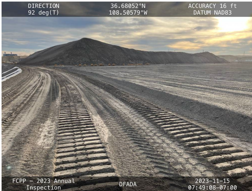
20231115 – IMG_2316 The top of Cell 3, facing east from the LAI crest.
