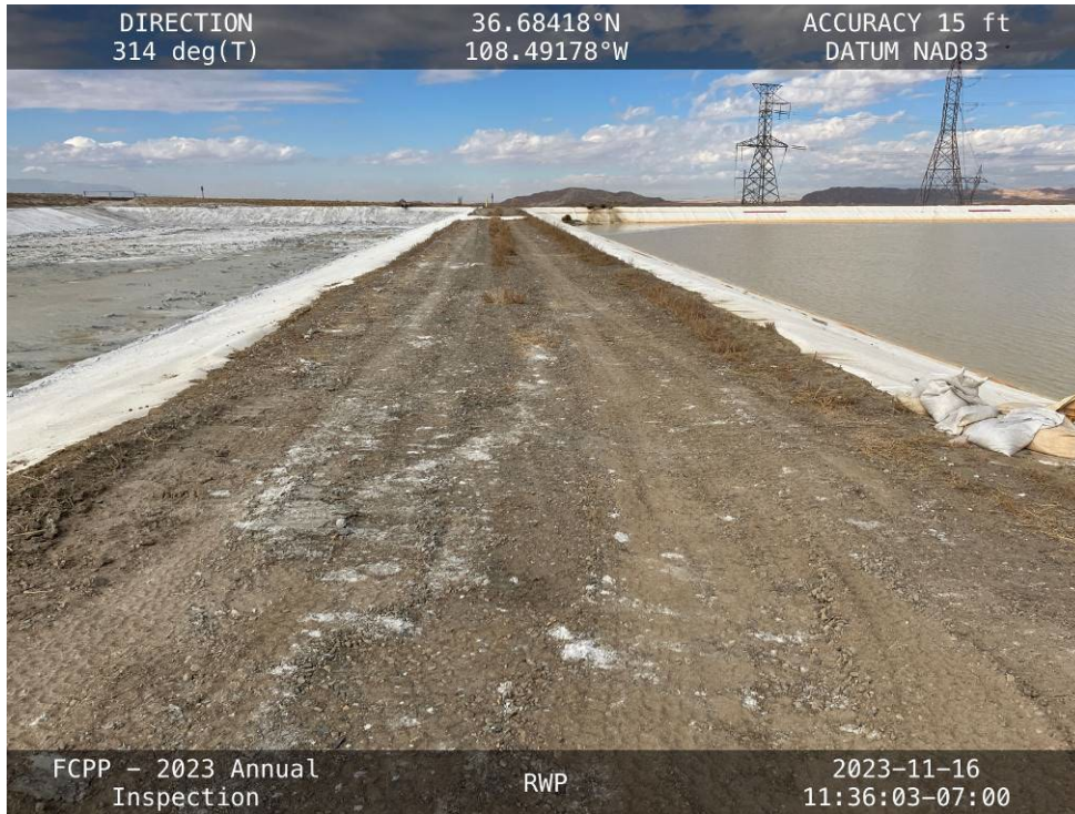
20231116 – IMG_3124 The crest of the Internal Embankment, facing northwest.
