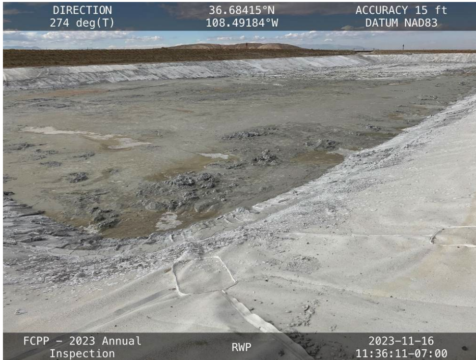
20231116 – IMG_3126 The empty FGD Pond cell, facing west.
