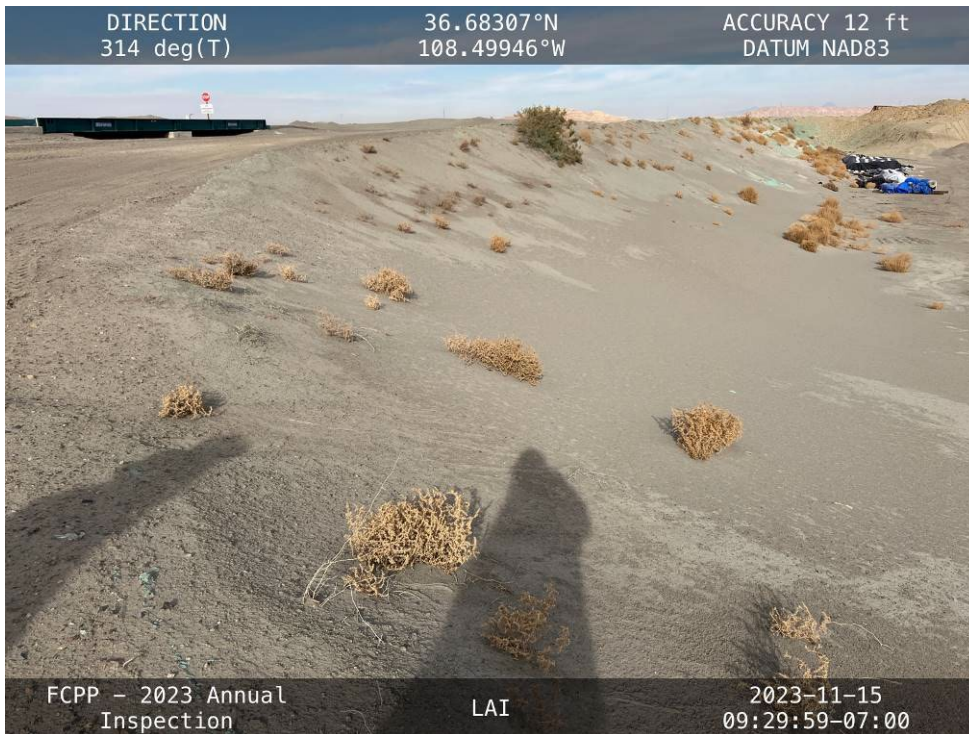
The downstream slope at the southern end of the East Embankment, with vertical scarps.
