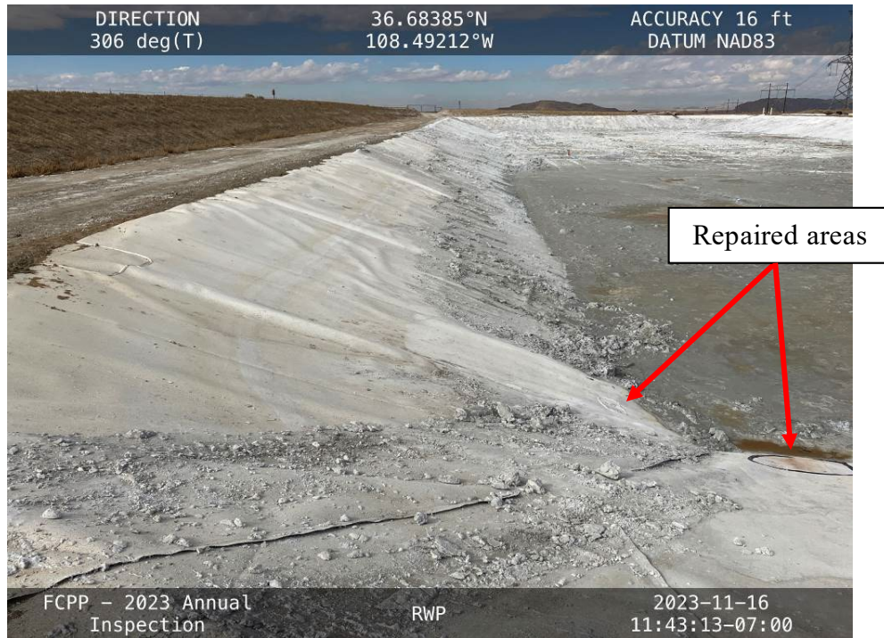
The upstream slope of the FGD Pond Southwest Embankment with two repaired areas in the foreground, facing northwest.
