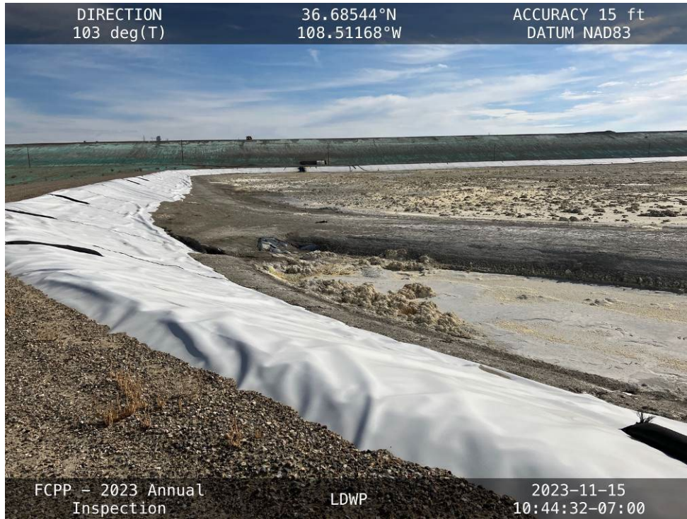
20231115 – IMG_2617 The upstream slope of the North Embankment, facing east.
