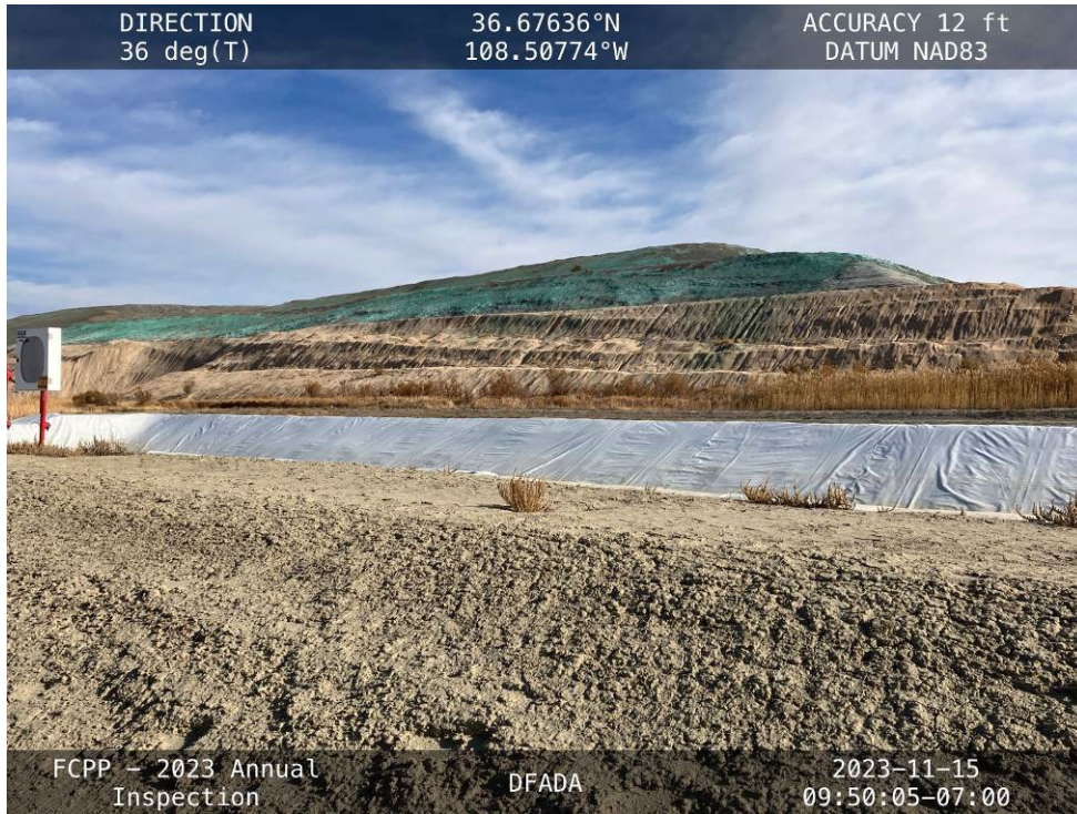
20231115 – IMG_2543 The western slope of Cell 1, facing east.
