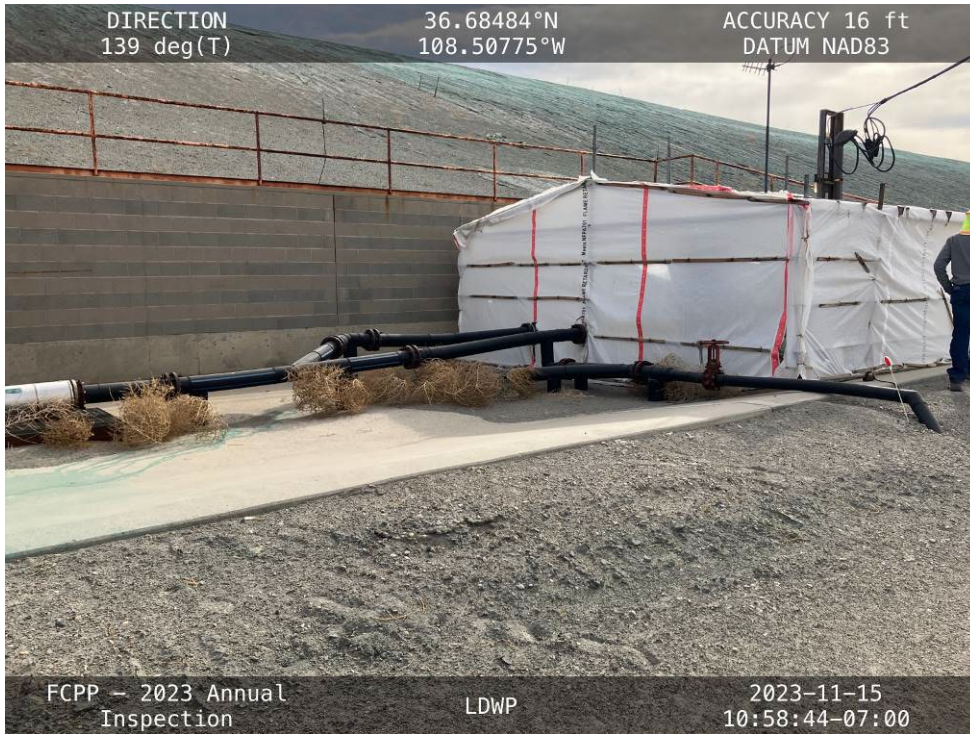
20231115 – IMG_2658 The LAI/LDWP pump station.
