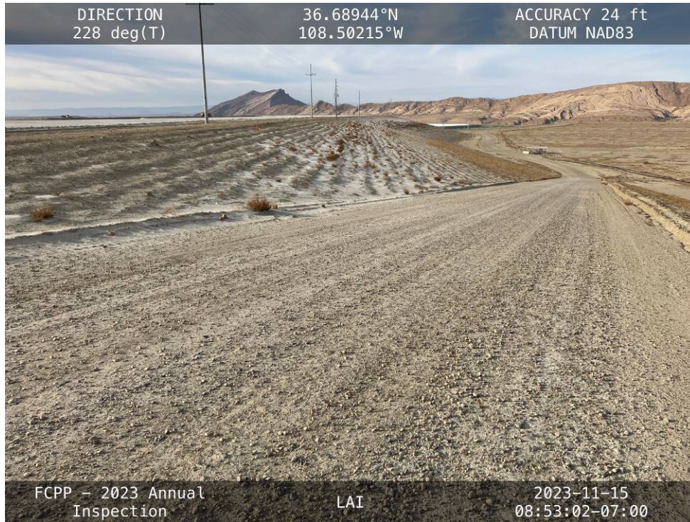
20231115 – IMG_2426 The downstream slope of the Northwest Embankment, facing west.
