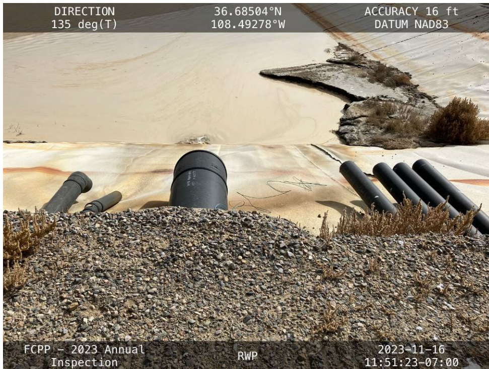
20231116 – IMG_3187 RWP cell inlet pipes.
