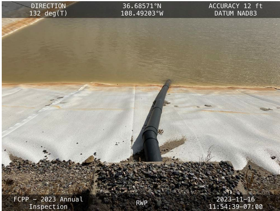
The return water pipe along the upstream slope of the Northwest Embankment.
