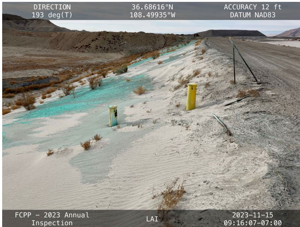
The old V-ditch and containment berm covered in FGD, facing southwest toward the reservoir.
