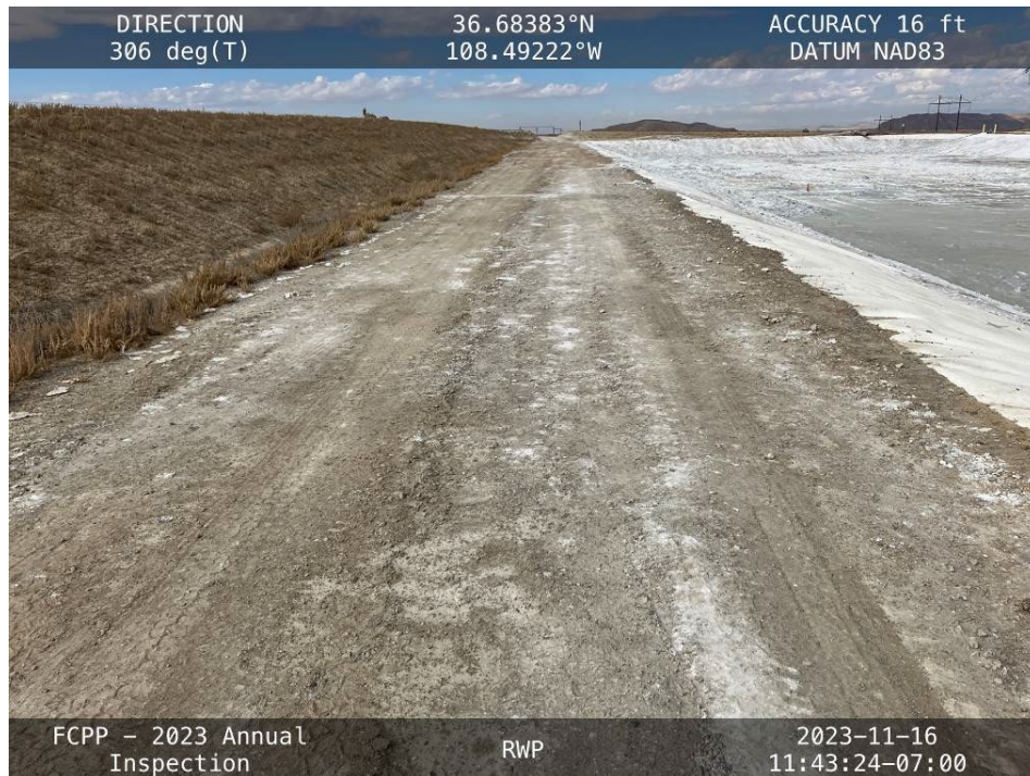
The upstream slope of the FGD Pond Southwest Embankment with two repaired areas in the foreground, facing northwest.
