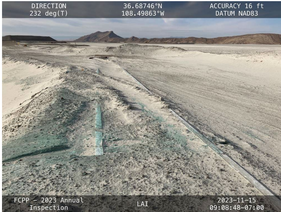
The old V-ditch and containment berm covered in FGD, facing southwest toward the reservoir.
