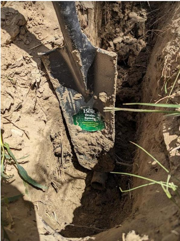
*Figure 6. Pressure Transducer Conduit.*
