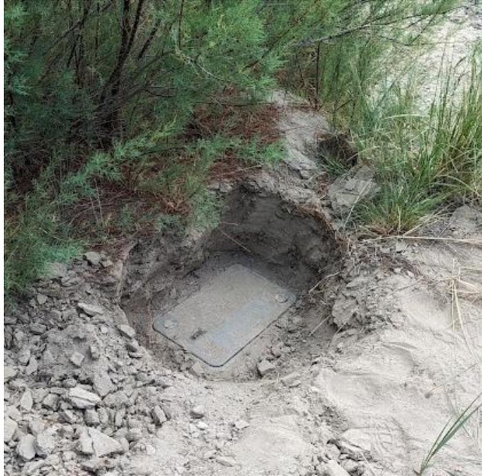
*Figure 5. Excavated Access Box.*
