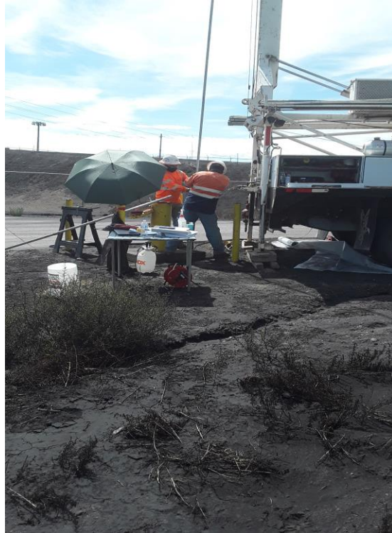
Photo 32: At CM-02. Drillers trip into well on 7/11/2020.
