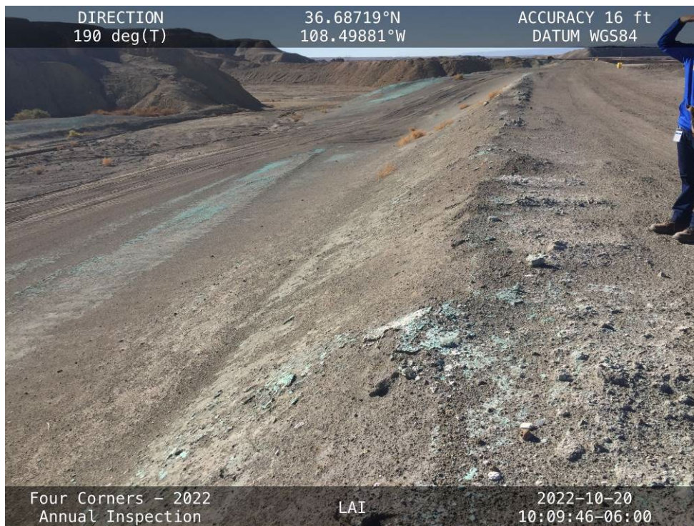
Bottom ash built up near the old V-ditch to contain the stormwater run-on.
