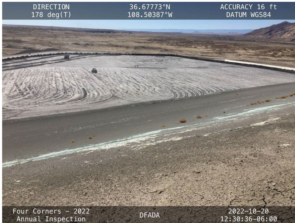
20221020 – IMG_4724 Cell 4, facing south from the southwest corner of Cell 1.
