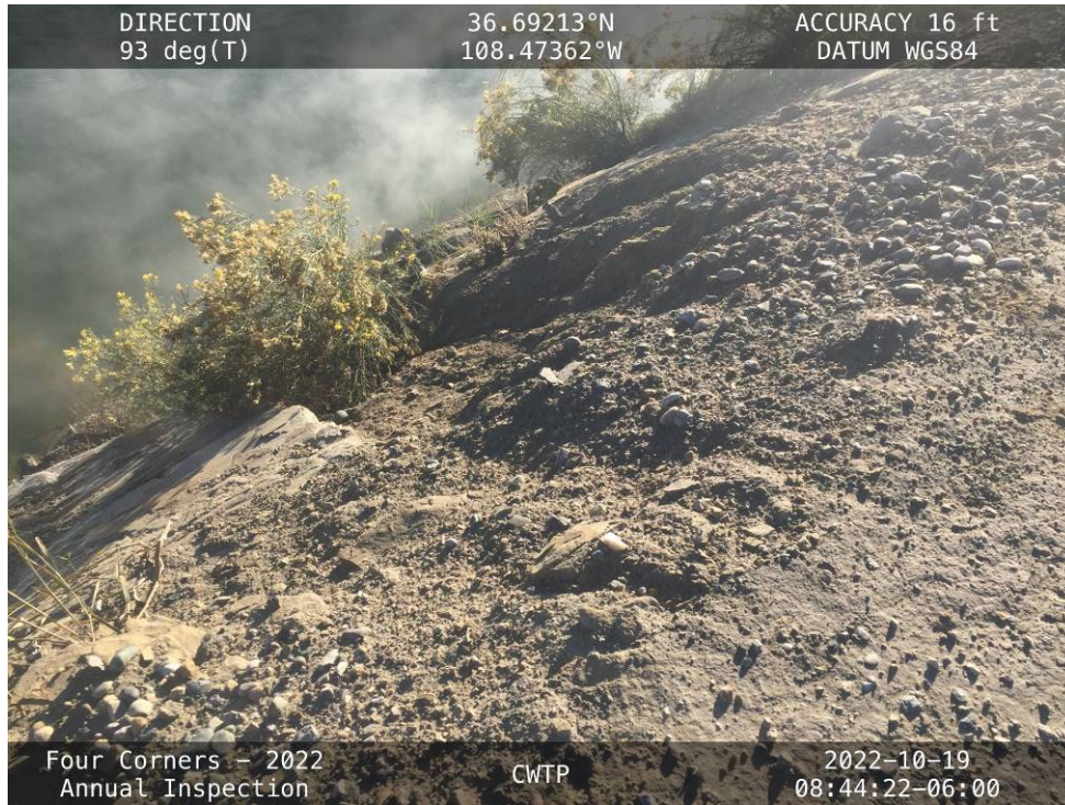
Erosion around riprap boulders along the downstream slope of the East Embankment.
