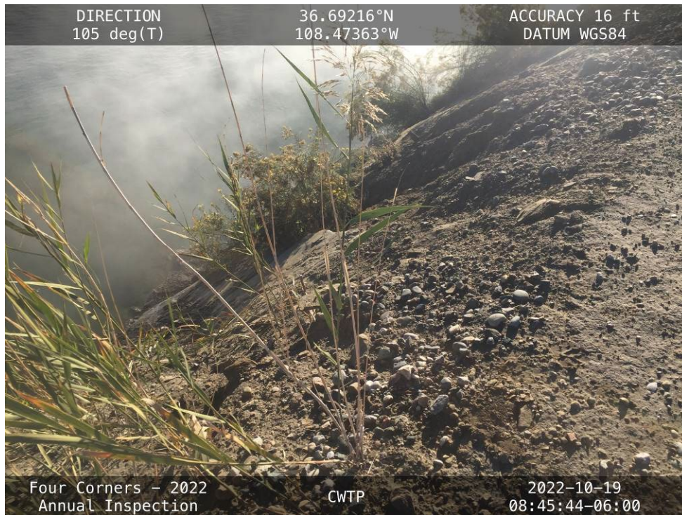
Erosion around riprap boulders along the downstream slope of the East Embankment.
