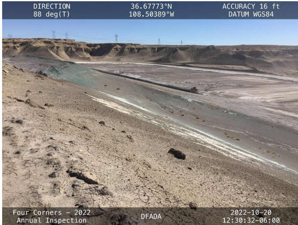
20221020 – IMG_4721 Cell 4, facing east from the southwest corner of Cell 1.
