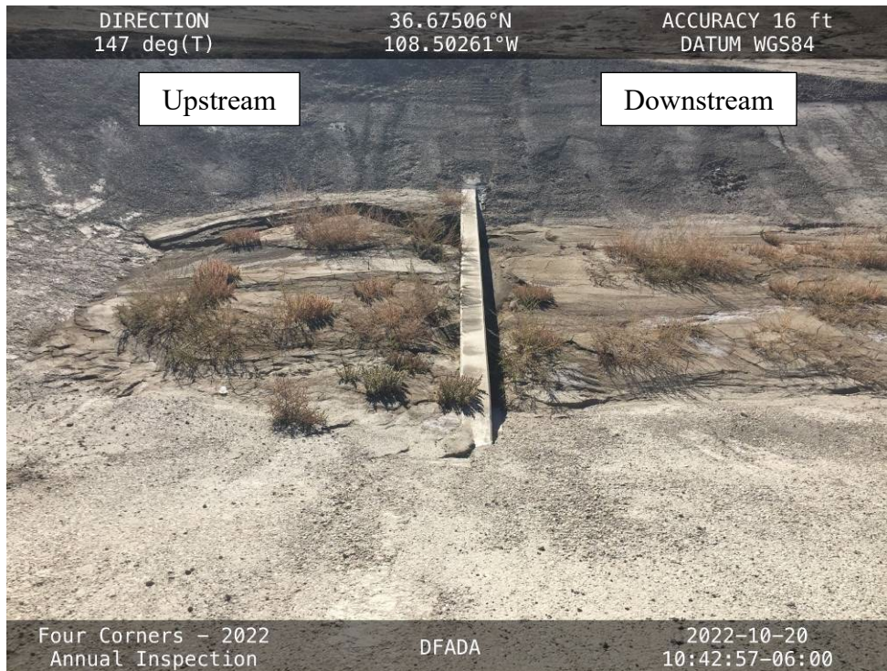
The new concrete weir wall in the new stilling basin with sediment on both sides.
