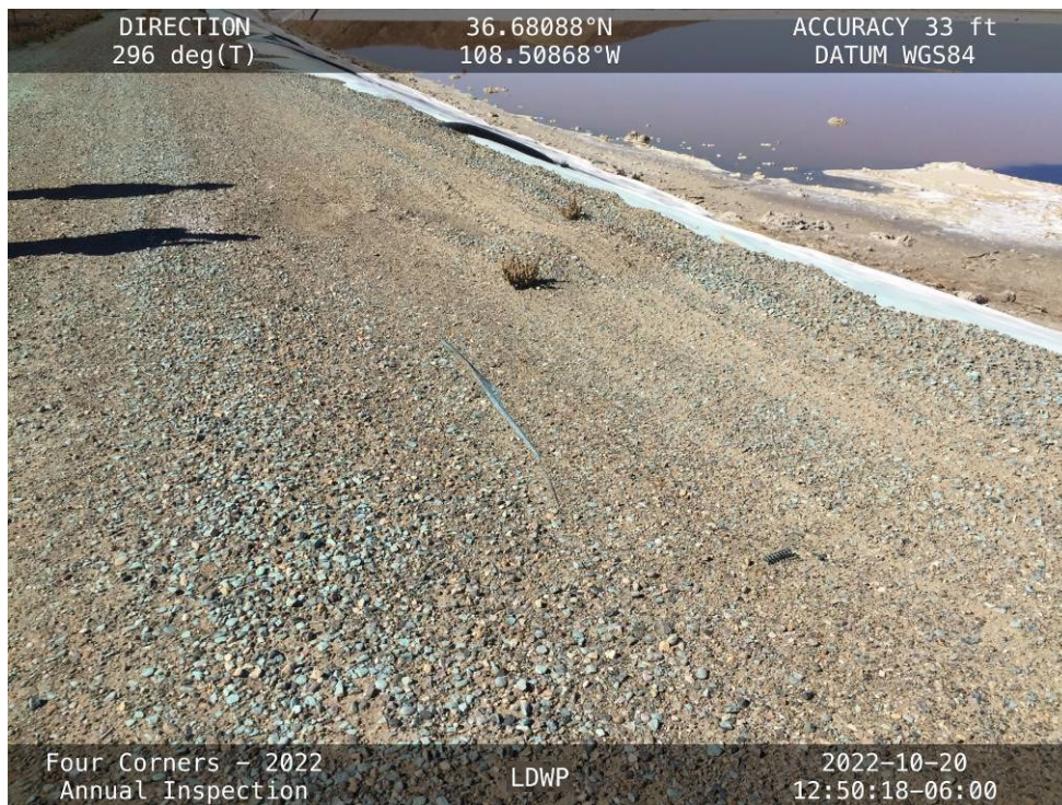
Erosion rills forming on the downstream slope in the upper half of the South Embankment.
