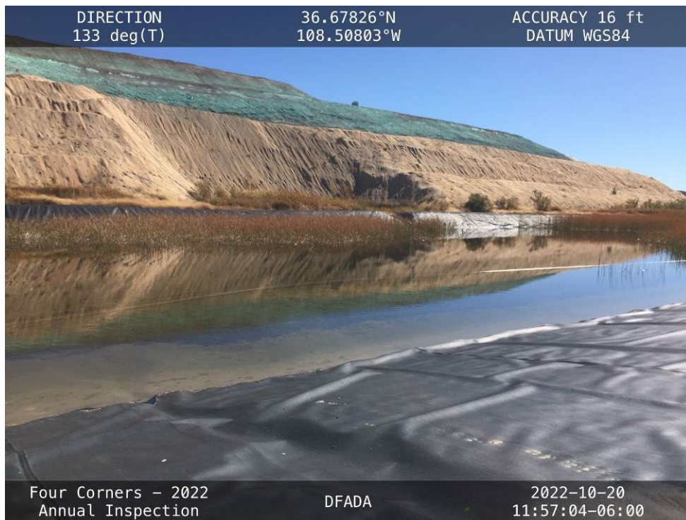
20221020 – IMG_4689 The Cell 1 leachate collection pond and western slope.
