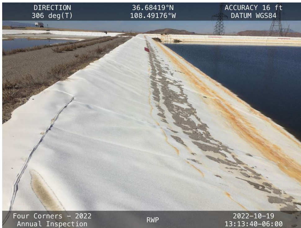
20221019 – IMG_4339 The upstream slope of the RWP Internal Embankment, facing northwest.
