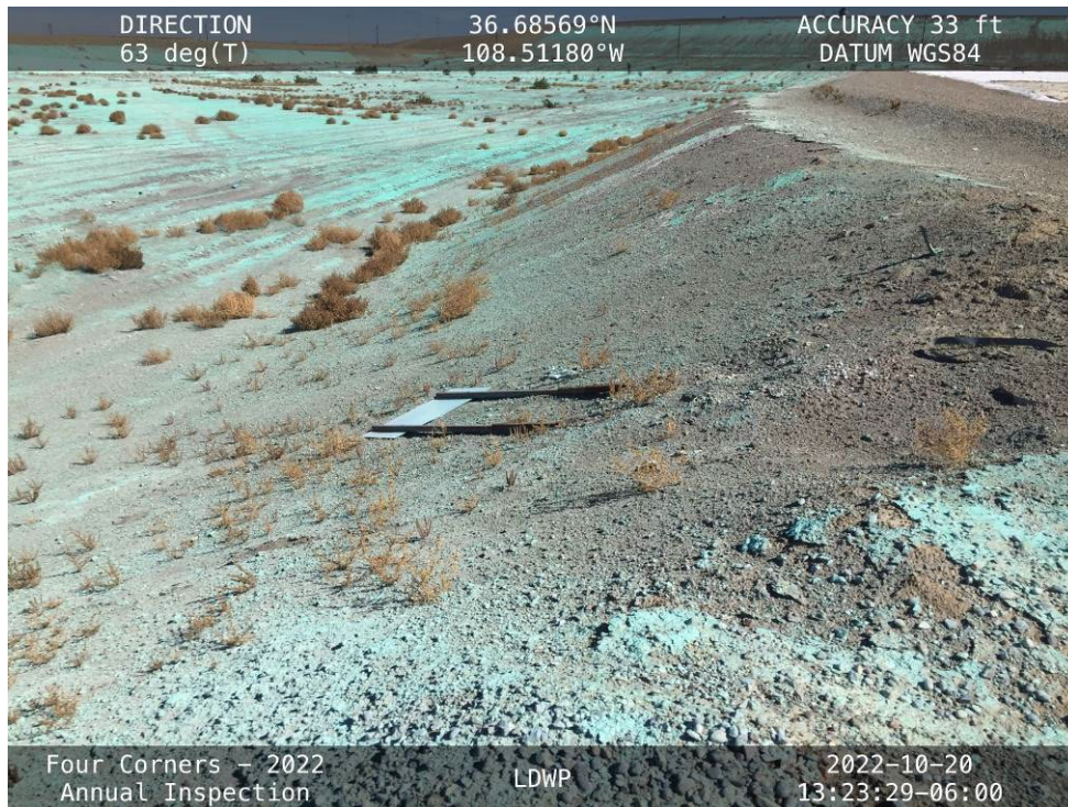
20221020 – IMG_4805 The sign for the CCR unit, to be re-erected.
