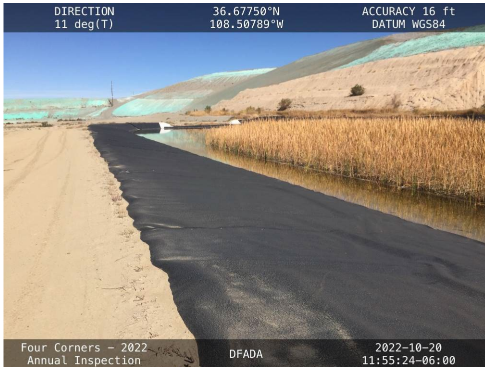
20221020 – IMG_4687 The Cell 1 leachate collection pond and western slope.
