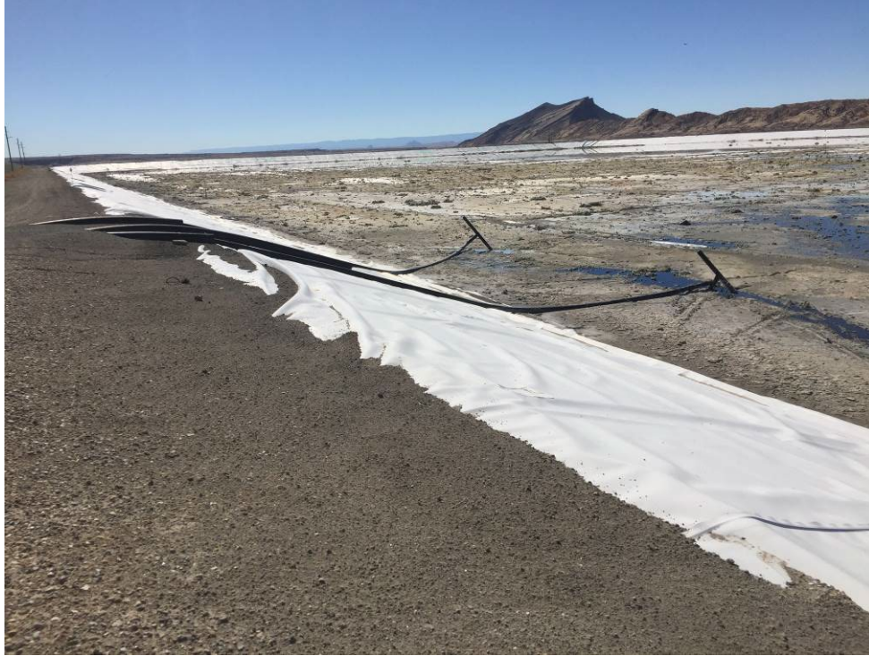
20221020 – IMG_4829 The suction intake lines in the northeast corner of the LDWP.
