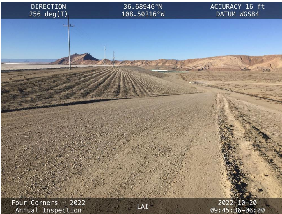
20221020 – IMG_4509 The downstream slope of the Northwest Embankment, facing west.
