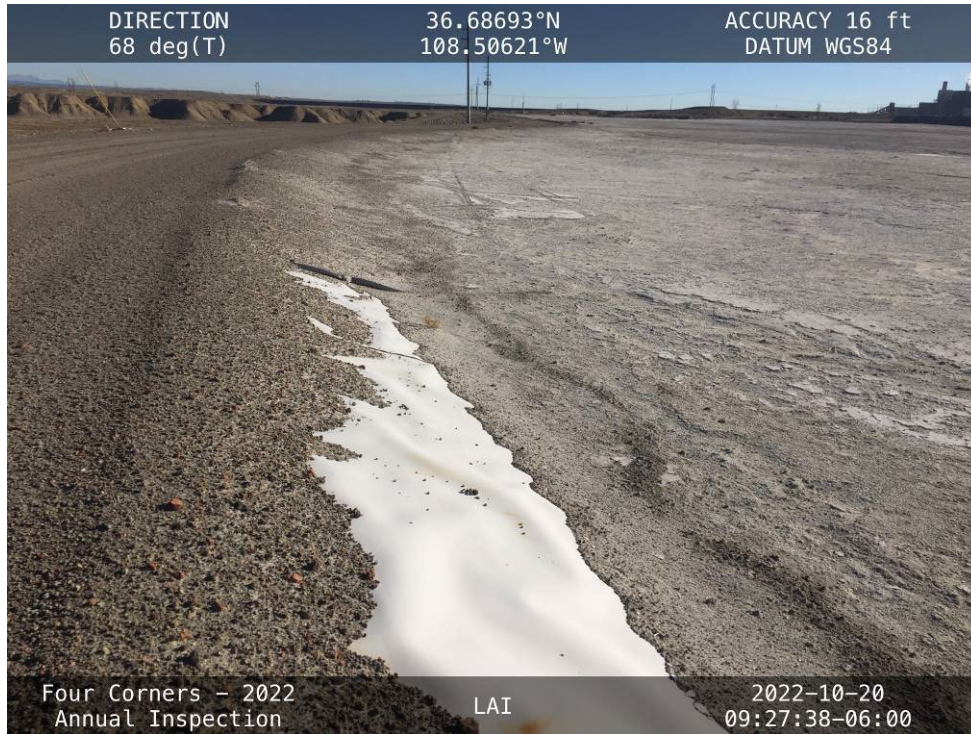
The impounded ash level nearly at the crest of the Northwest Embankment, facing northeast.
