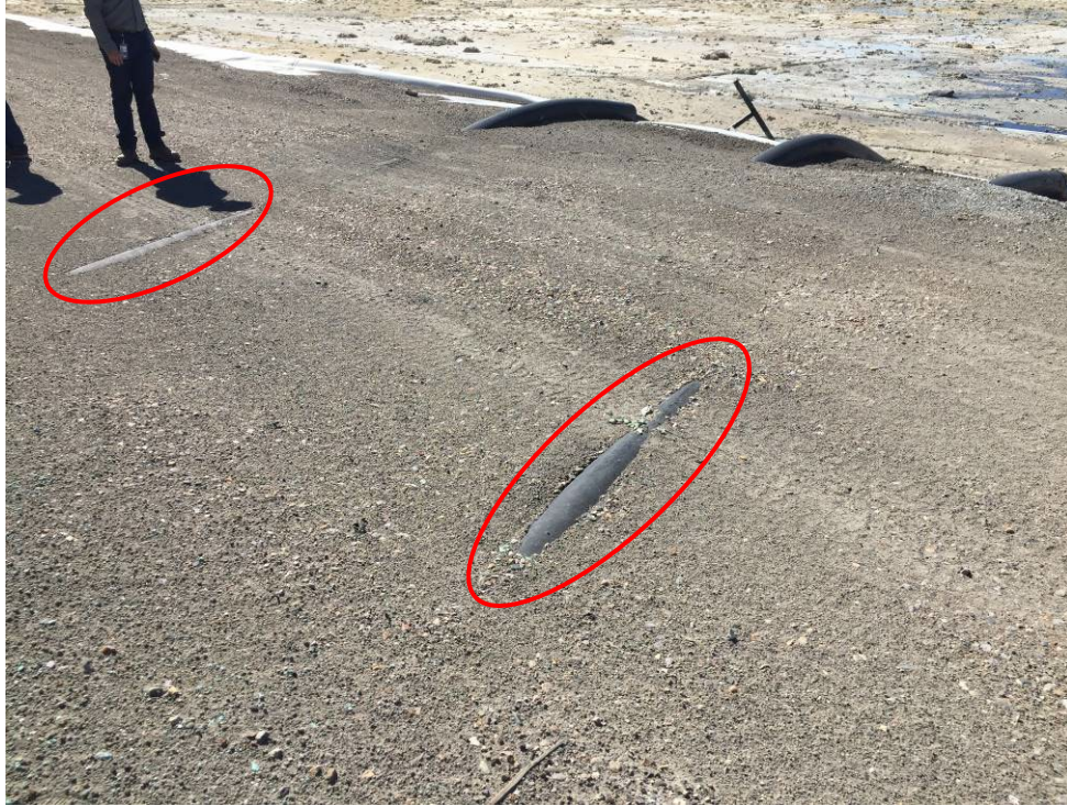
Portions of the outer pipes for the suction intake lines exposed across the East Embankment crest.
