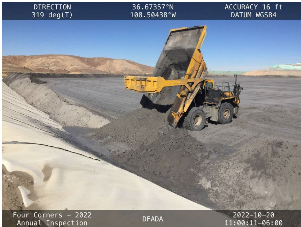
20221020 – IMG_4625 APS placing ash in Cell 4.
