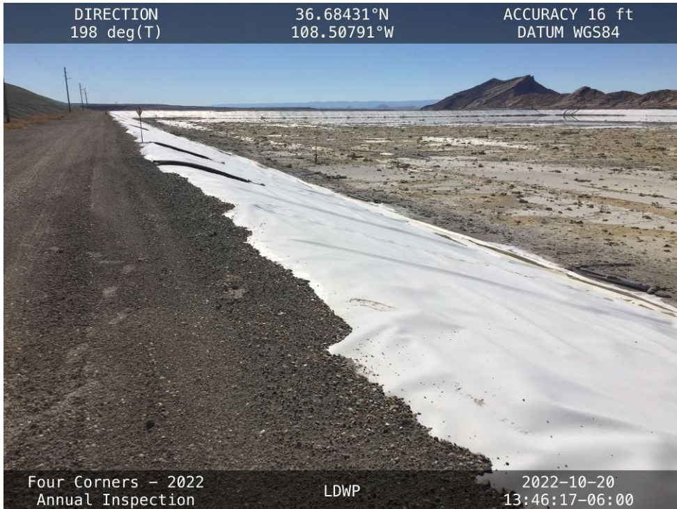
Portions of the outer pipes for the suction intake lines exposed across the East Embankment crest.
