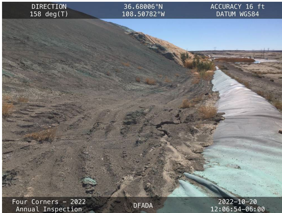
20221020 – IMG_4708 The downstream toe of the Cell 3 West Embankment, facing south.
