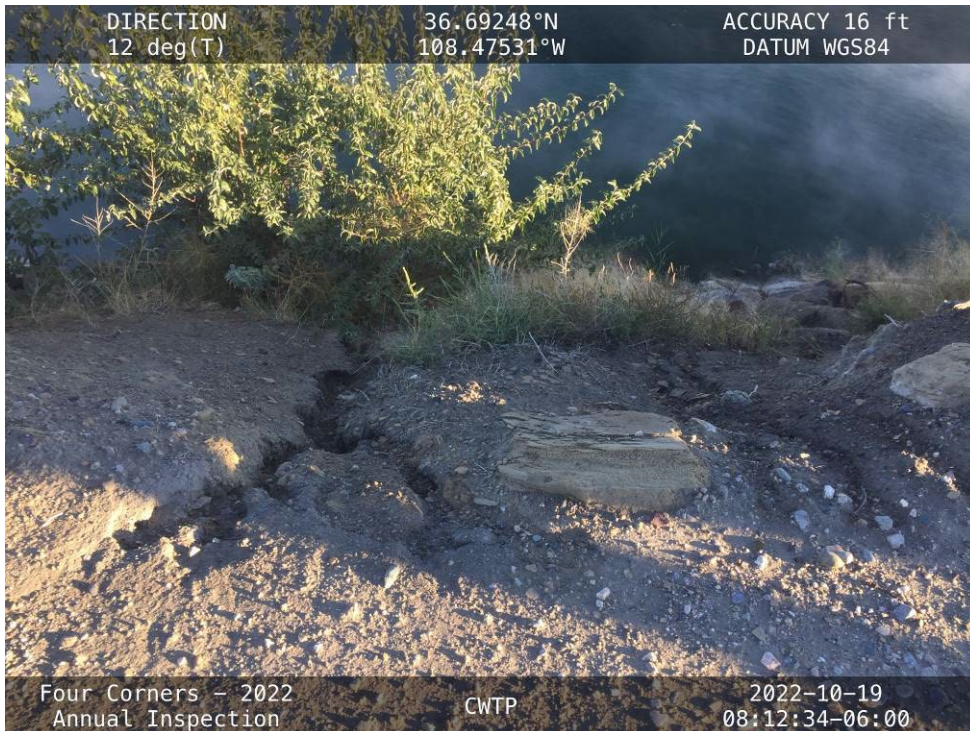
Loose soil and a 6-inch deep erosion hole on the downstream shoulder of the North Embankment.
