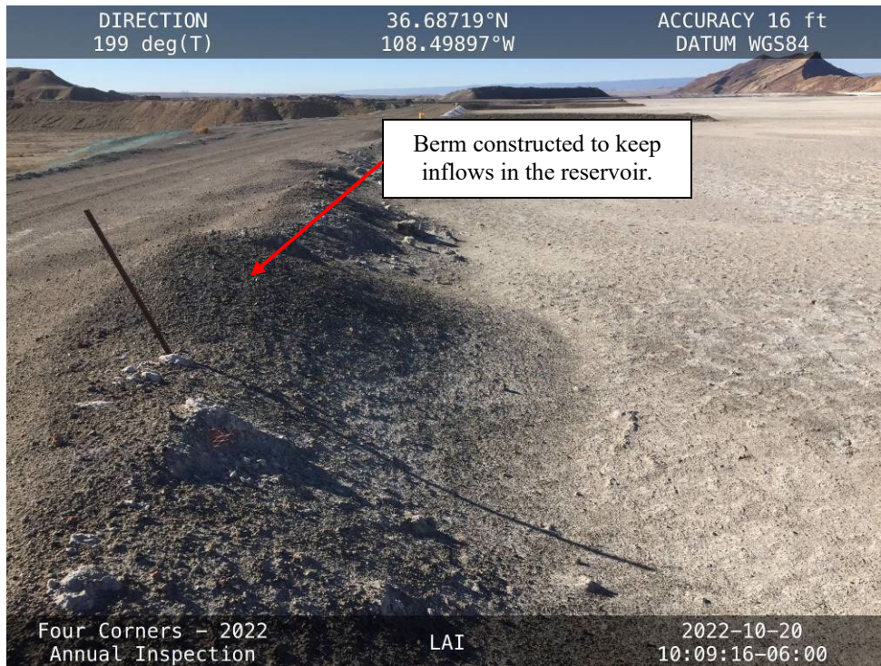
Bottom ash built up near the old V-ditch to contain the stormwater run-on.
