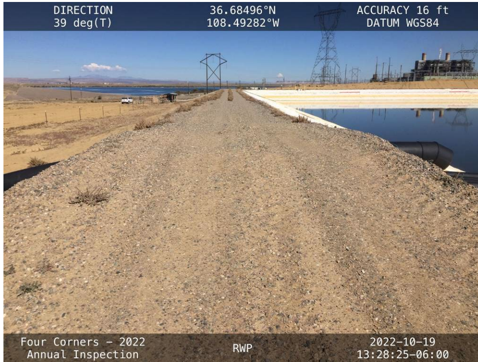
20221019 – IMG_4376 The crest of the RWP Cell Northwest Embankment, facing northeast.
