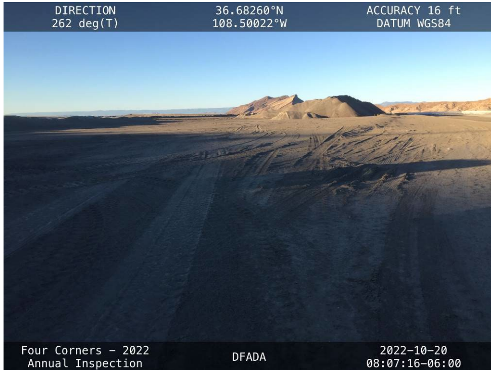
20221020 – IMG_4412 Cell 3, facing southwest from the South Embankment of the LAI.
