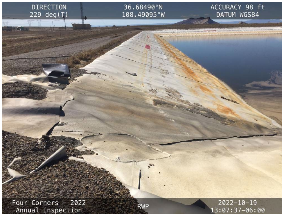
The liner pulling out of the anchor trench along the Northeast Embankment.
