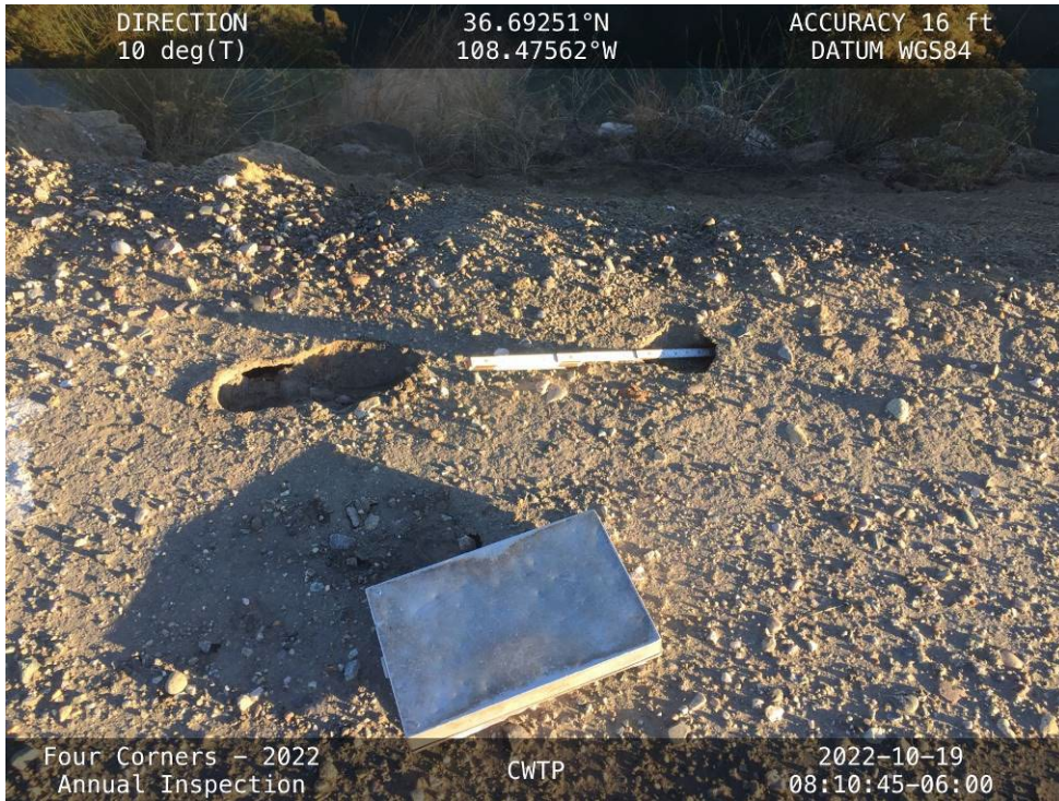
Loose soil and a 6-inch deep erosion hole on the downstream shoulder of the North Embankment.
