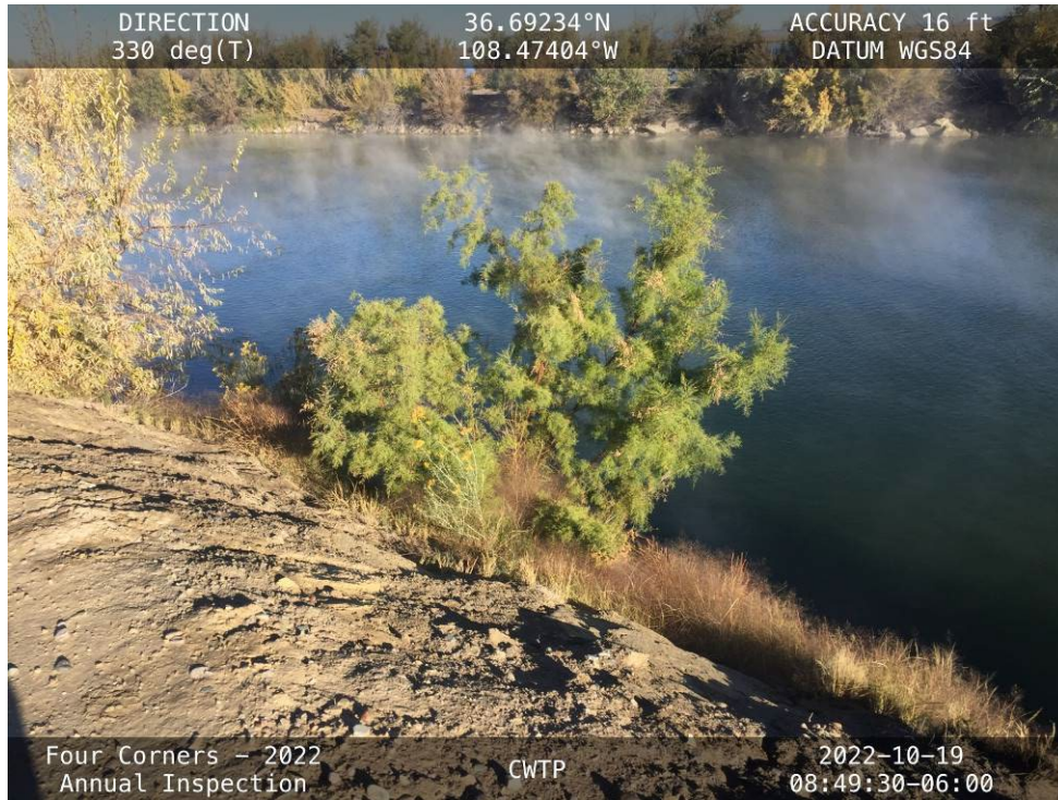
20221019 – IMG_4085 Vegetation to be removed from the downstream slope.
