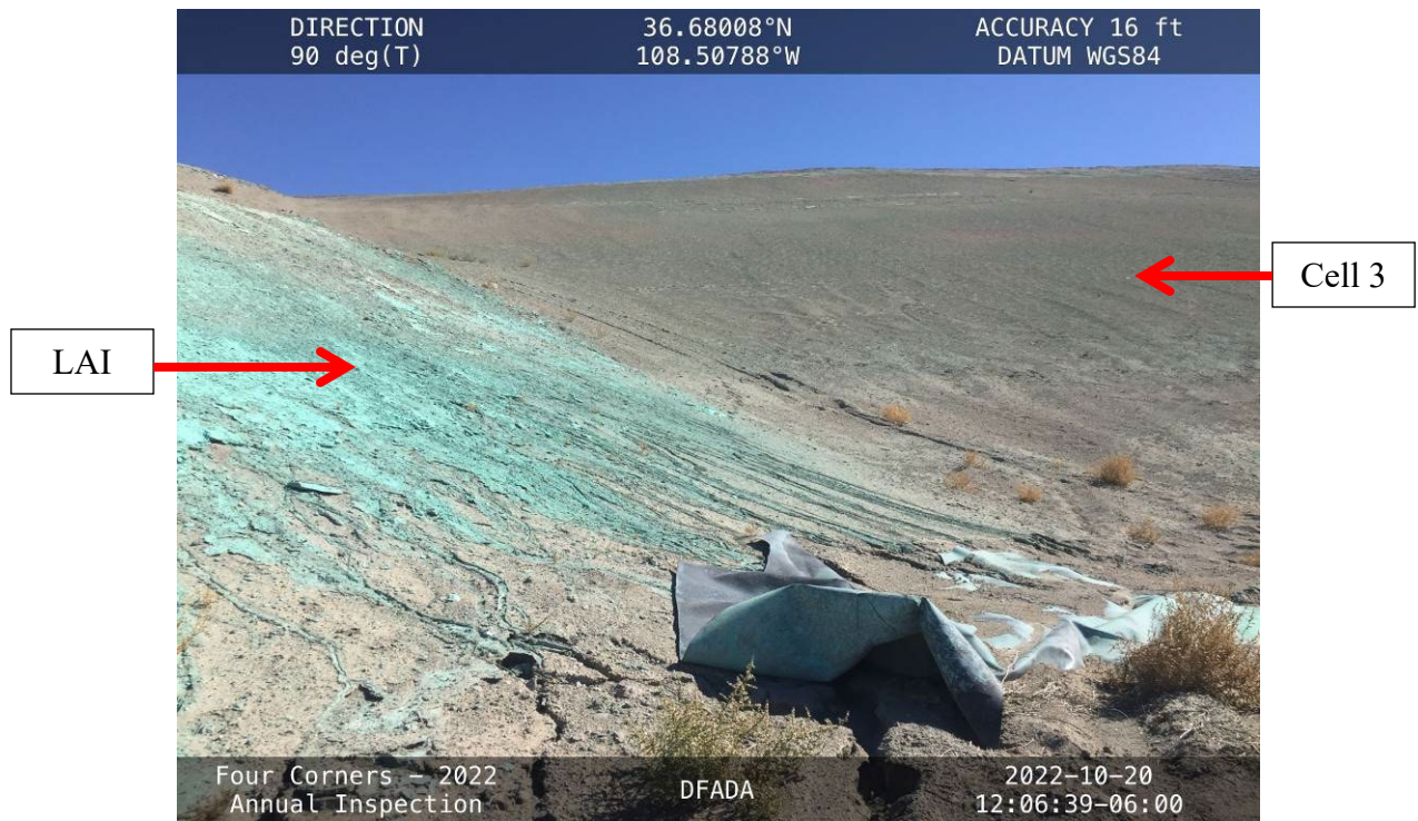
20221020 – IMG_4707 The junction of the LAI and Cell 3, facing east.
