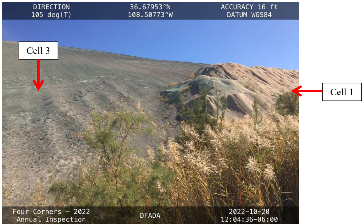
20221020 – IMG_4702 The Cell 3/Cell 1 junction, facing east from the toe.
