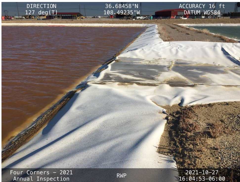
20211027-IMG_8106 The RWP cell reservoir below the elevation of the overflow weir in the Internal Embankment.
