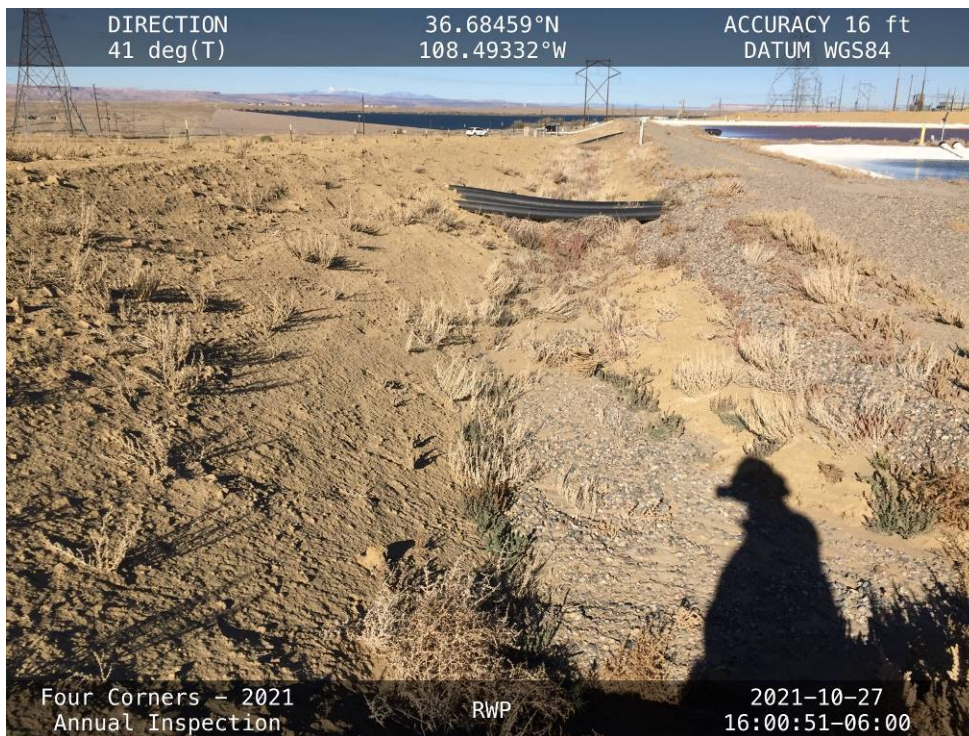
Tension cracks forming on the slope of the drainage ditch along the western corner of the pond.
