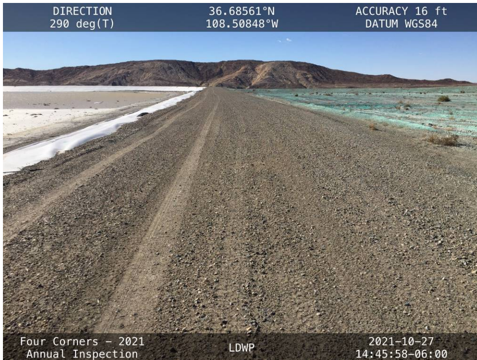
An area of previous liner repairs on the upstream slope of the North Embankment.
