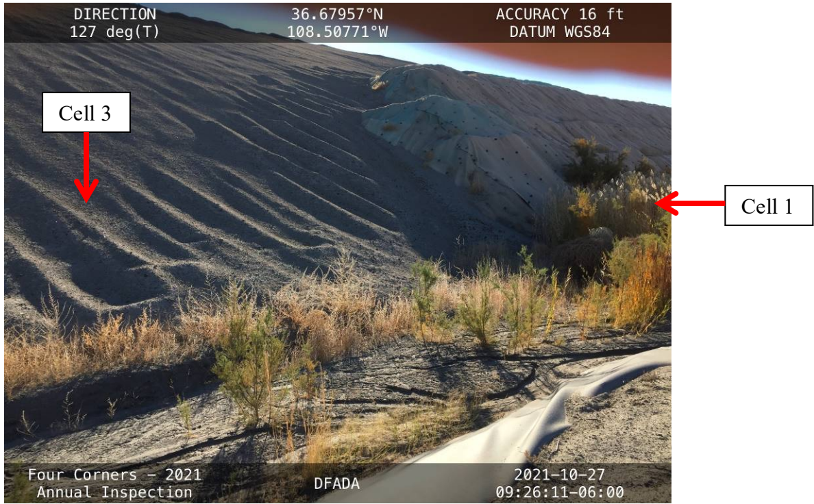
20211027-IMG_7596 The Cell 3/Cell 1 abutment, facing east from the toe.
