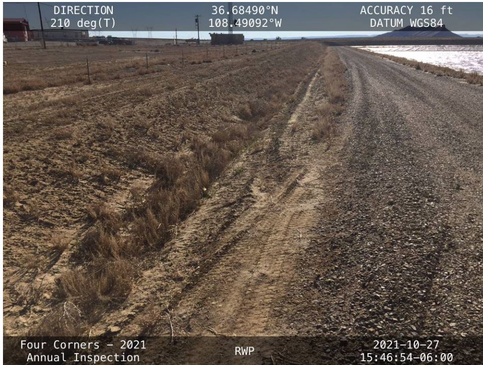
The drainage ditch along the downstream slope of the Southeast Embankment, facing southwest.
