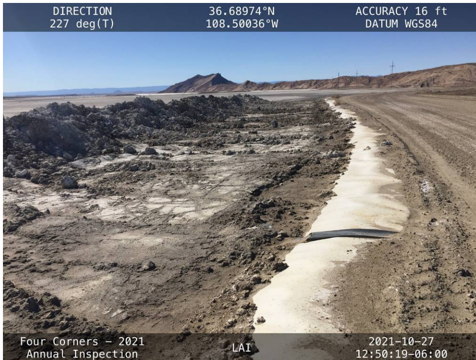
Ash and the CCR berm constructed to keep inflows off the crest at the north V-ditch, facing northeast.
