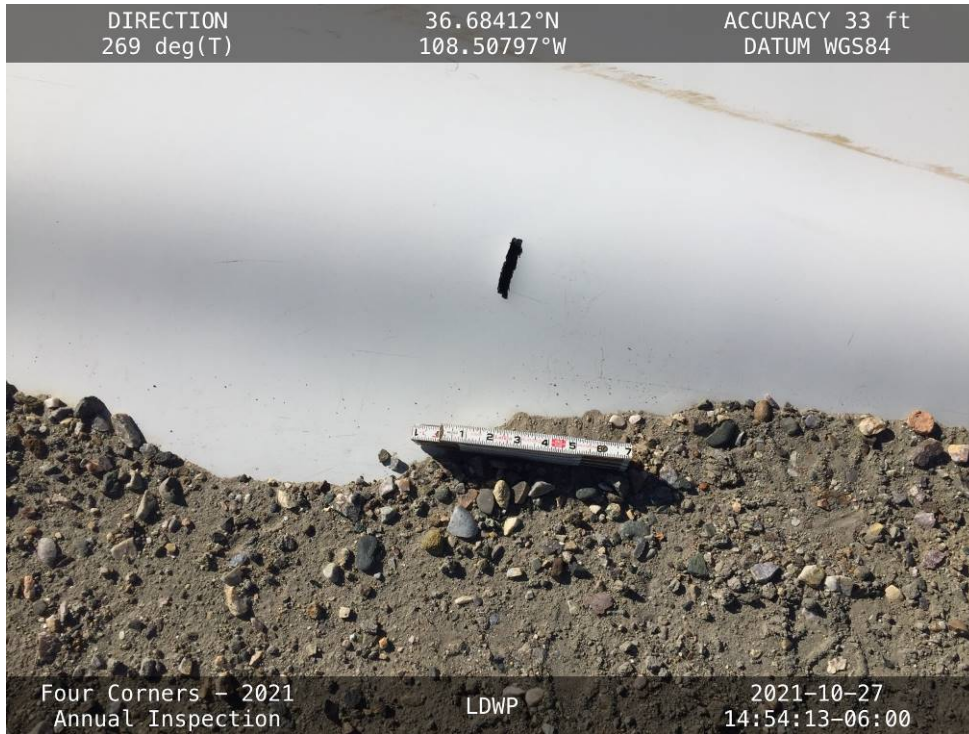
A 2-inch notch in the liner on the upstream shoulder of the East Embankment.
