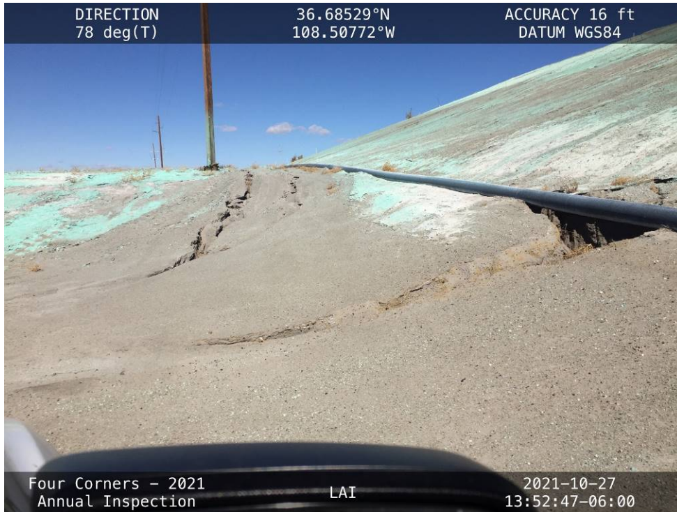
Erosion gullies at the toe of the West Embankment near the south end of the North Toe Butress.
