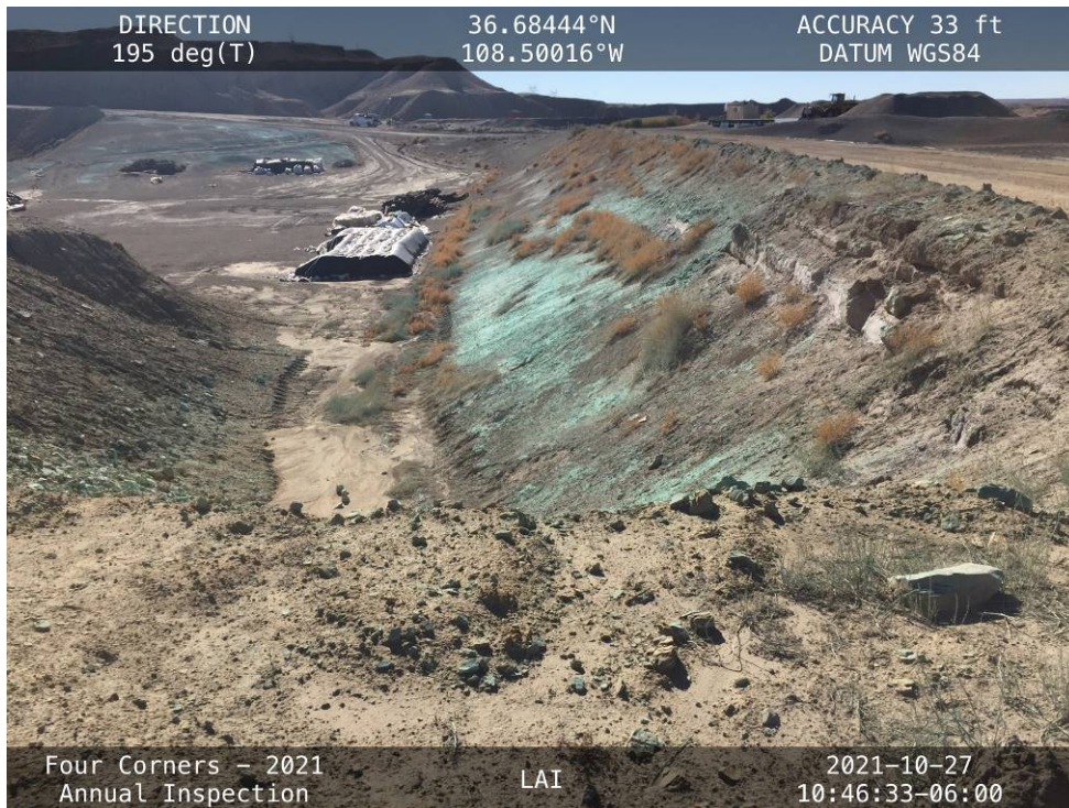
Holes at the edge of the anchor trench along the upstream side of the East Embankment.
