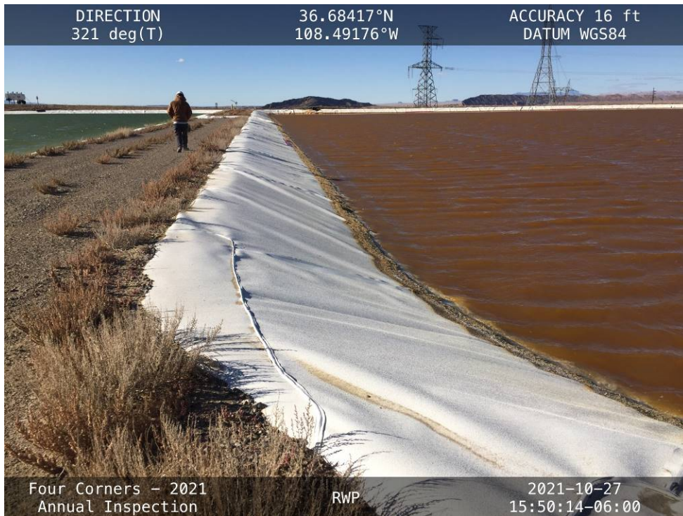
The drainage ditch along the downstream slope of the Southeast Embankment, facing southwest.
