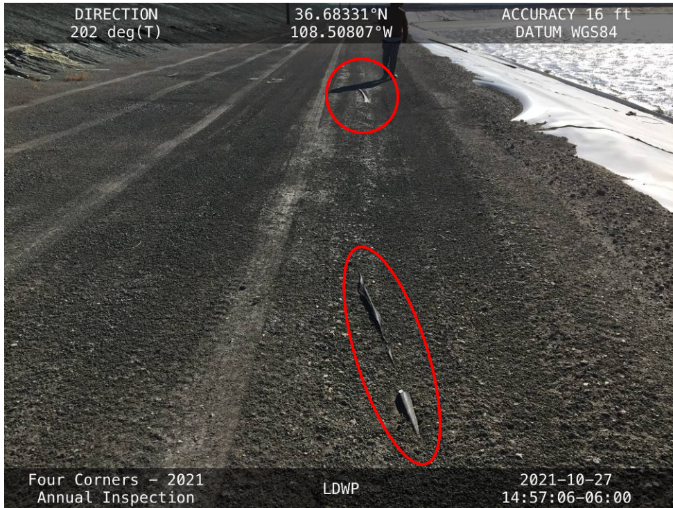
Portions of the liner exposed in the anchor trench along the East Embankment crest.
