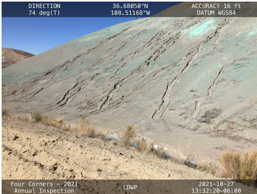
Erosion on the western half of the South Embankment downstream slope, facing north from the toe.
