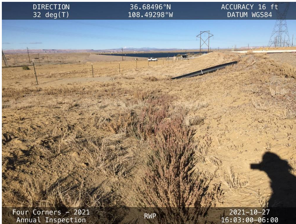
20211027-IMG_8095 The downstream slope of RWP Cell Northwest Embankment, facing northeast.
