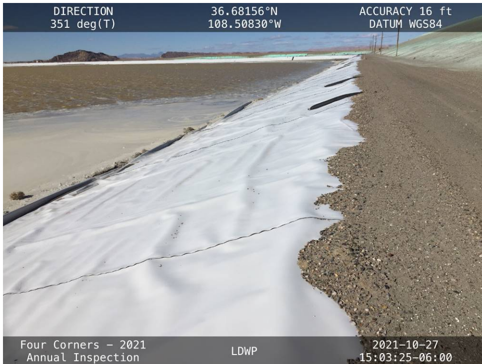
Portions of the liner exposed in the anchor trench along the East Embankment crest.
