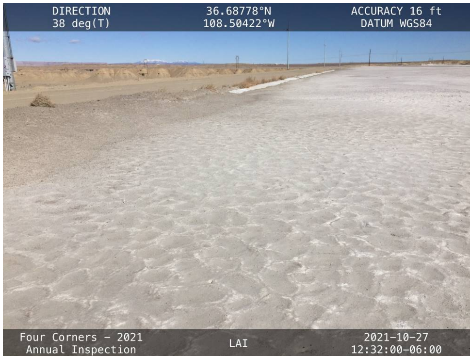
An erosion rill on the downstream slope of the Northwest Embankment.
