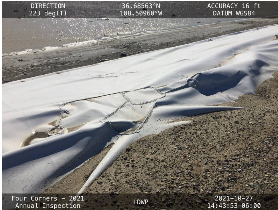
An area of previous liner repairs on the upstream slope of the North Embankment.
