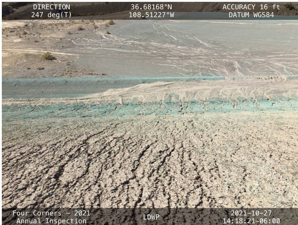
20211027-IMG_7945 The runout channels shown in IMG_8017 as seen from the crest of the West Embankment.
