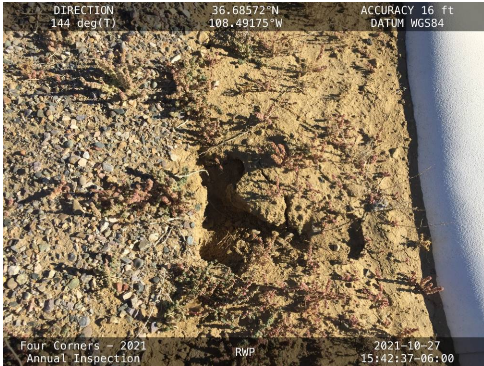
A shallow hole in the anchor trench on the Northeast Embankment.
