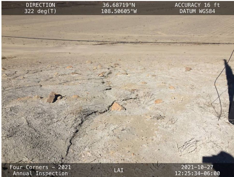
An erosion rill on the downstream slope of the Northwest Embankment.
