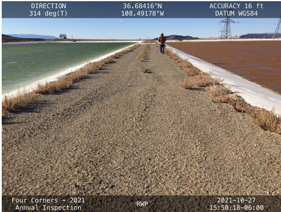
The crest of the FGD Pond cell Internal Embankment, facing northwest.
