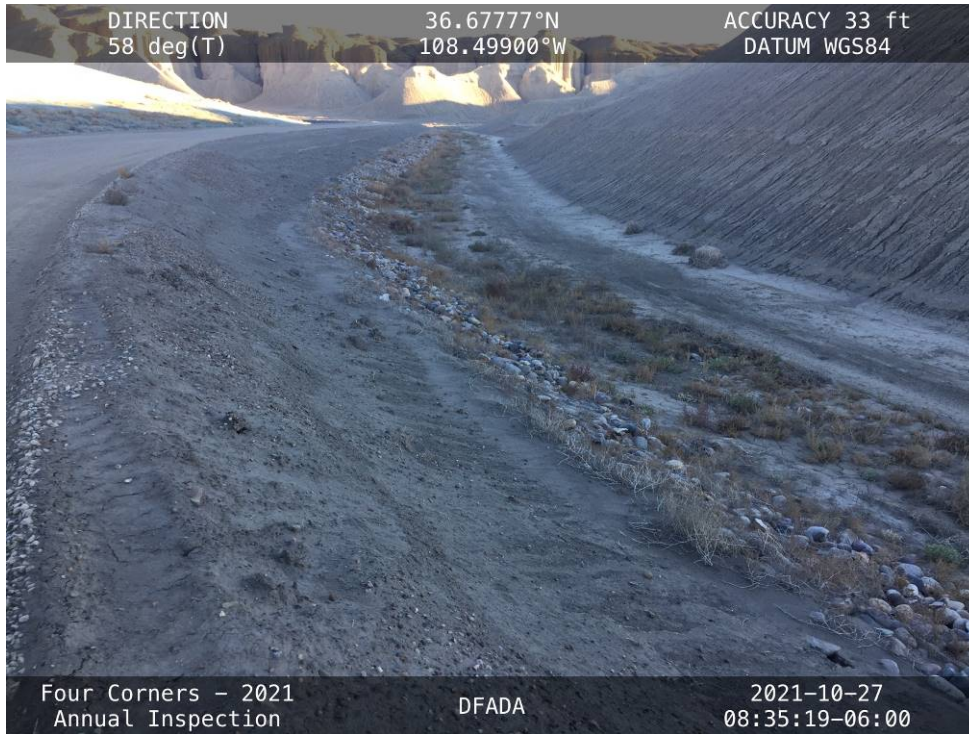
The Stormwater Diversion Channel along the southeast side of Cell 2.
