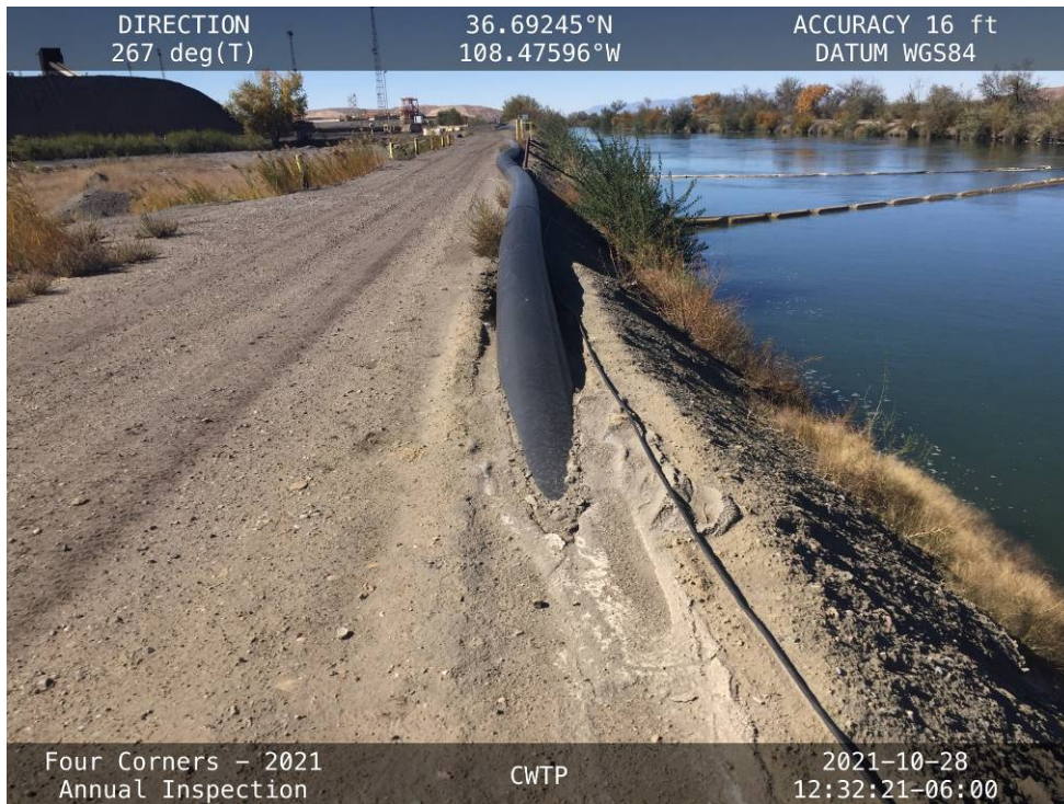
The 18-inch pipe that transfers water from the canal to the CWTP and the water level transducer.
