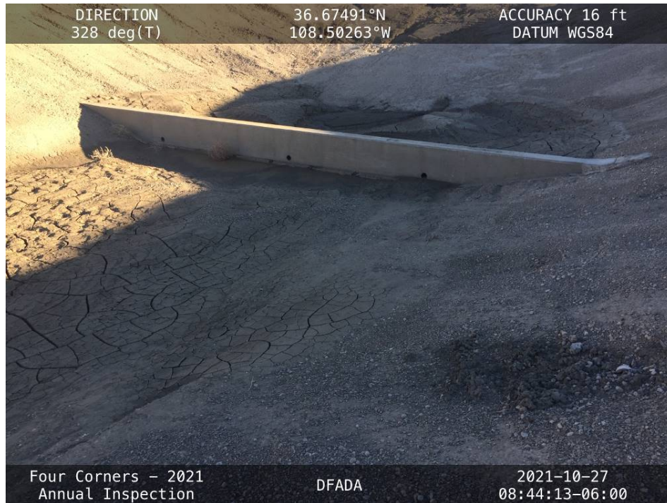
20211027 – IMG_7536 The new concrete weir wall in the new stilling basin.
