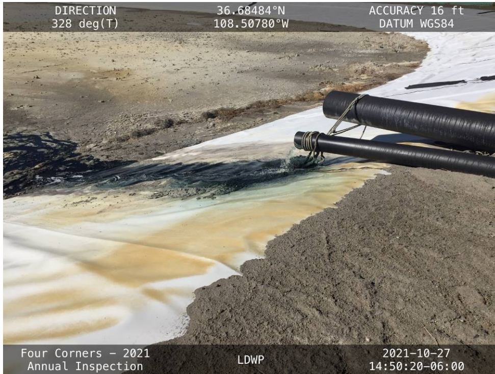
The 8-inch and 16-inch HDPE outlet pipes used to convey decant water from the LAI.
