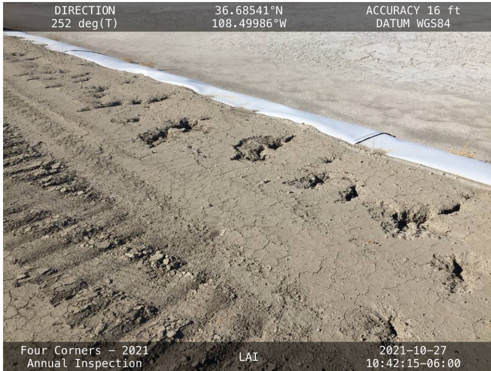
Holes at the edge of the anchor trench along the upstream side of the East Embankment.
