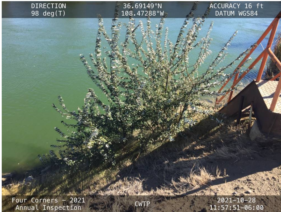
Vegetation near and erosion around the steps leading to the outfall headwall.
