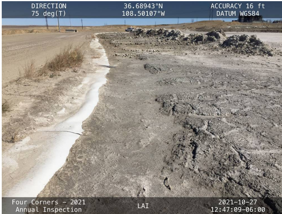
Ash and the CCR berm constructed to keep inflows off the crest at the north V-ditch, facing northeast.
