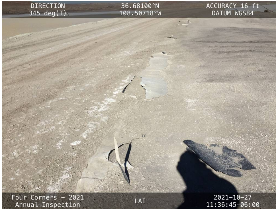
Tears in the exposed liner at the cenosphere mining area in the Southwest Corner.
