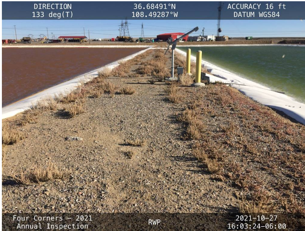
20211027-IMG_8099 The crest of the Internal Embankment, facing southeast.
