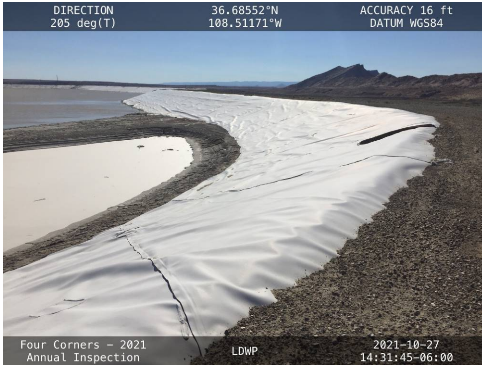
20211027-IMG_7966 The upstream slope of the West Embankment, facing south.
