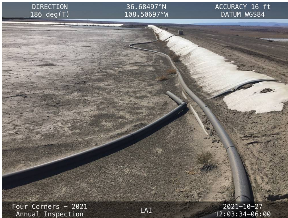
A liner mud crack on the upstream side of the West Embankment crest.
