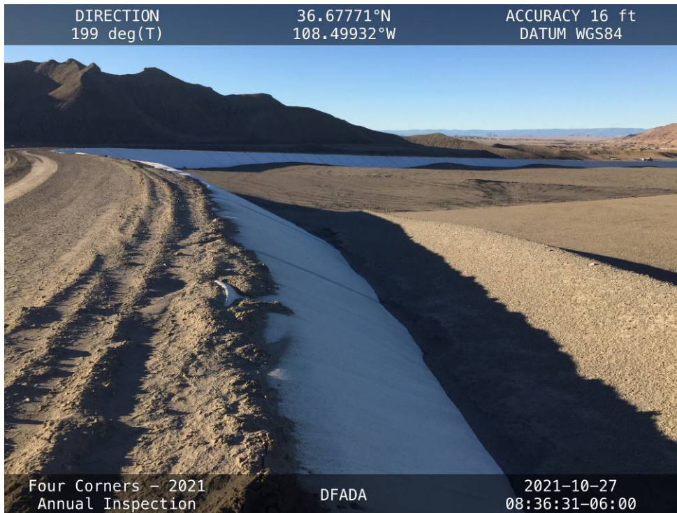
The Stormwater Diversion Channel along the southeast side of Cell 2.
