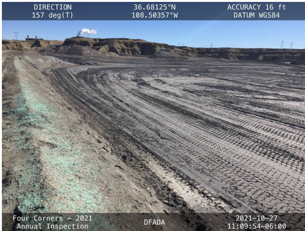
20211027-IMG_7691 The top of the eastern portion of Cell 1, facing east from the LAI crest.
