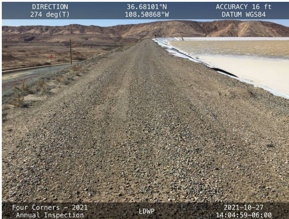
The upstream slope of the East Embankment, facing north from the southeast corner.
