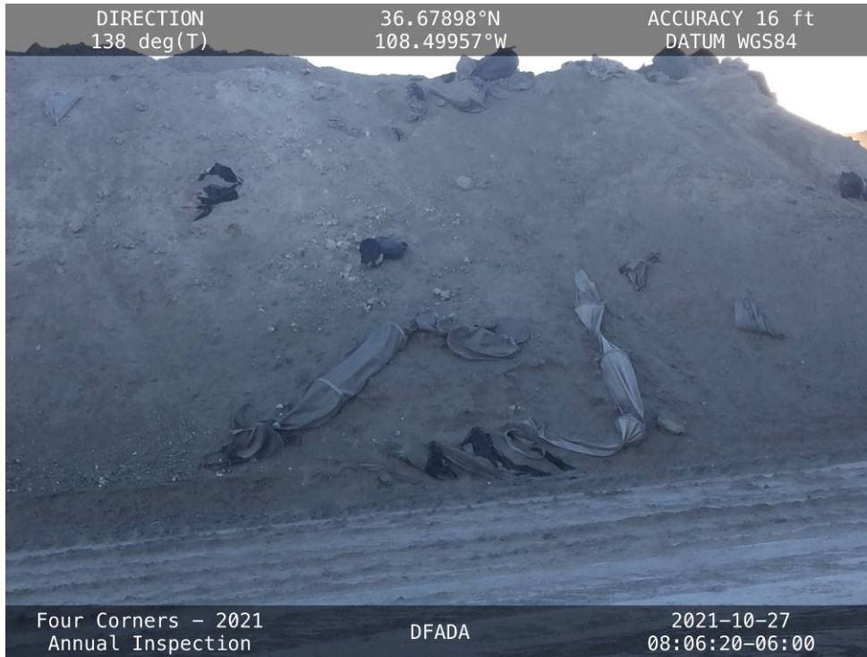
20211027-IMG_7497 Filter bags and other debris disposed of in Cell 2.
