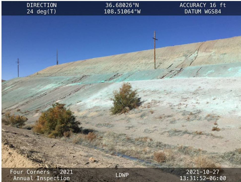
Erosion on the western half of the South Embankment downstream slope, facing north from the toe.
