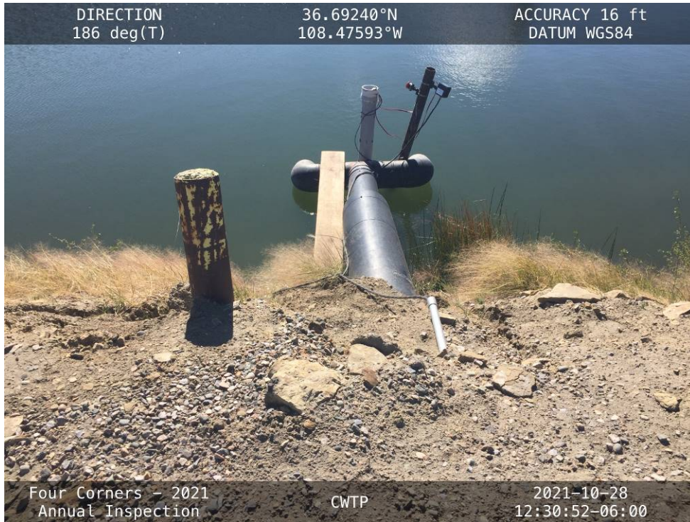
The 18-inch pipe that transfers water from the canal to the CWTP and the water level transducer.
