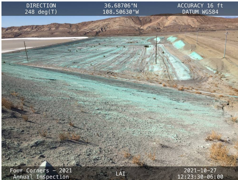
Erosion along the upper portion of the West Embankment, facing downstream from the crest.
