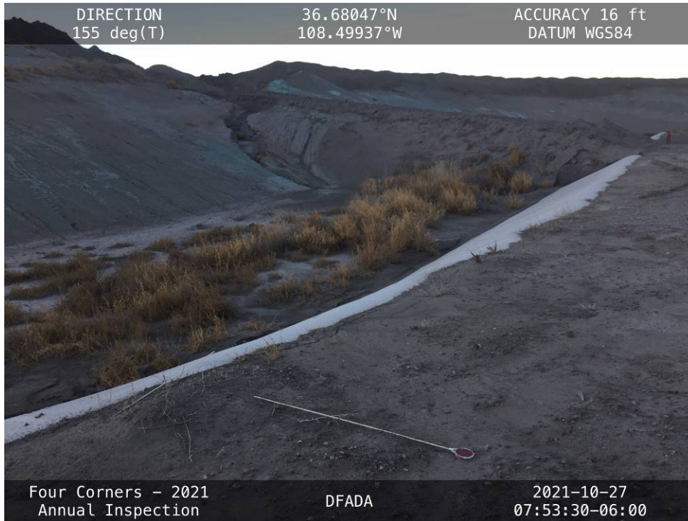
An erosion gully in the groin of the access ramp to Cell 2, facing south from the north side.
