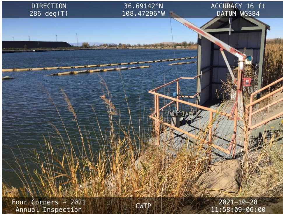
The CWTP flow monitoring structure on the eastern portion of the embankment.
