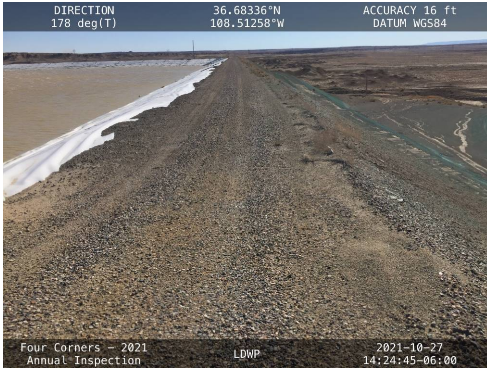
20211027-IMG_7949 The crest of the West Embankment, facing south.
