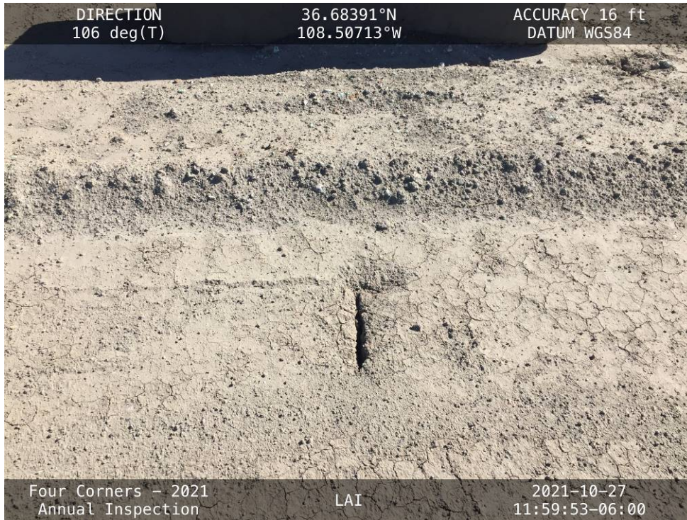
A liner mud crack on the upstream side of the West Embankment crest.
