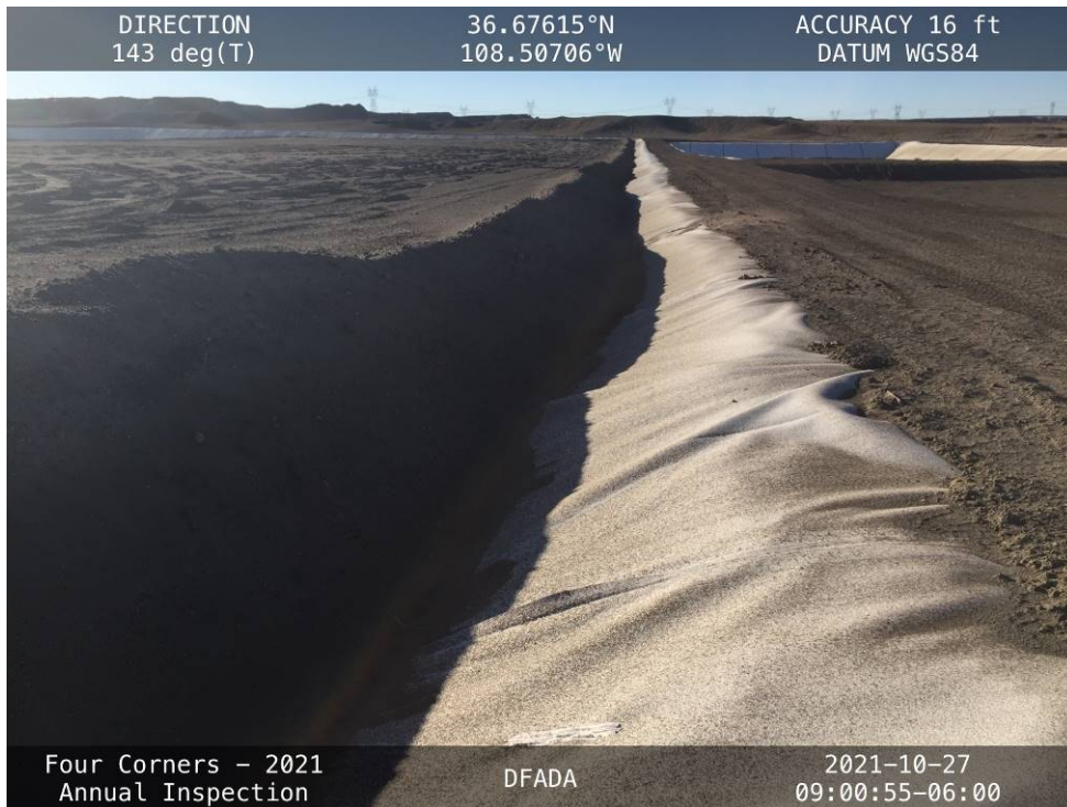
The new Cell 4 leachate collection pond, facing south from the north side.
