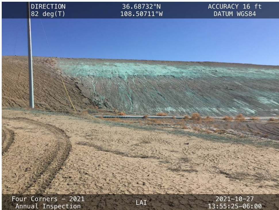
Erosion gullies at the toe of the West Embankment near the south end of the North Toe Butress.
