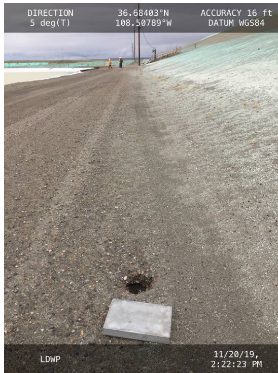
A settlement monument pin on the East Embankment crest.
