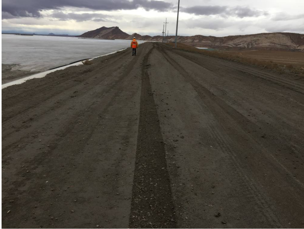
20191120 – IMG_6623 The crest of the Northwest Embankment, facing southwest.
