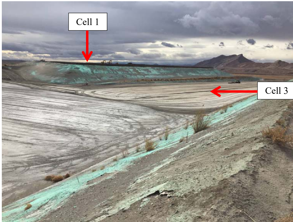
20191120 – IMG_6521 DFADA Cell 1 and the western portion of Cell 3, facing southwest.
