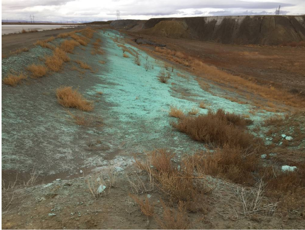
20191120 – IMG_6549 The downstream slope of the East Embankment.
