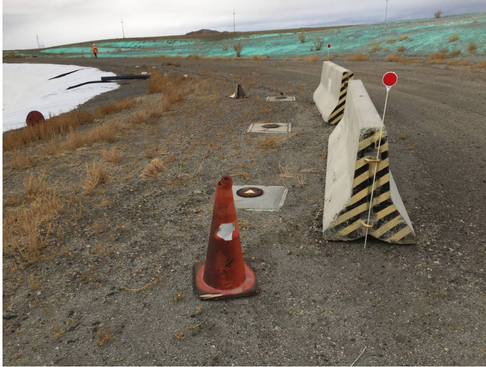
20191120 – IMG_6748 The surface monuments for piezometers P-23, P-24, and P-25.
