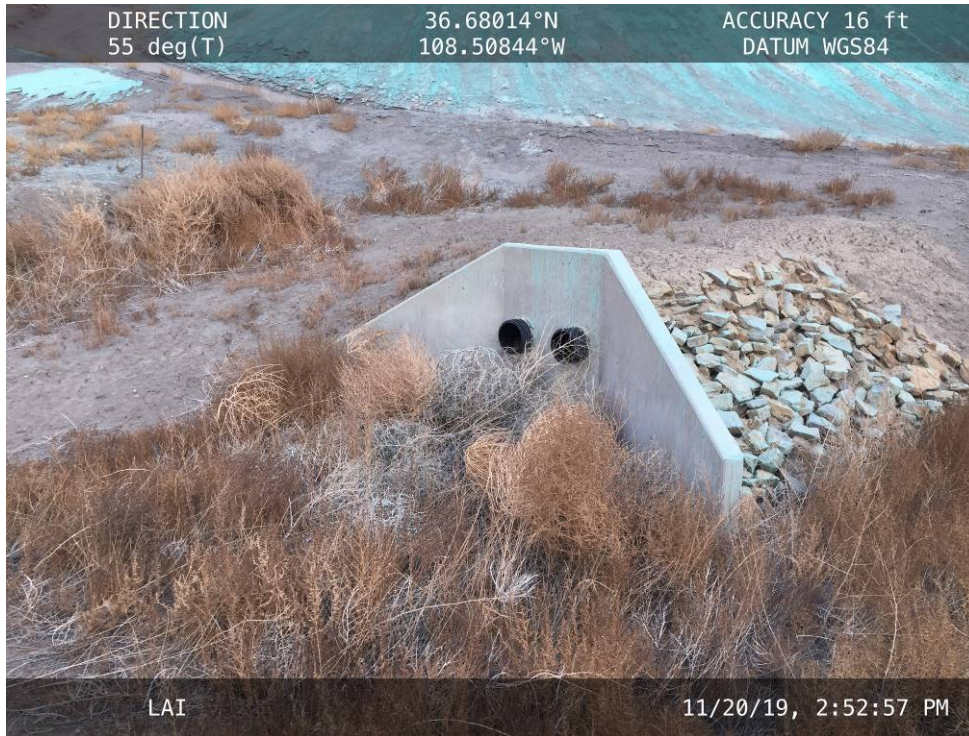
20191120 – IMG_6795 The South Embankment toe drain in a dry condition.
