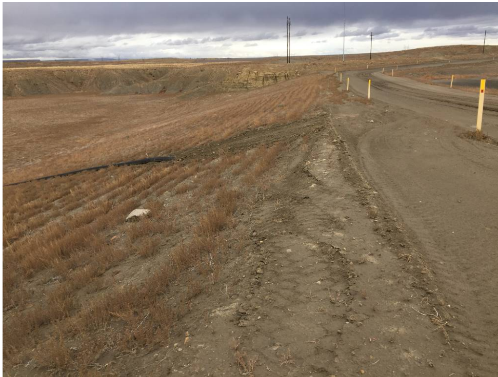
20191120 – IMG_6605 The downstream slope of the Northwest Embankment, facing east.
