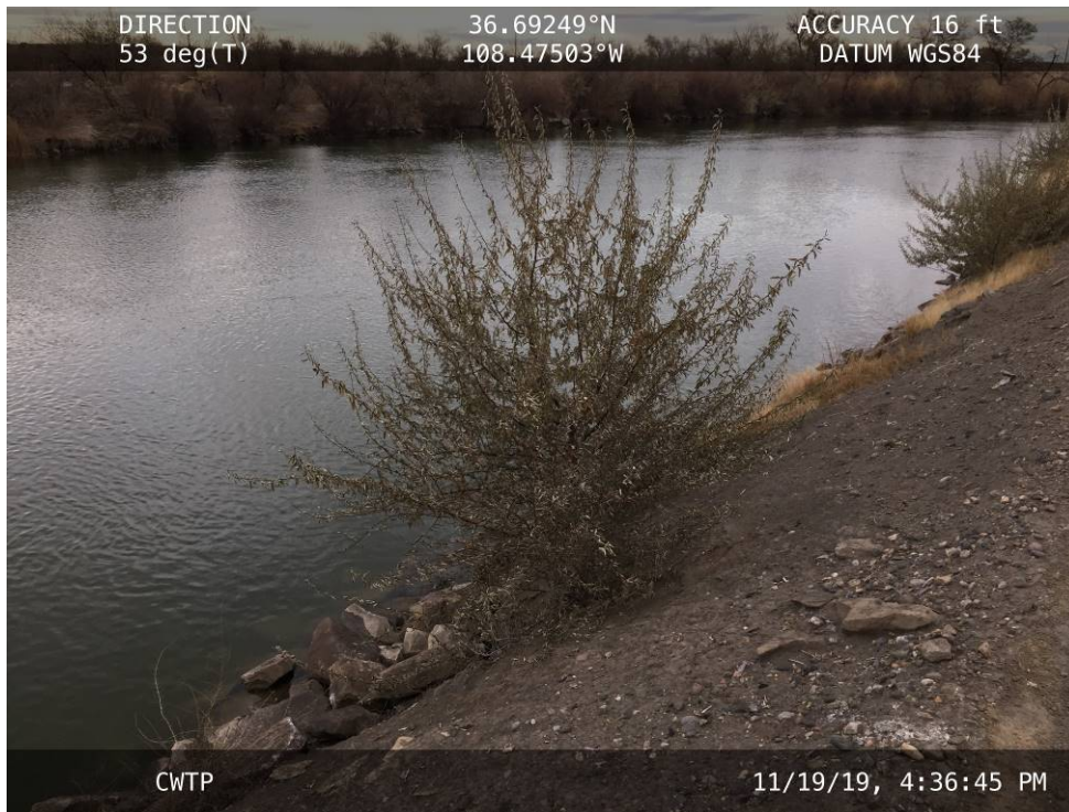
Erosion on the upstream slope along the northern portion of the embankment.
