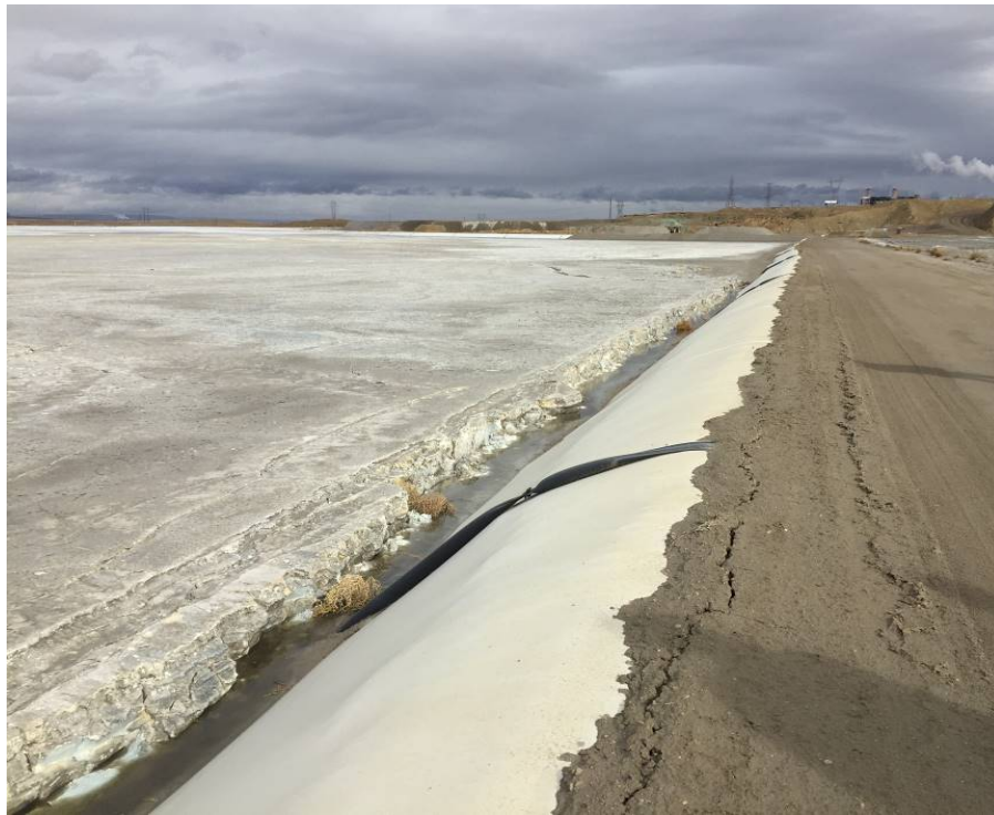
20191120 – IMG_6517 The upstream slope of the South Embankment, facing east.
