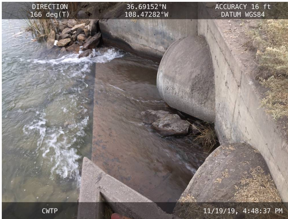
20191119 – IMG_6288 The outfall from the CWTP to the discharge canal.
