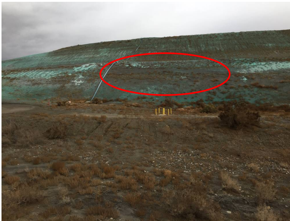
20191120 – IMG_6772 Repair of surface slough observed during the 2018 inspection (2018 IMG_1435).
