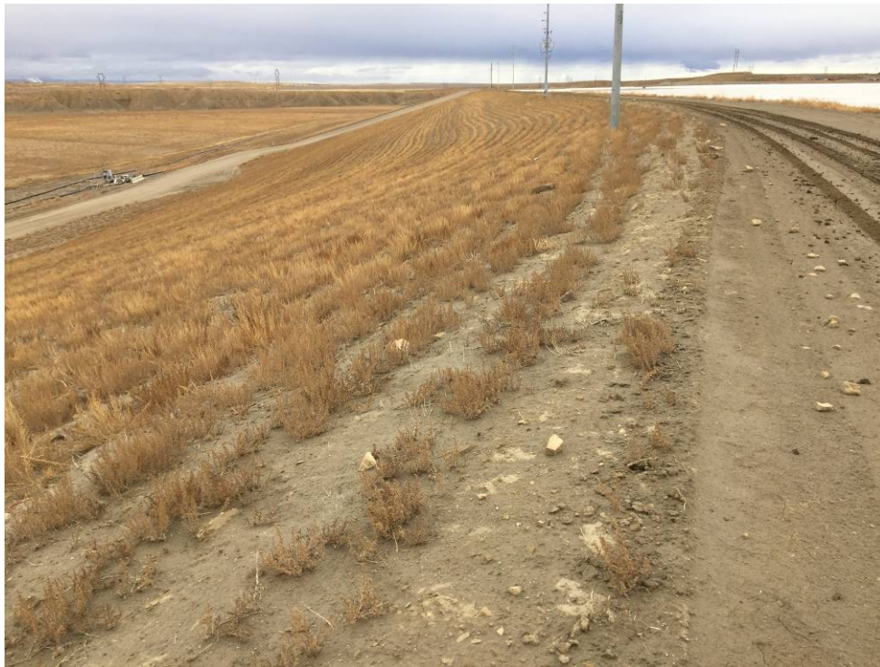
20191120 – IMG_6631 The downstream slope of the Northwest Embankment, facing northeast.
