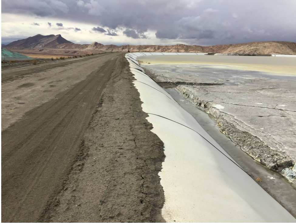
20191120 – IMG_6513 The upstream slope of the South Embankment, facing west.
