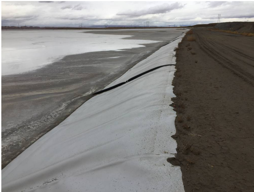
20191120 – IMG_6552 The upstream slope of the East Embankment, facing north.
