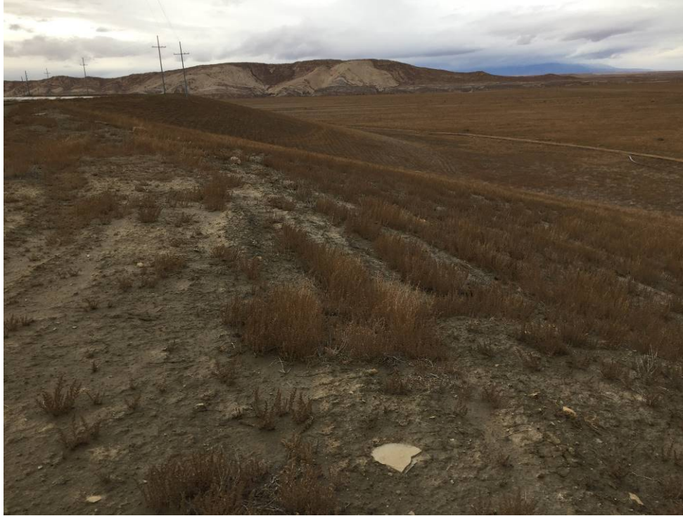
20191120 – IMG_6600 The downstream slope of the Northwest Embankment, facing west.
