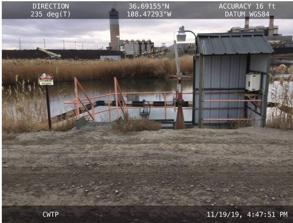
20191119 – IMG_6287 The CWTP flow monitoring structure on the eastern portion of the embankment.
