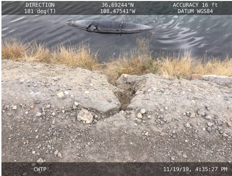
Erosion on the upstream slope along the northern portion of the embankment.
