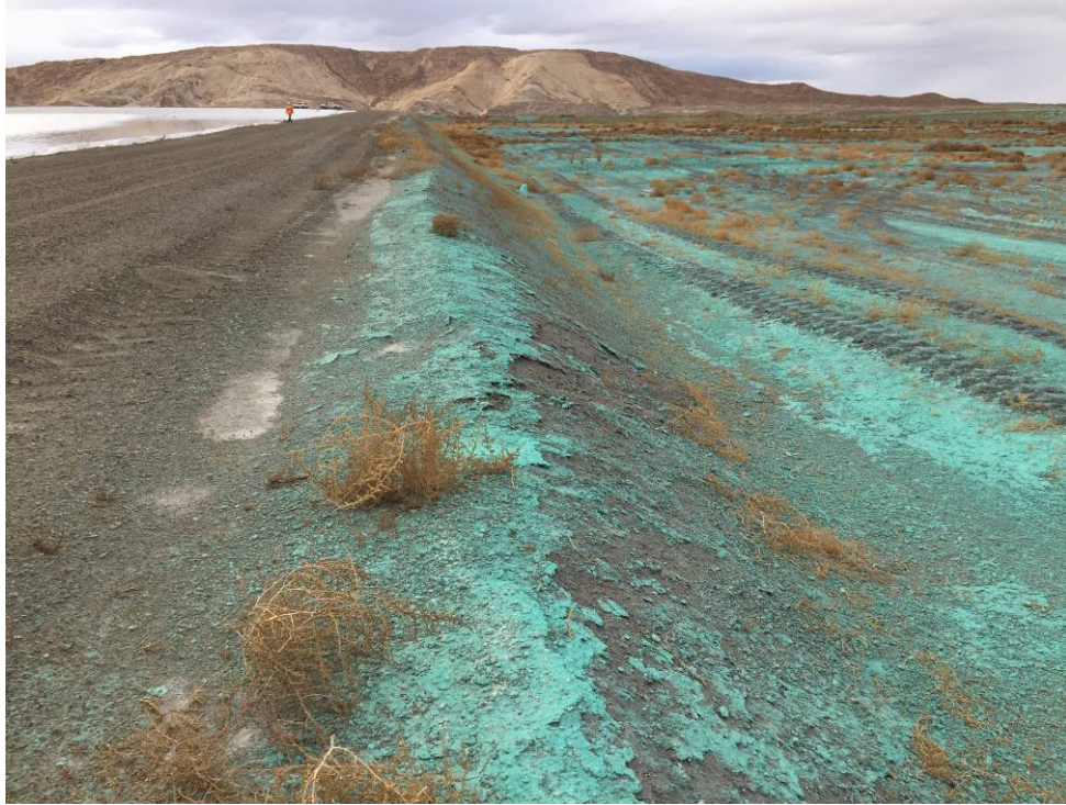
20191120 – IMG_6762 The downstream slope of the North Embankment, facing west.
