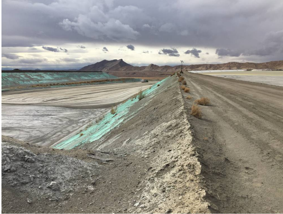
20191120 – IMG_6527 The downstream slope of the South Embankment, facing west.
