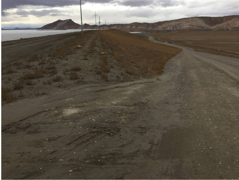
20191120 – IMG_6620 The downstream slope of the Northwest Embankment, facing west.
