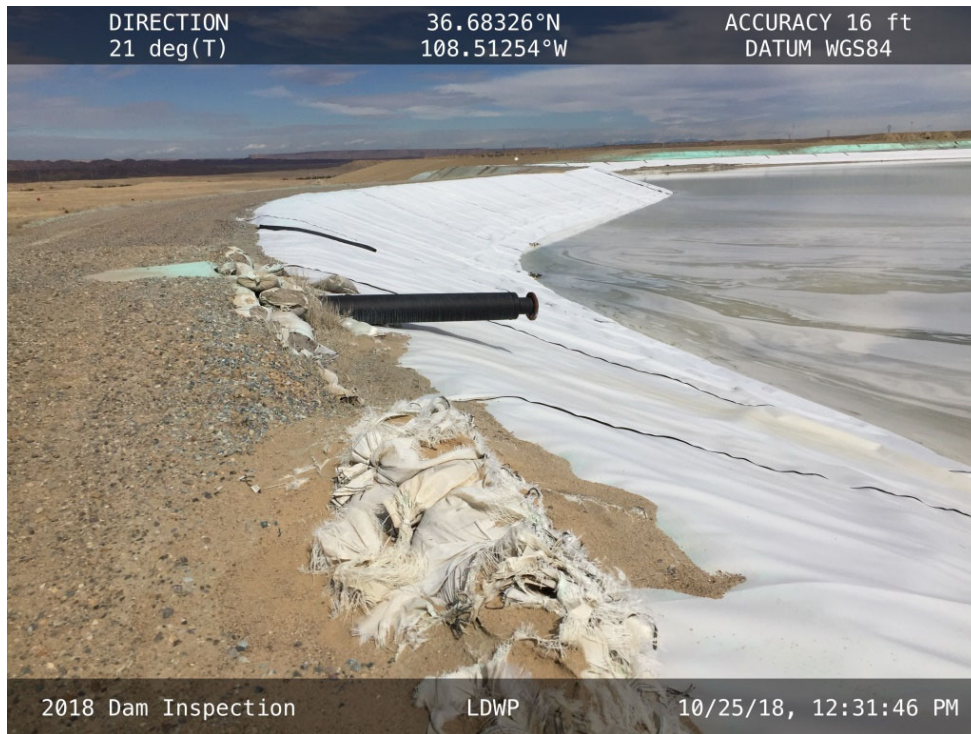
The discharge pipe from the Pond 3 Pump House along the West Embankment.
