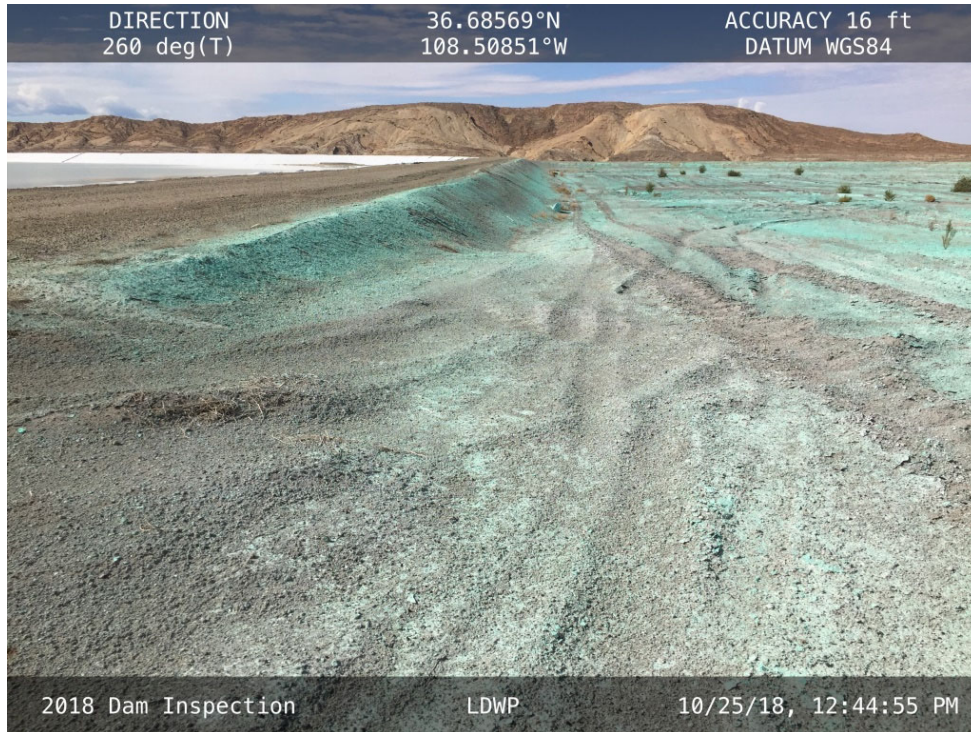
20181025 – IMG_1539 The downstream slope of the North Embankment, facing west.
