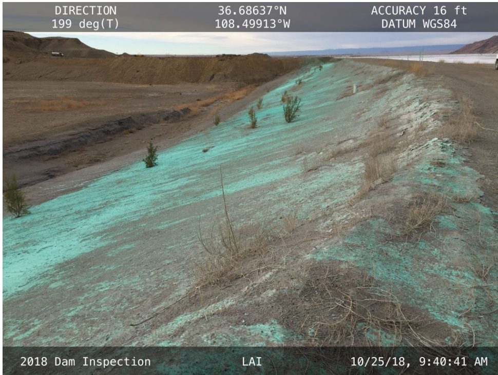
20181025 – IMG_1383 The downstream slope of the East Embankment, facing south.
