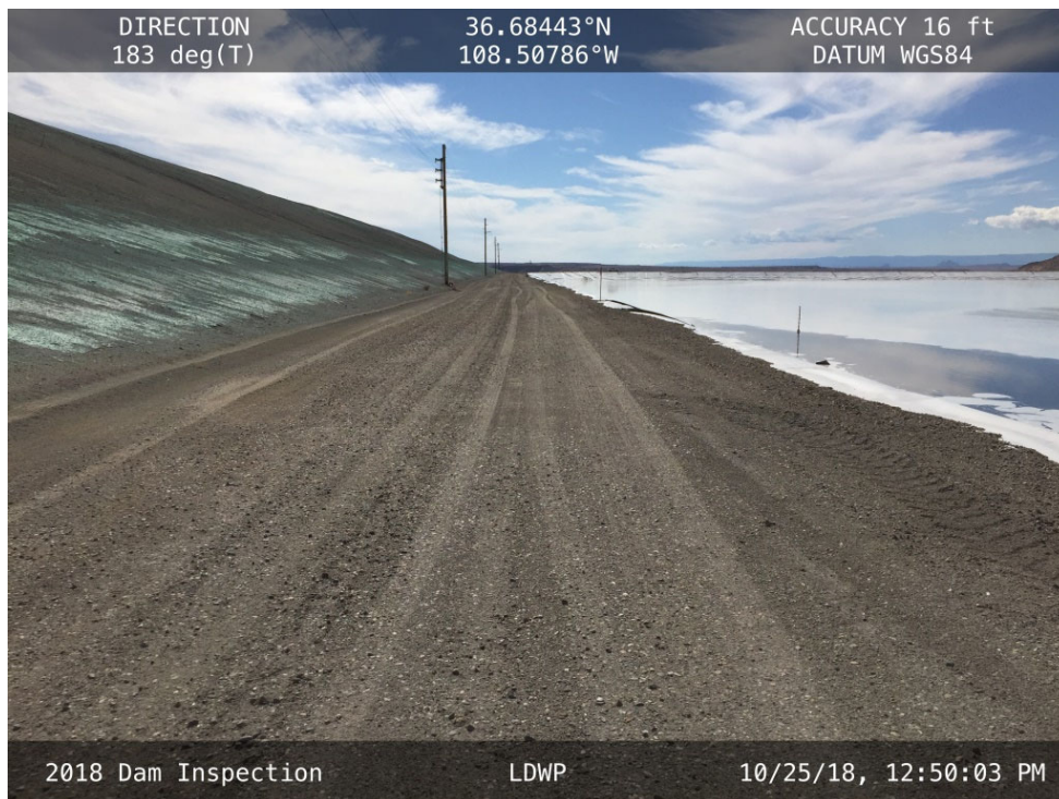
20181025 – IMG_1566 The crest of the East Embankment, facing south.
