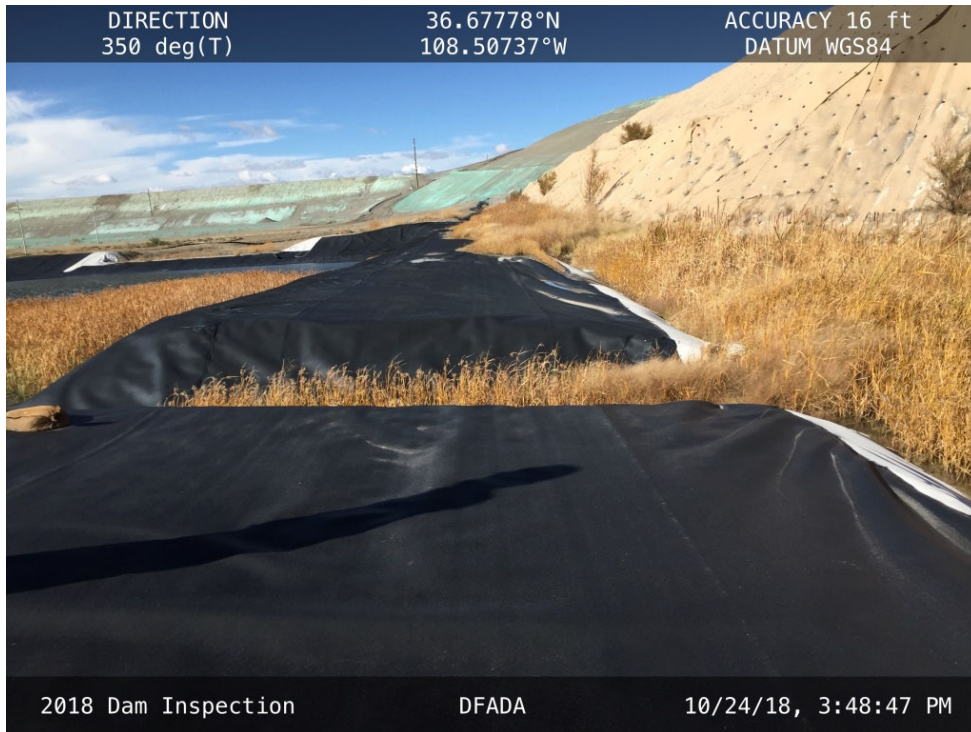
Vegetation growing in the drainage ditch and overflow channel of the leachate collection pond.
