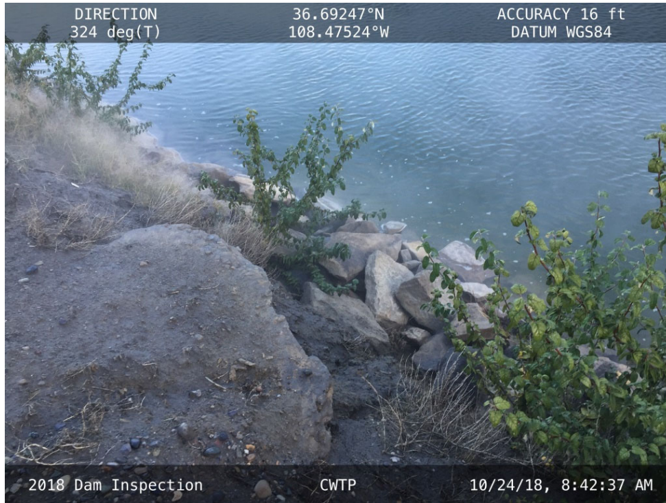
20181024 – IMG_0915 Vegetation and riprap along the waterline of the downstream slope.
