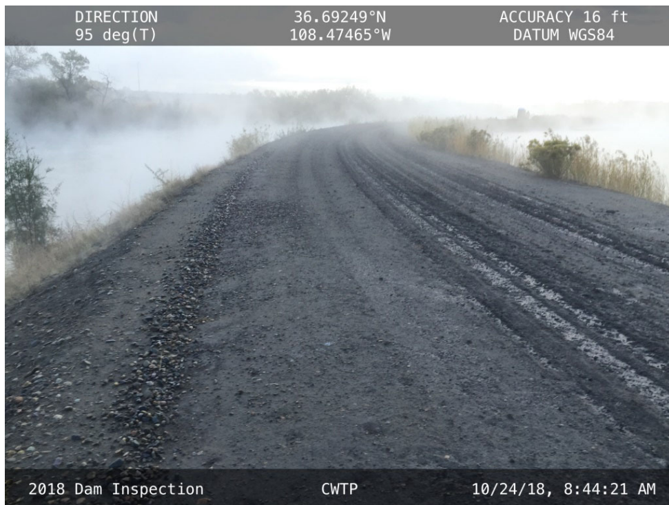
20181024 – IMG_0920 The crest of the CWTP embankment, facing east.
