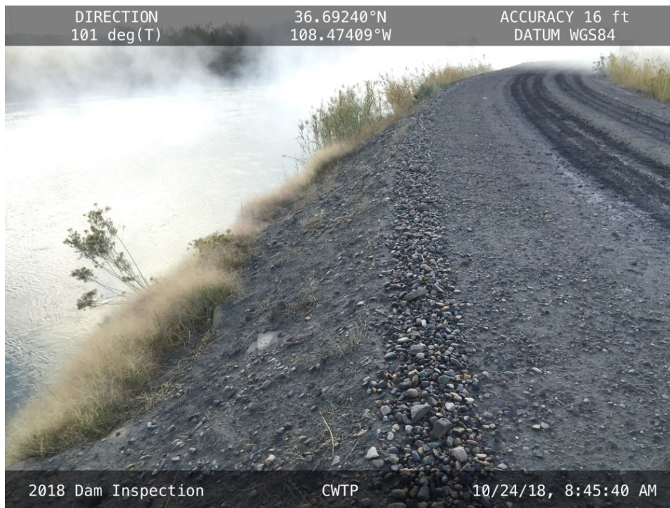
20181024 – IMG_0923 The downstream slope of the CWTP embankment, facing east.
