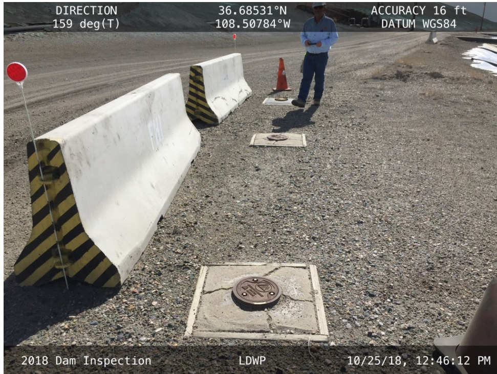
20181025 – IMG_1543 The surface monuments for piezometers P-23, P-24, and P-25.
