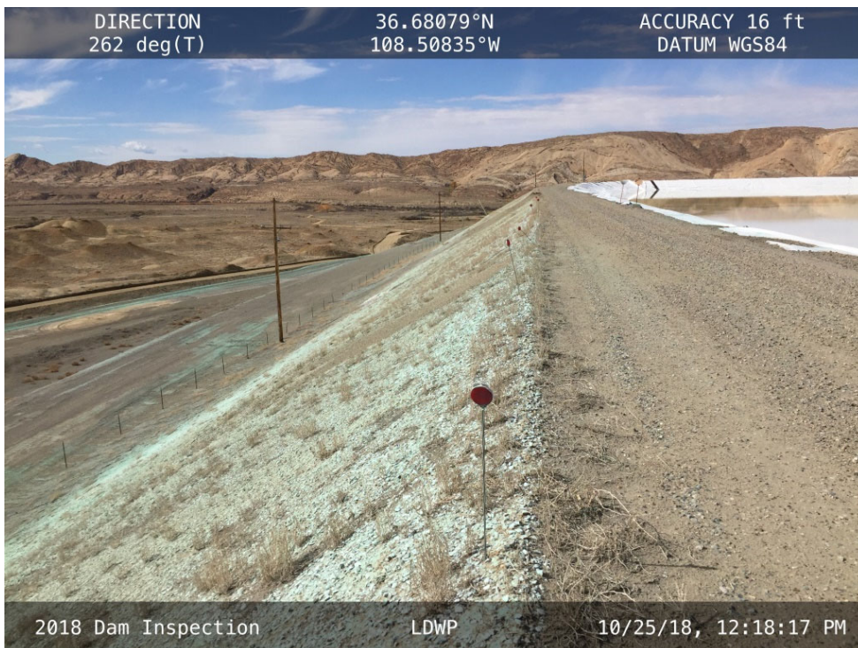
20181025 – IMG_1448 The downstream slope of the South Embankment, facing west.
