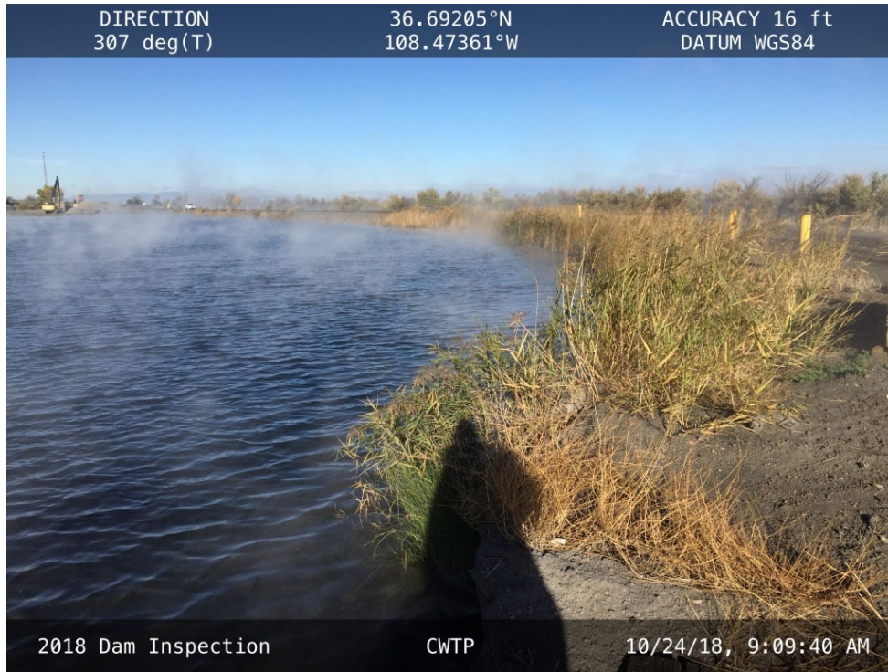
20181024 – IMG_0954 The upstream slope of the CWTP, facing west.
