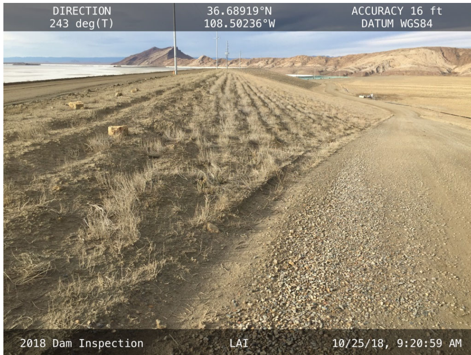
20181025 – IMG_1335 The downstream slope of the Northwest Embankment, facing west.
