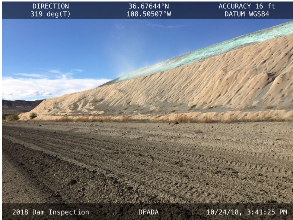
20181024 – IMG_1135 The south slope of DFADA Cell 1, facing west along the toe.
