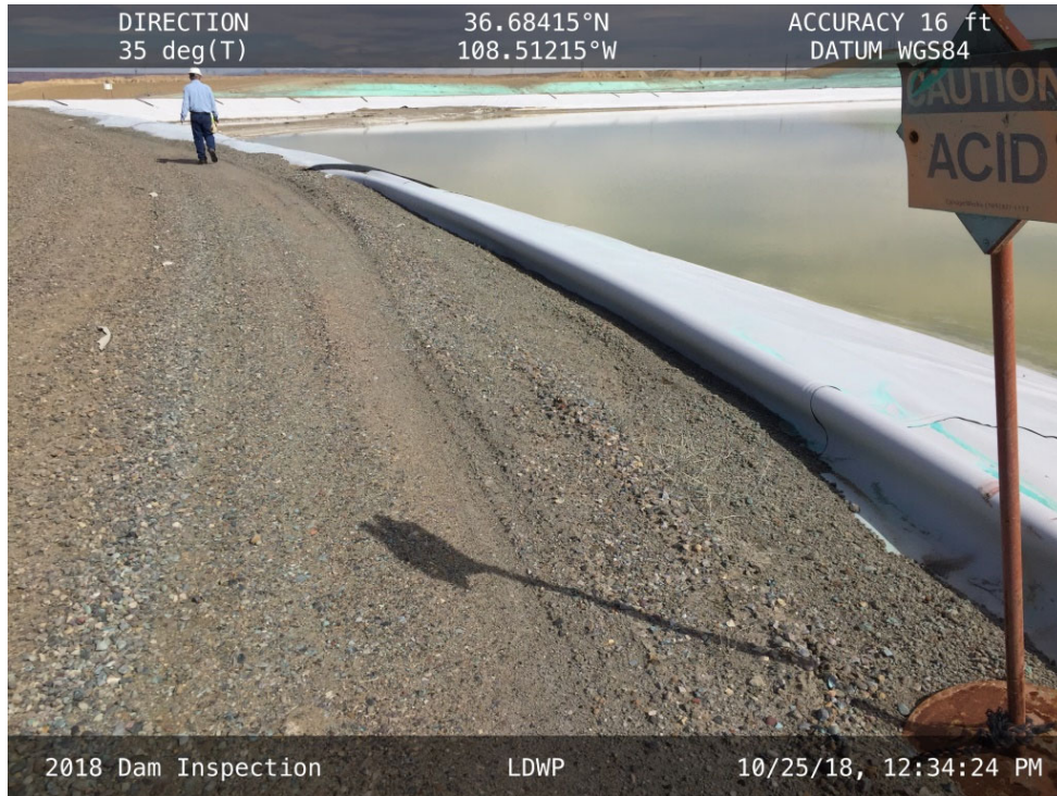
The liner pulling out of the anchor trench in the northern portion of the West Embankment.
