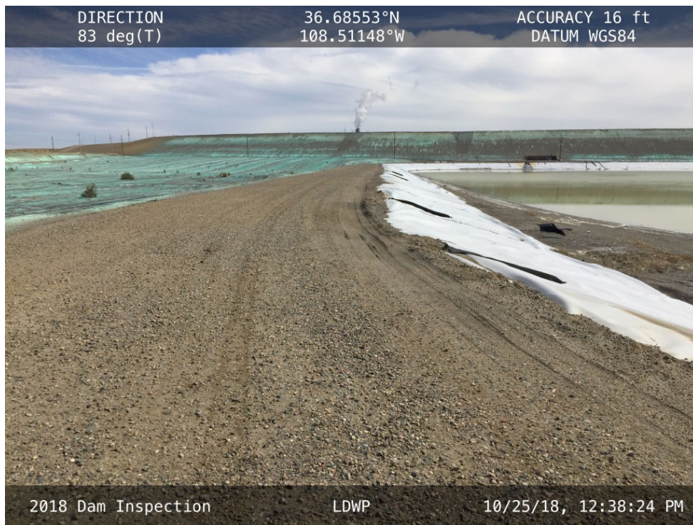
20181025 – IMG_1526 The crest of the North Embankment, facing east.
