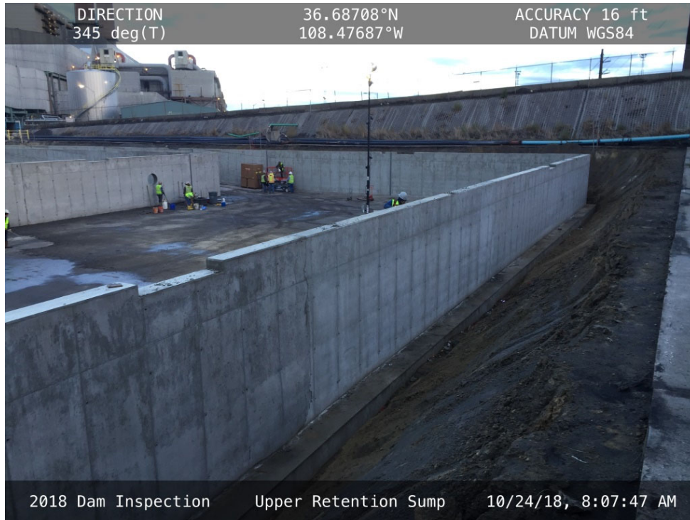
20181024 – IMG_0882 Construction of the Upper Retention Sump Tank, facing northwest.
