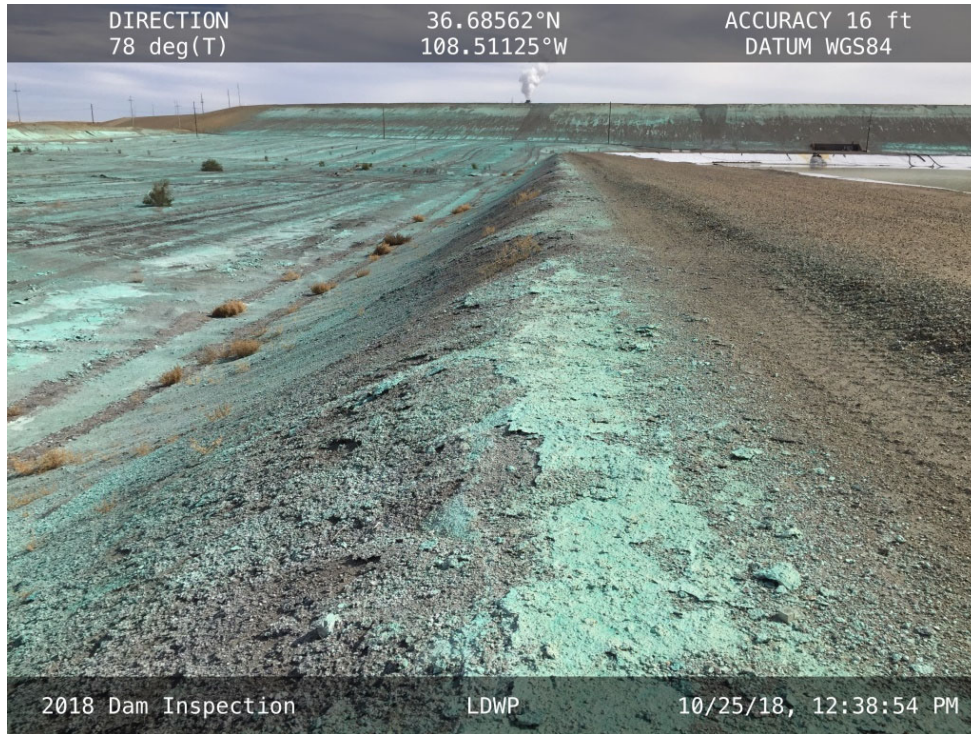
20181025 – IMG_1528 The downstream slope of the North Embankment, facing east.
