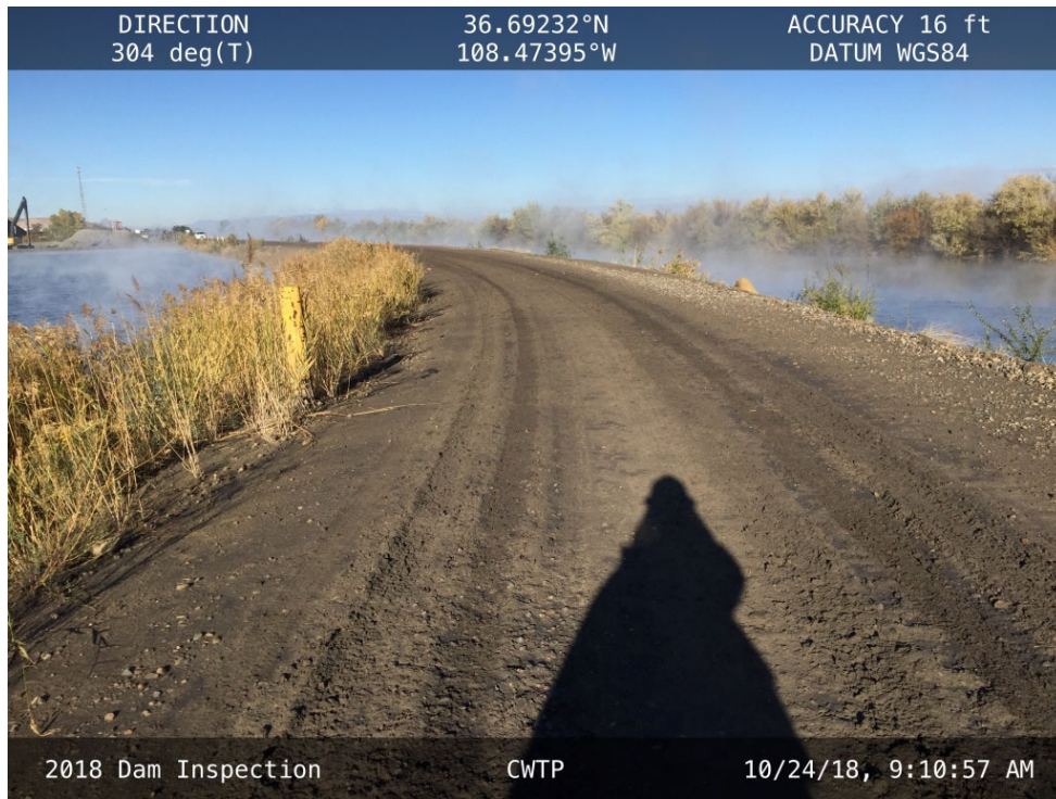
20181024 – IMG_0959 The crest of the CWTP embankment, facing west.
