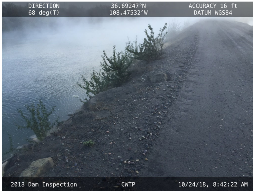
A shallow erosion rill on the downstream slope of the CWTP embankment.
