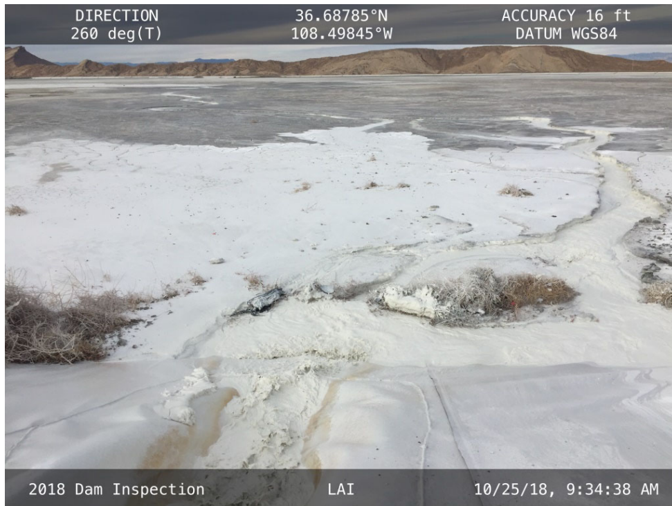
20181025 – IMG_1369 FGD sludge being deposited into the LAI from the V-ditch at the East Embankment.
