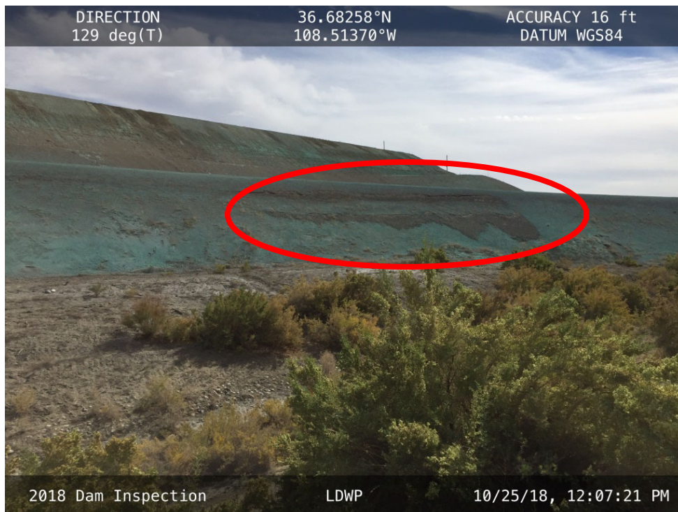
A shallow surface slough on the lowermost bench of the West Embankment.
