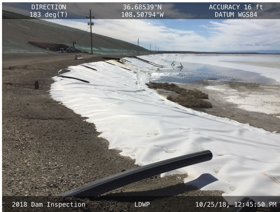
20181025 – IMG_1540 The upstream slope of the East Embankment, facing south.
