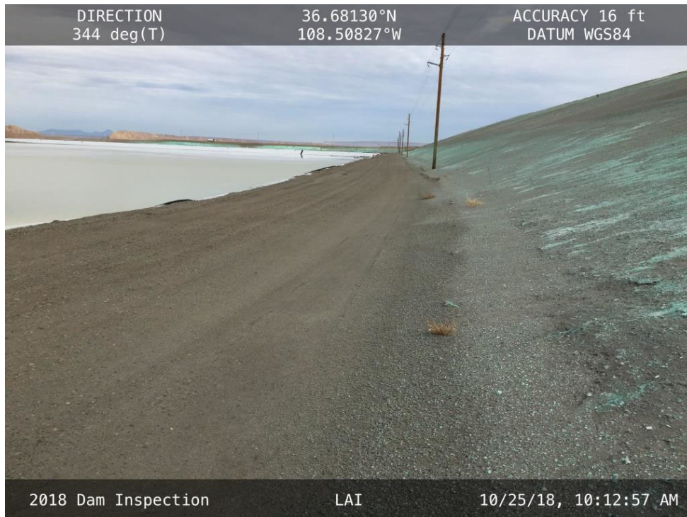
20181025 – IMG_1389 The downstream toe of the West Embankment, facing north.
