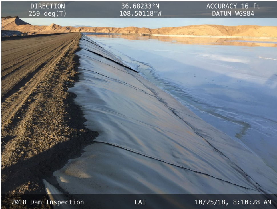
20181025 – IMG_1206 The upstream slope of the South Embankment, facing west.
