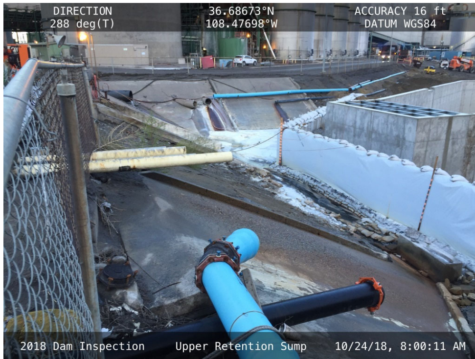
Temporary pumping equipment on the south side of the Upper Retention Sump.
