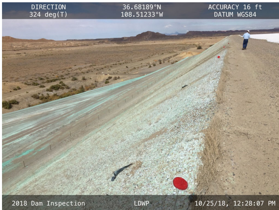
20181025 – IMG_1489 The downstream slope of the West Embankment, facing north.
