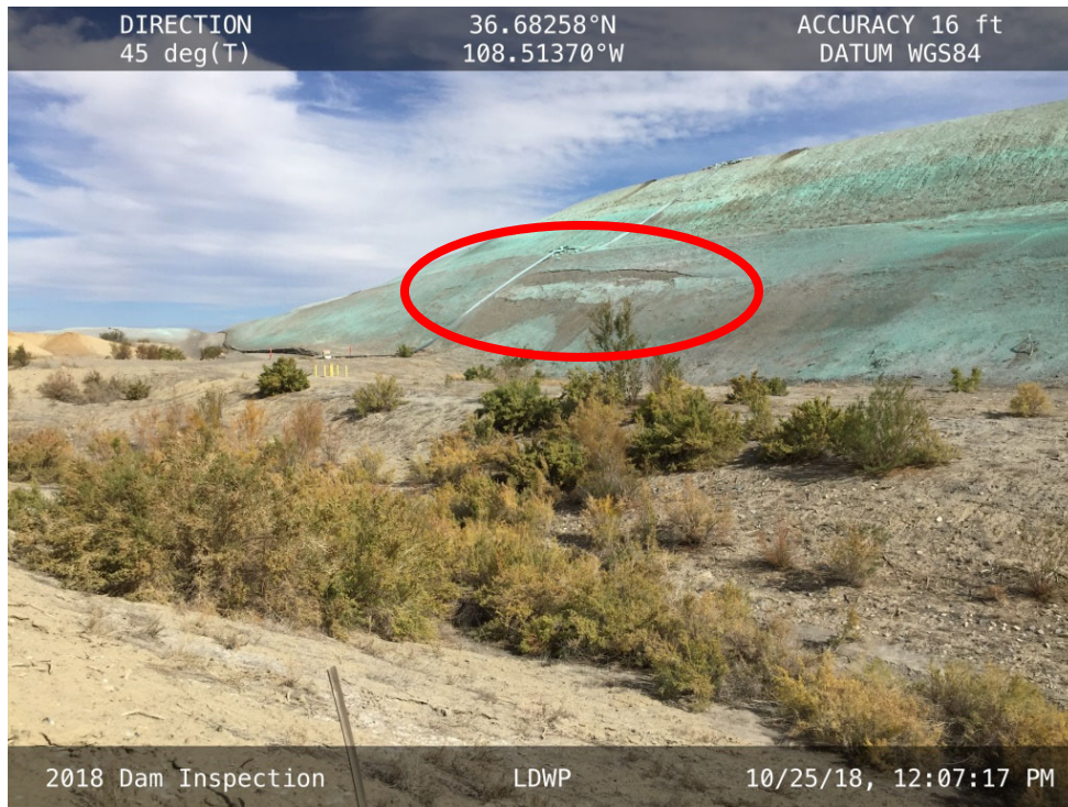
A shallow surface slough on the lowermost bench of the West Embankment.
