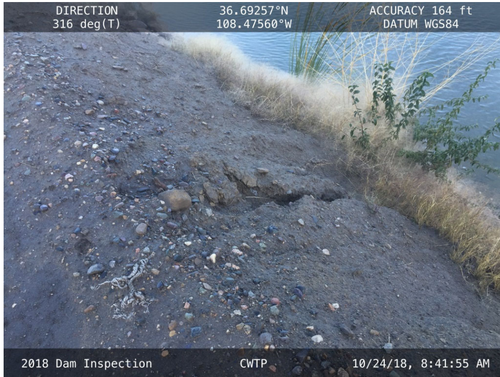
A shallow erosion rill on the downstream slope of the CWTP embankment.
