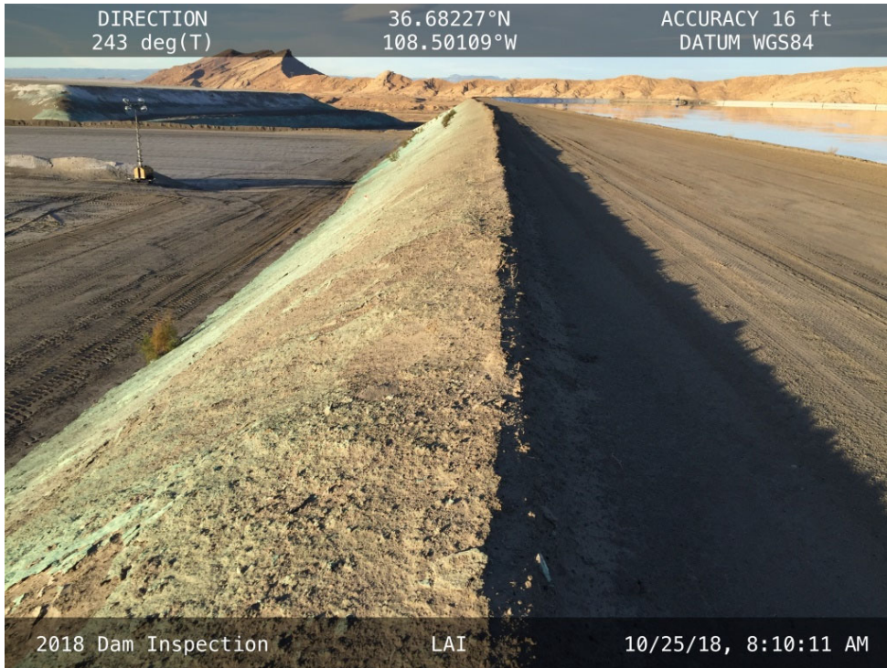
20181025 – IMG_1205 The downstream slope of the South Embankment, facing west.
