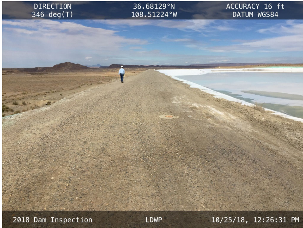
20181025 – IMG_1481 The crest of the West Embankment, facing north.
