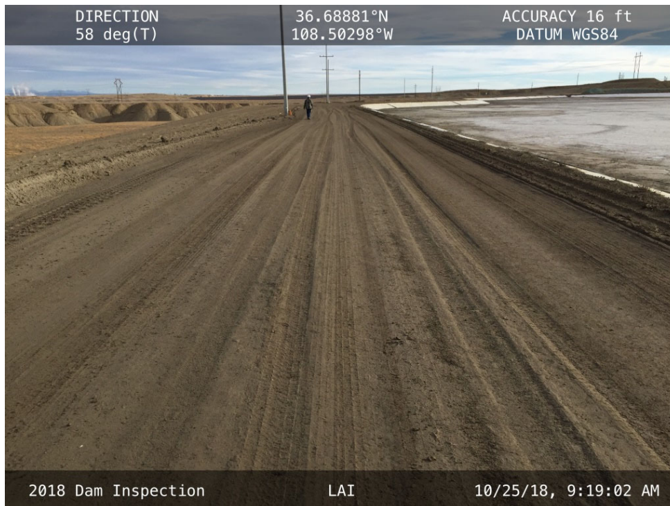
20181025 – IMG_1333 The crest of the Northwest Embankment, facing northeast.
