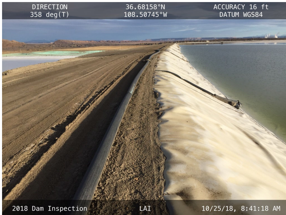
20181025 – IMG_1256 The HDPE pipe that conveys water from the pump in the Southwest Corner to the Drop Inlet Structure.
