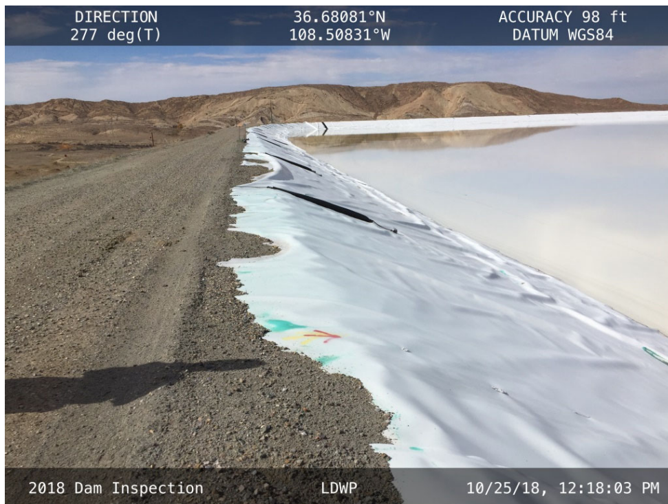
20181025 – IMG_1446 The upstream slope of the South Embankment, facing west.
