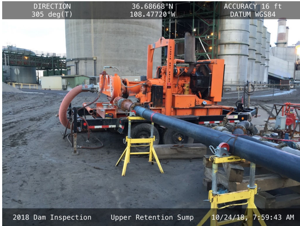
Temporary pumping equipment on the south side of the Upper Retention Sump.
