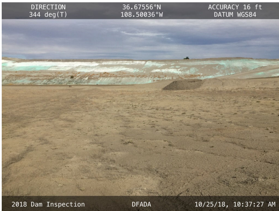
20181025 – IMG_1426 The south slope of DFADA Cells 1 and 2, facing north.
