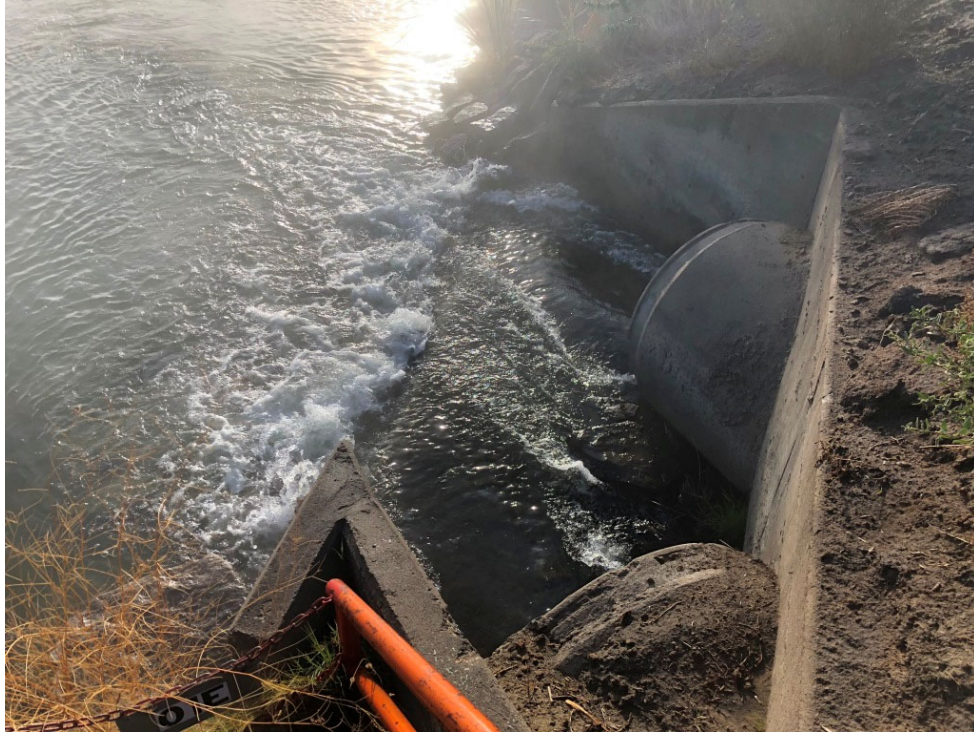
20181024 – IMG_0888 The outfall from the CWTP to the discharge canal.
