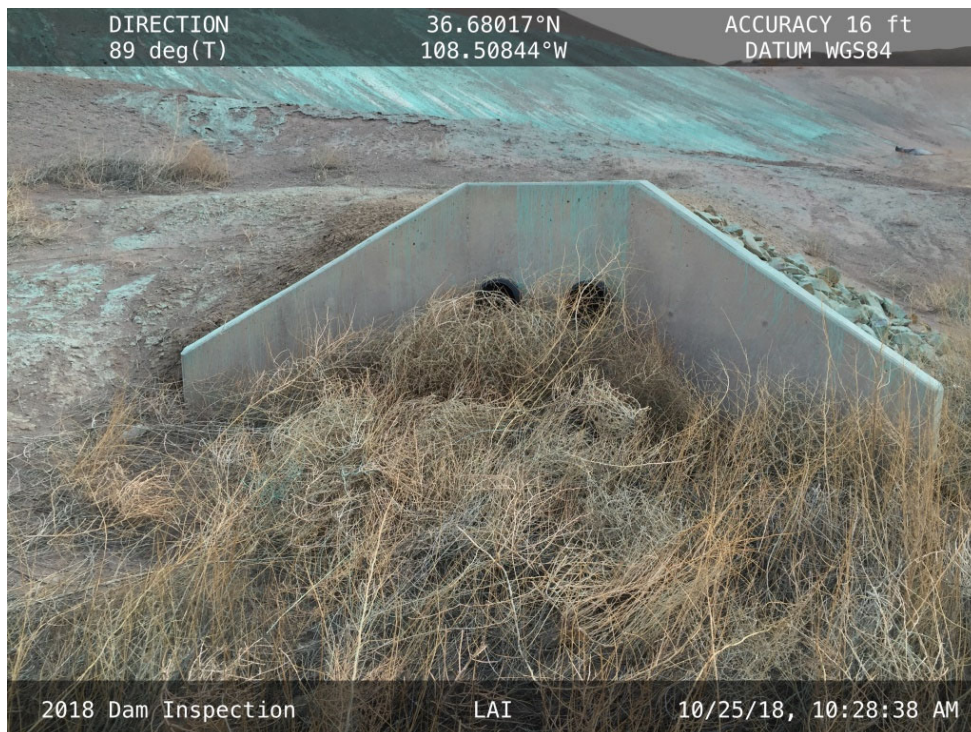
20181025 – IMG_1415 The South Embankment toe drain in a dry condition.
