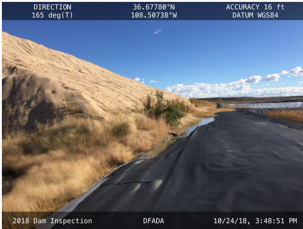
Vegetation growing in the drainage ditch and overflow channel of the leachate collection pond.
