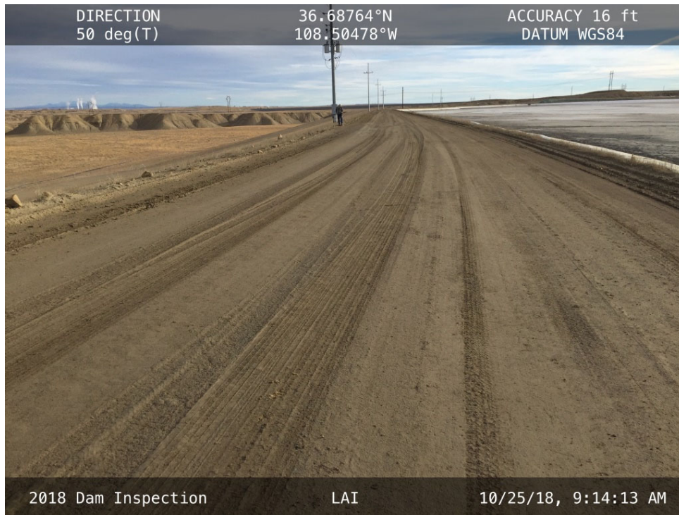
20181025 – IMG_1322 The crest of the Northwest Embankment, facing northeast.
