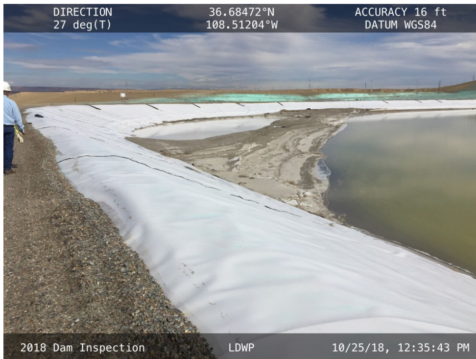
The liner pulling out of the anchor trench in the northern portion of the West Embankment.
