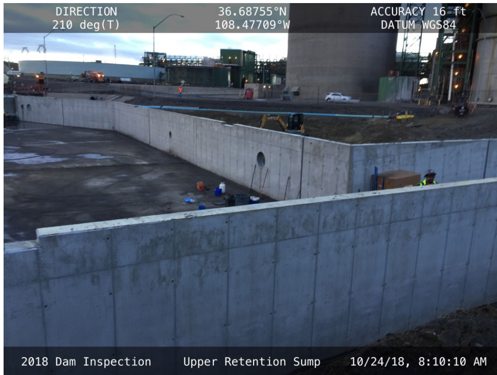
Construction of the Upper Retention Tank Sump in the URS footprint, facing south.
