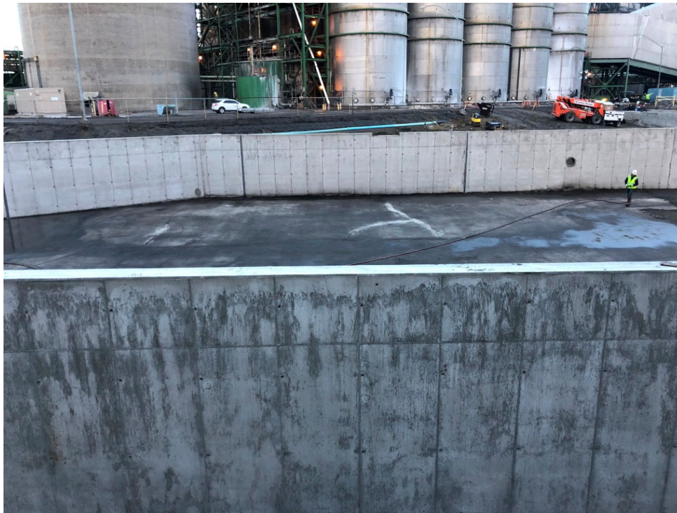
20181024 – IMG_0869 Construction of the Upper Retention Sump Tank, facing west.
