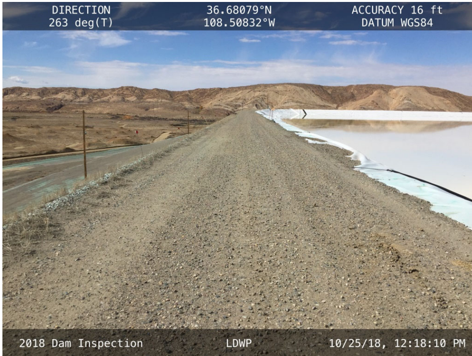
20181025 – IMG_1447 The crest of the South Embankment, facing west.
