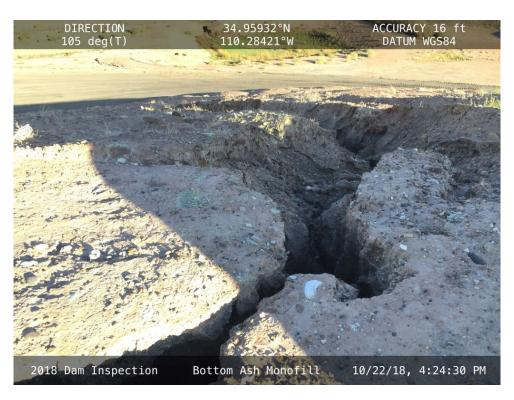
${\bf 20181022-IMG\_0565}$  An erosion gully on the east side of the Bottom Ash Monofill requiring repair.
