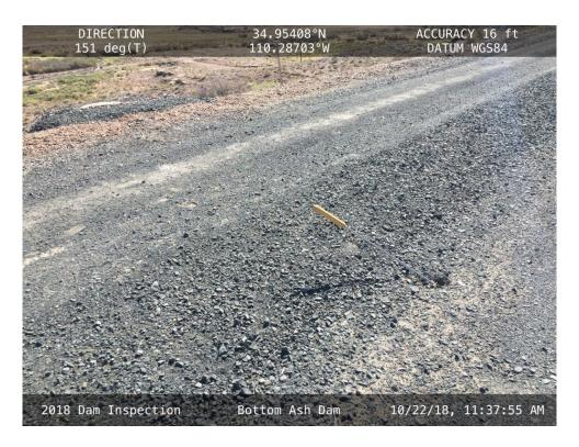
20181022 – IMG\_0343 Additional erosion hole near settlement monument M-16.
