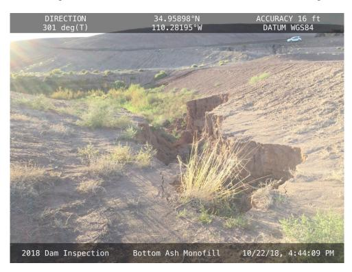
$20181022-IMG\_0626$  Headcutting on the east side of the Stormwater Detention Basin, facing west.
