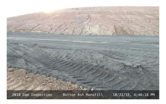
$20181022-IMG\_0628$  Minor erosion rills along the eastern side of the Bottom Ash Monofill, facing west.
