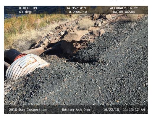
$20181022-IMG\_0283$  Shallow erosion on the upstream slope and crest near the western siphon line.
