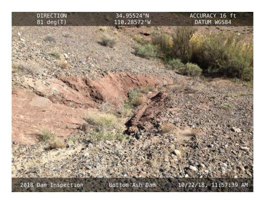
${\bf 20181022-IMG\_0381}$  A second erosion gully on the downstream slope of the East Embankment.
