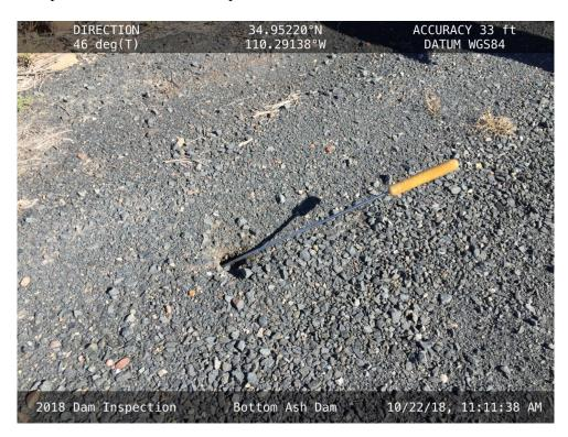
**20181022 – IMG\_0281**Shallow erosion hole on the South Embankment crest.
