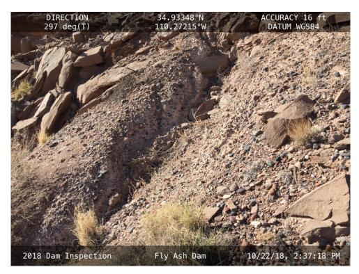
20181022 – IMG\_0502 Minor erosion at the Northwest Abutment contact.
