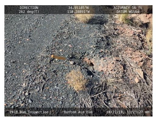
$20181022-IMG\_0304$  Minor erosion hole on the downstream side of the South Embankment crest.
