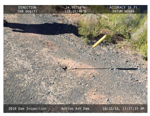
$20181022-IMG\_0325$  An erosion hole in the crest at the southeast corner of the Bottom Ash Dam.
