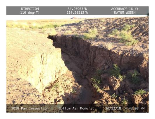
20181022 – IMG\_0620 Headcutting on the east side of the Stormwater Detention Basin, facing east.
