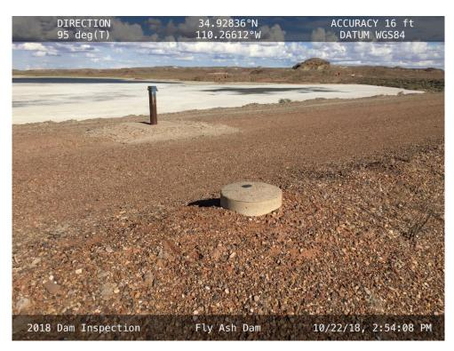
$\label{eq:condition} 20181022-IMG\_0512$  A piezometer and a settlement monument along the crest.
