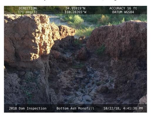
$20181022-IMG\_0607$  Significant erosion in the northwest corner of the Stormwater Detention Basin, facing south.
