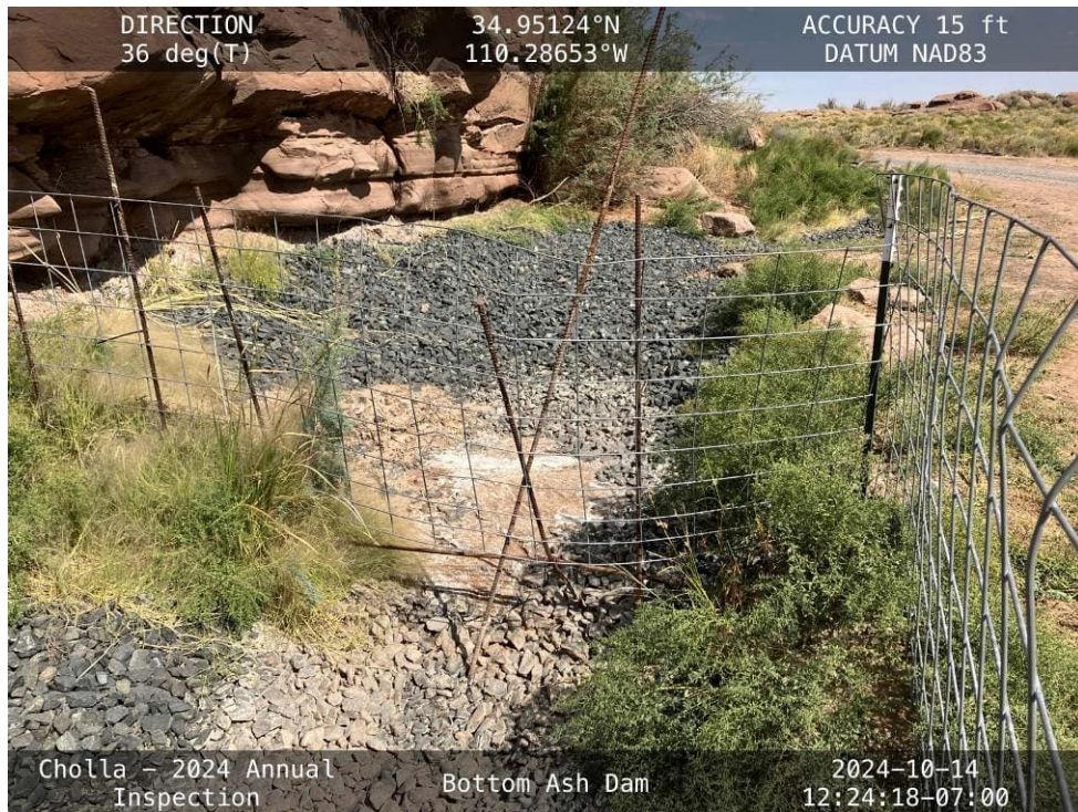
20241014 – IMG_6355 The ditch adjacent to the Petroglyph Seep, regraded since the 2023 inspection.
