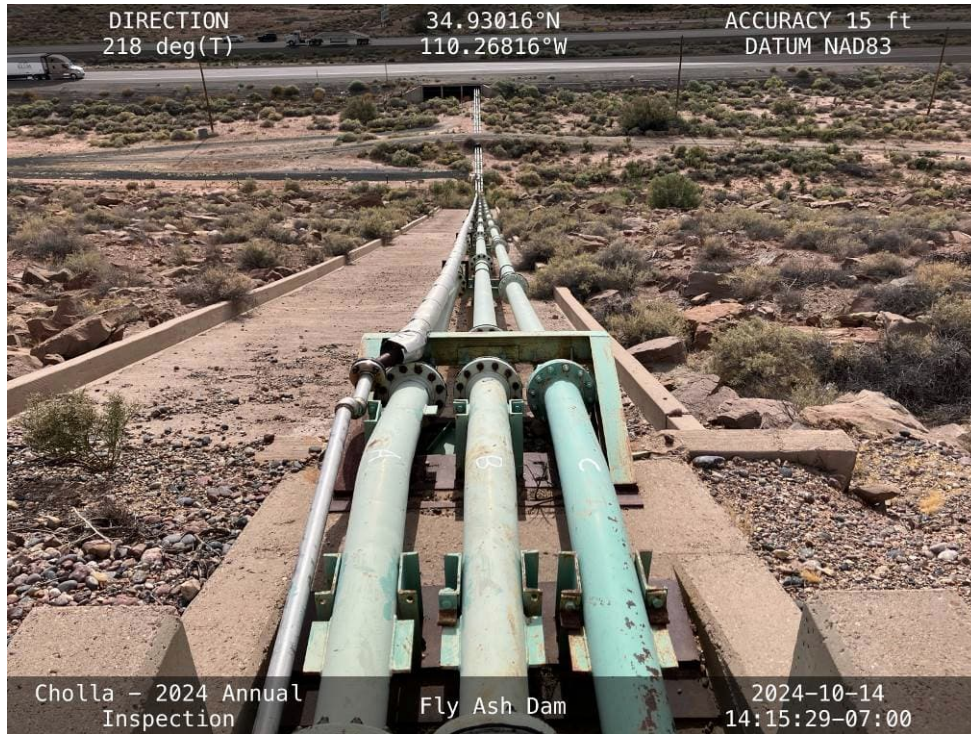
20241014 – IMG_6476 The inlet pipes along the downstream slope.
