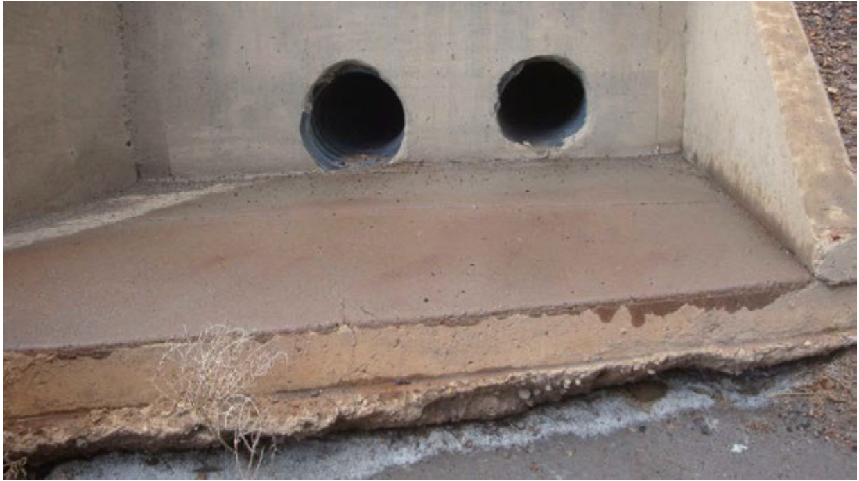
20151016 – Photo 3 Downstream slope. Outlet to Tanner Wash.
