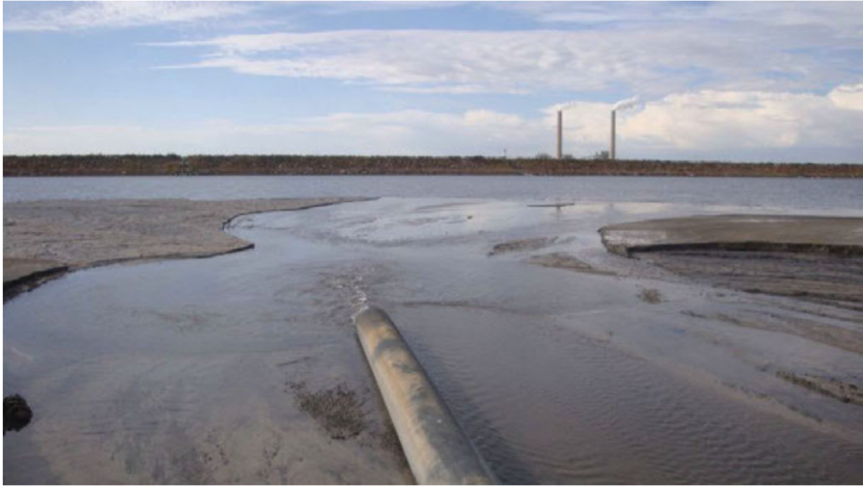
20151016 – Photo 48 Impoundment. Decant from settling cell to free water reclaim pond.
