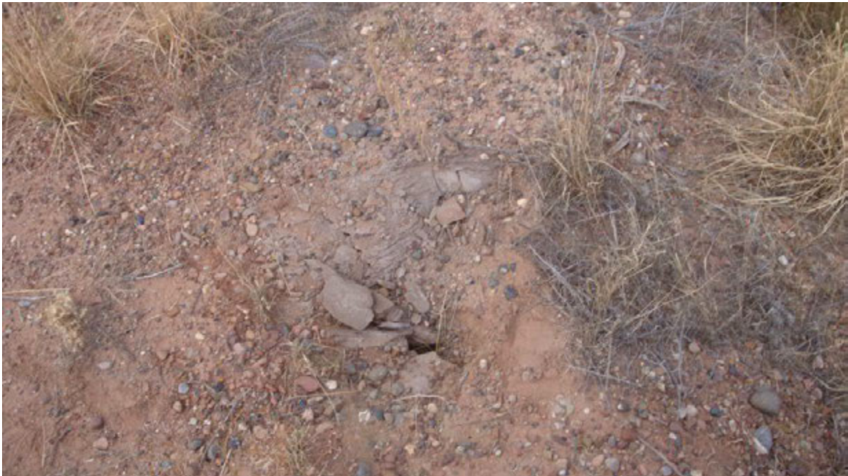
20151016 – Photo 10 Crest. Apparent minor animal burrow.
