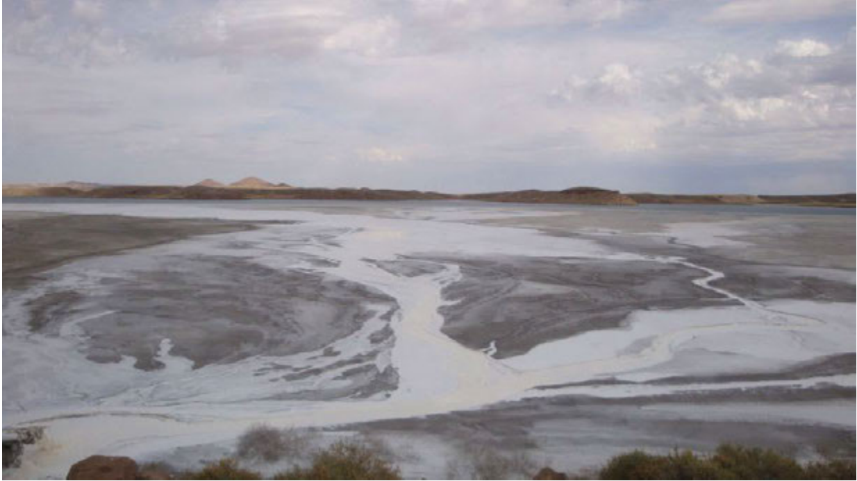
20151016 – Photo 15 Impoundment. Beach created by deposition at upstream slope of dam.
