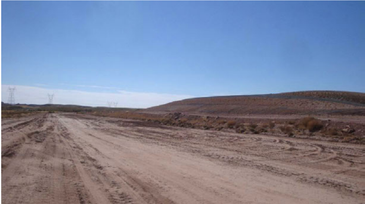
20151016 – Photo 11 Lateral expansion finished grade. Ready to receive bottom ash.
