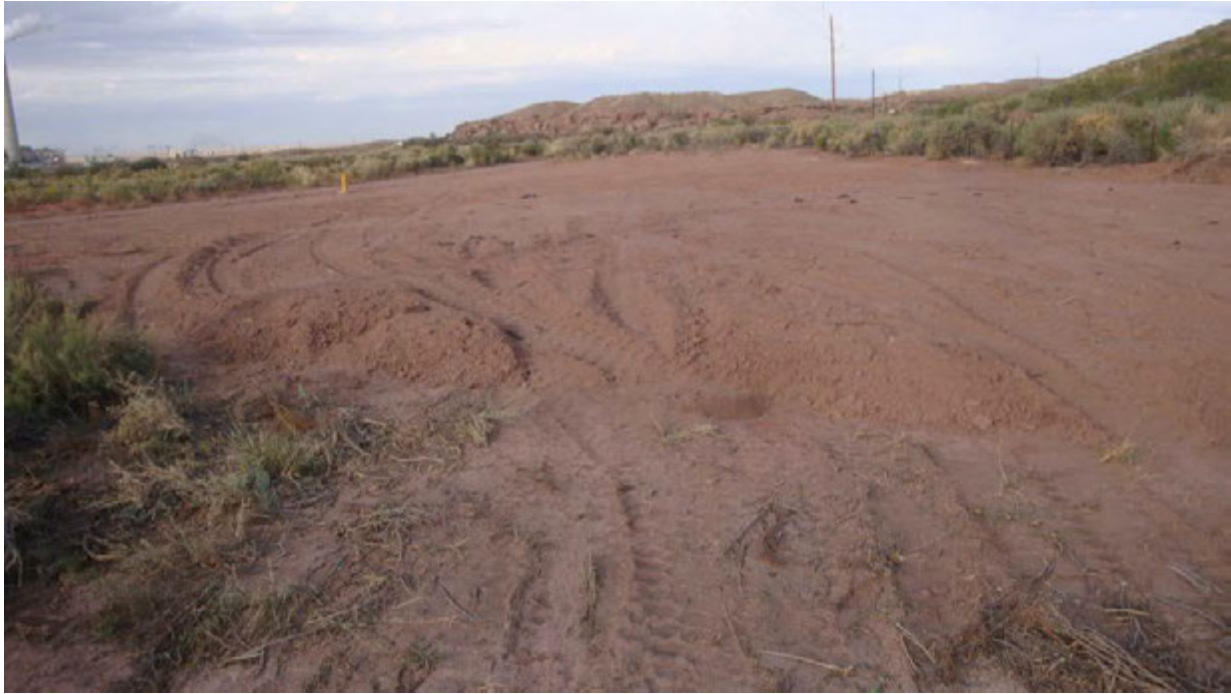
20151016 – Photo 20 Downstream slope. Toe area clearing for planned monitoring well.
