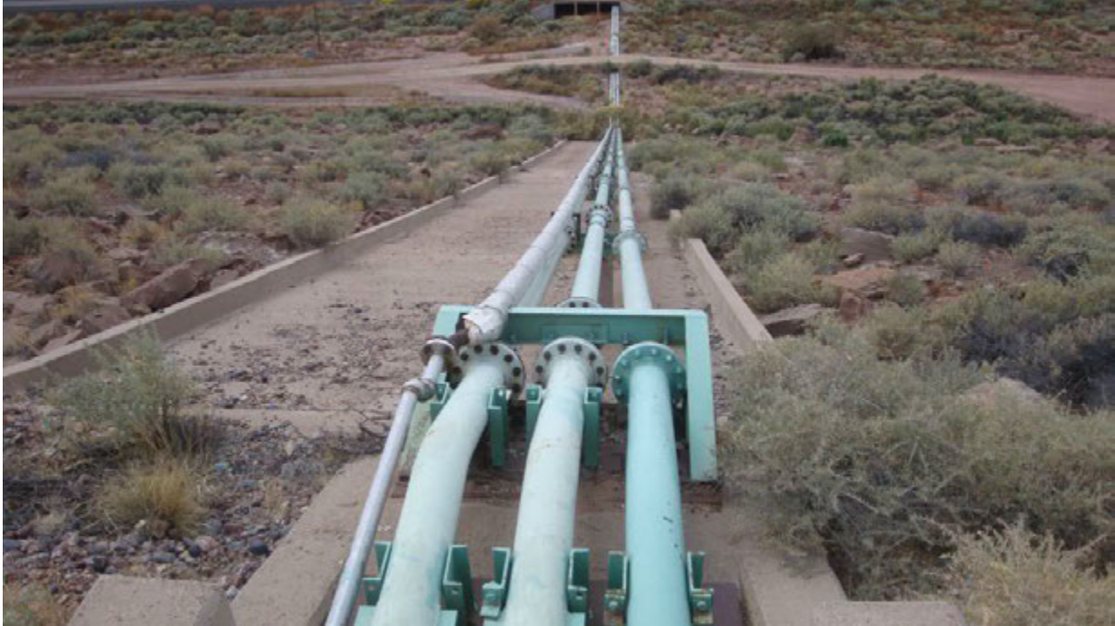
20151016 – Photo 11 Downstream slope. FGD/ash lines. Vegetation generally less than 3 feet high.
