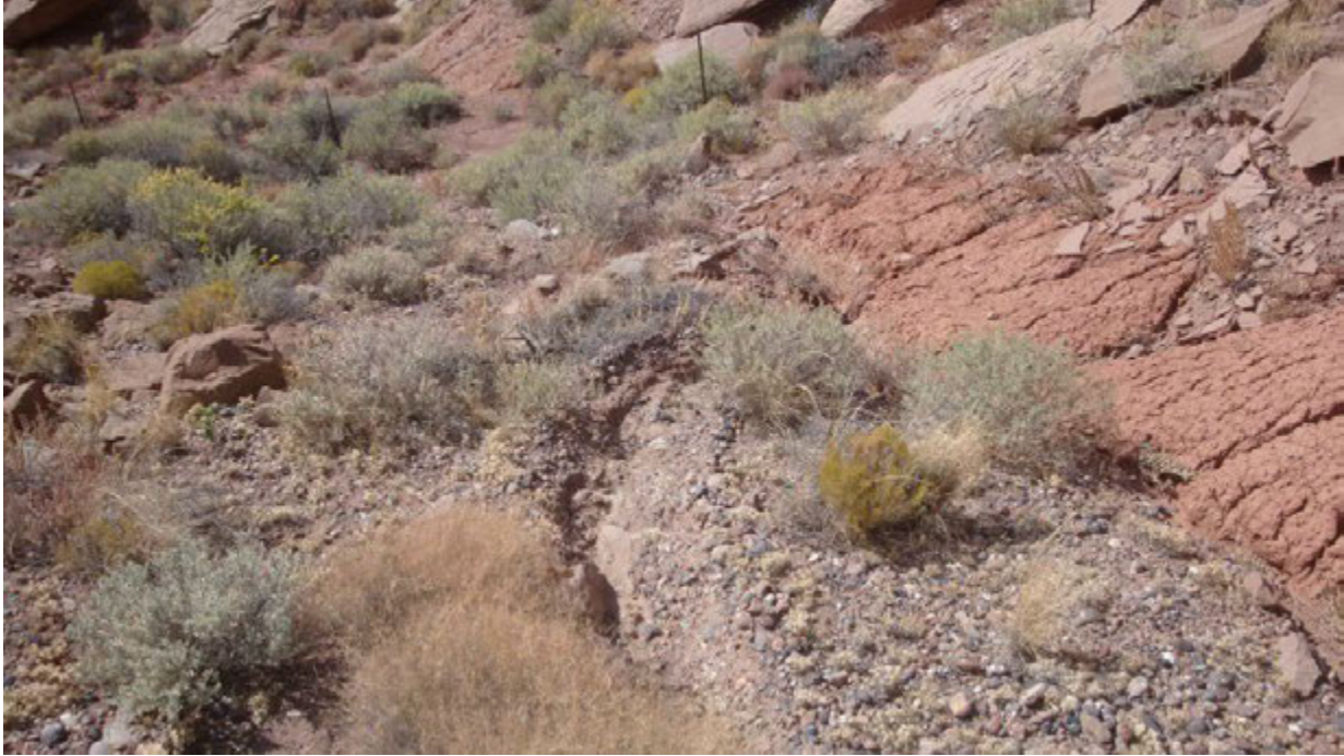
20151016 – Photo 8 Downstream slope, right abutment groin. Erosion at contact.
