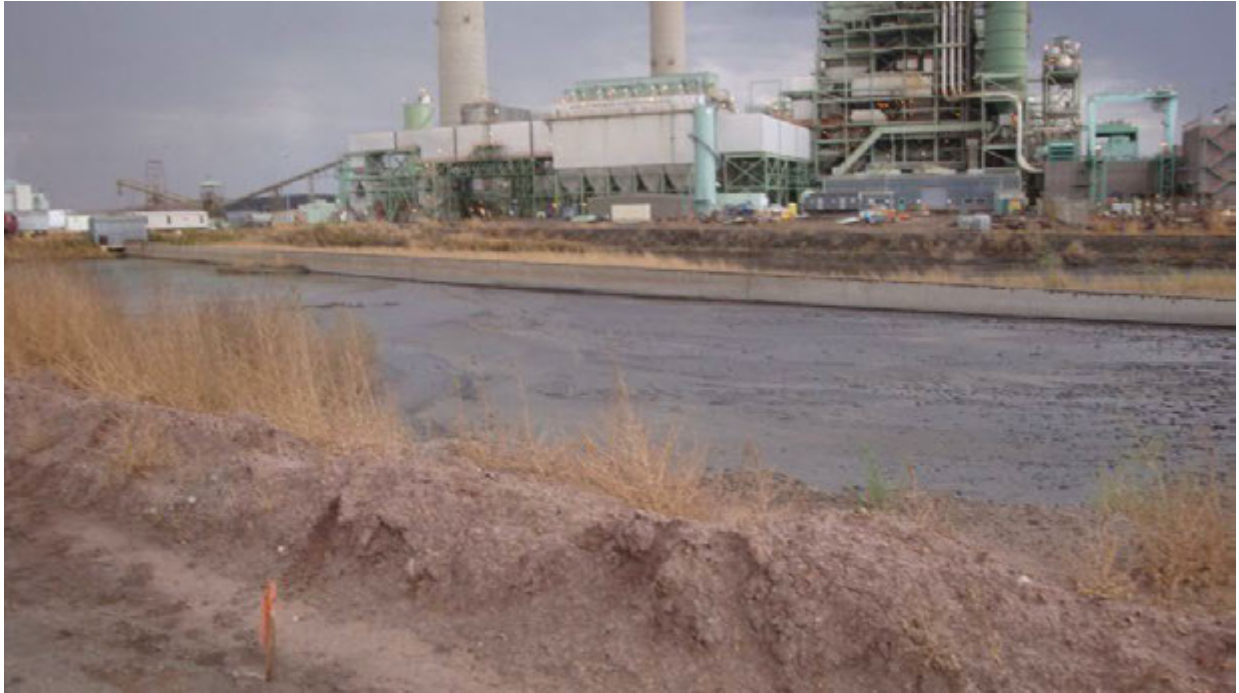
20151016 – Photo 1 Sedimentation Pond. View across pond to northeast.
