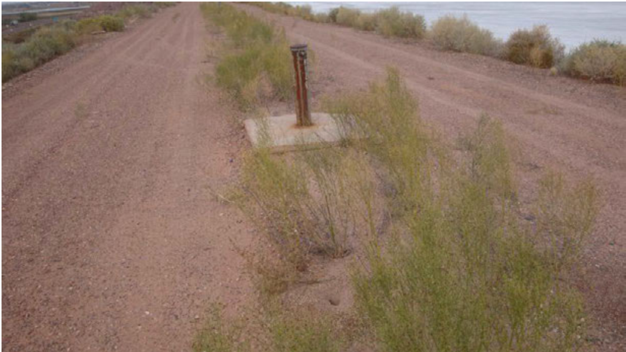
20151016 – Photo 18 Crest. Piezometer completion.
