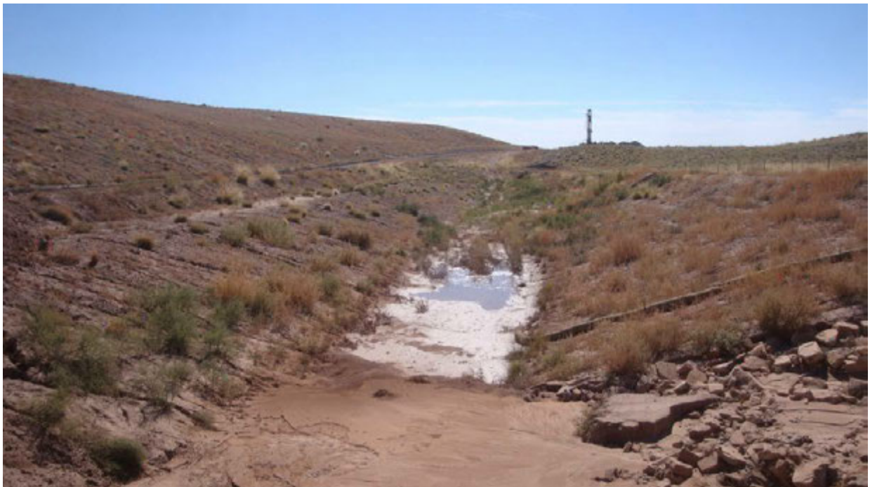
20151016 – Photo 21 Run-on diversion channel. Looking up-gradient. Partially blocked by debris side drainage.
