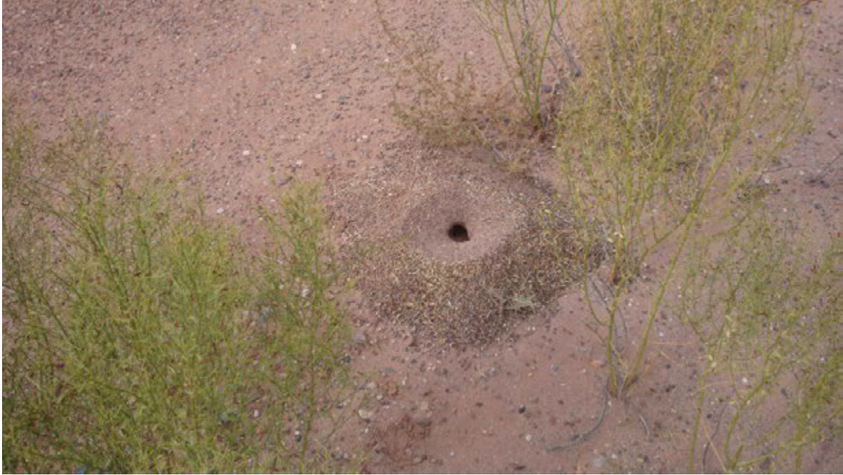
20151016 – Photo 17 Crest. Apparent minor animal burrow.
