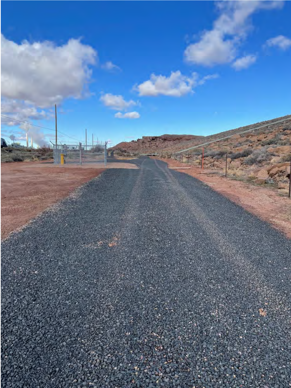
Figure 24: Final Gravel Road at Geronimo looking west
