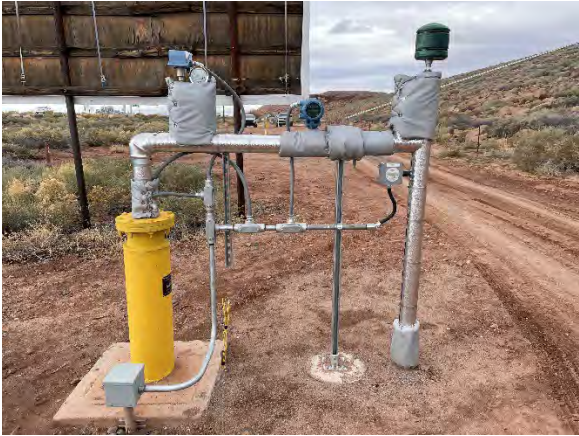
EW-01 final insulation
