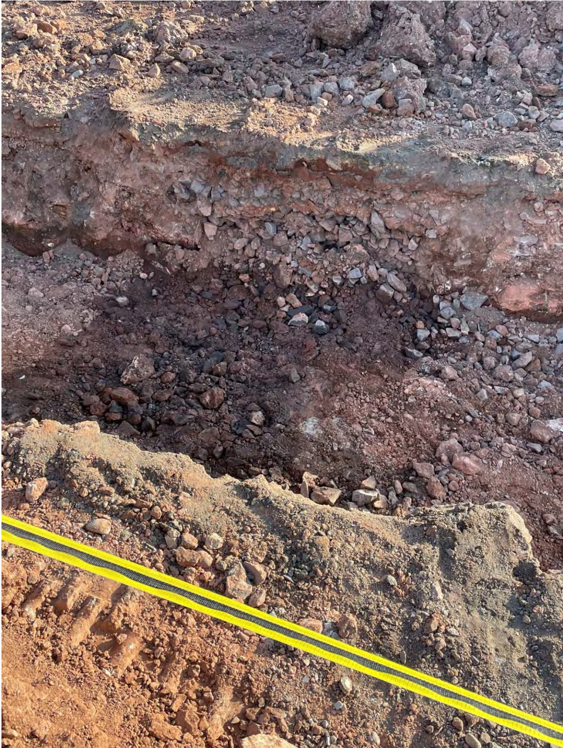
Figure 1: Existing Seepage Trench Crossing
