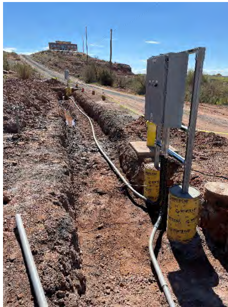
looking east – HDPE and conduit trench
