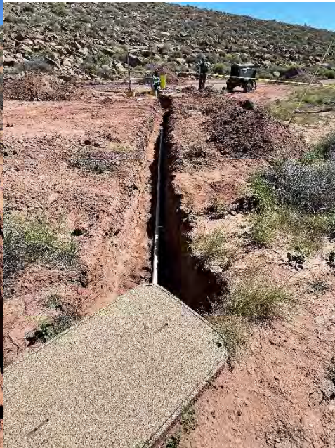
electrical tie into box
