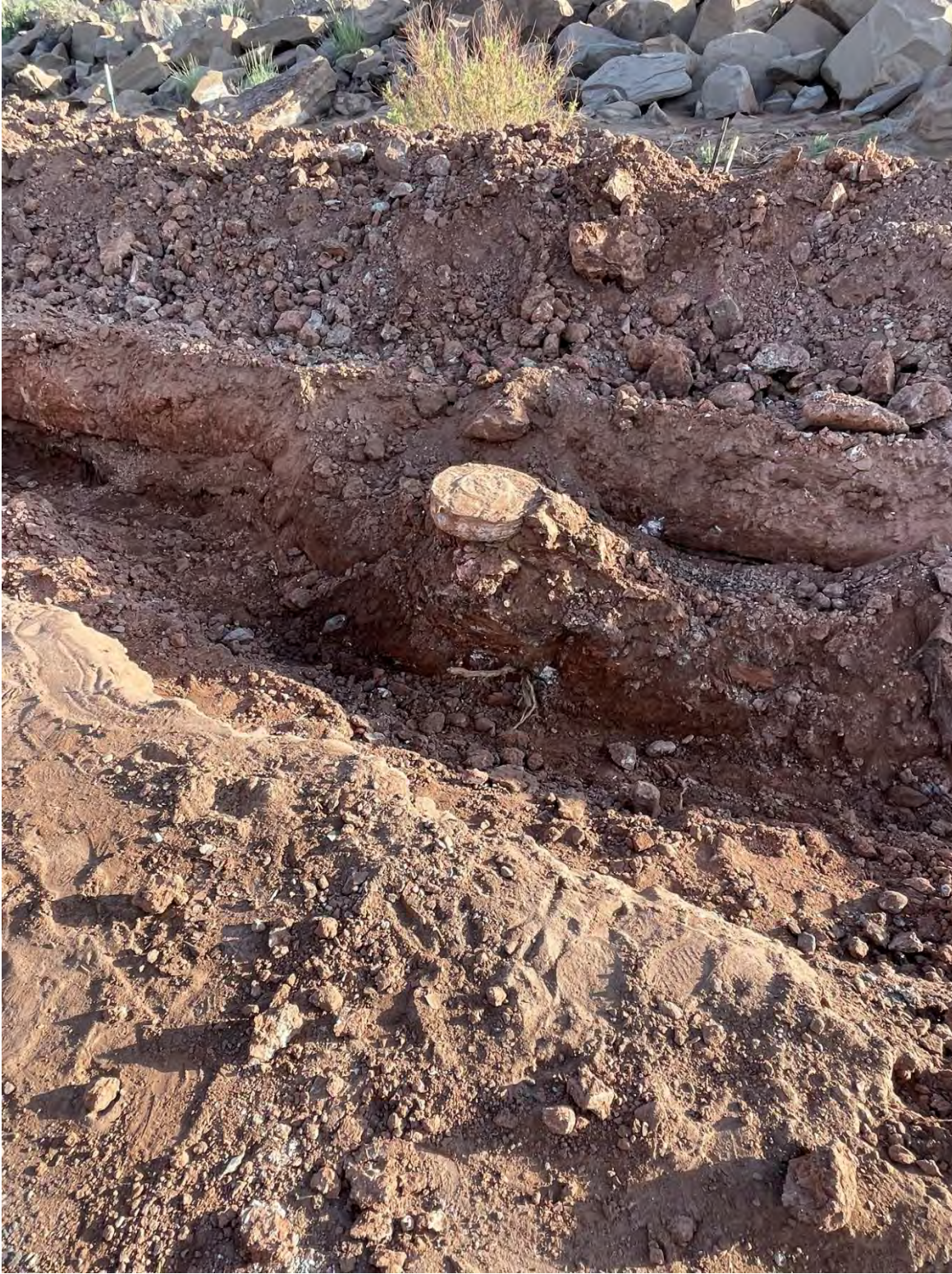
Figure 2: Unknown Monitoring Well discovered during trench excavation
