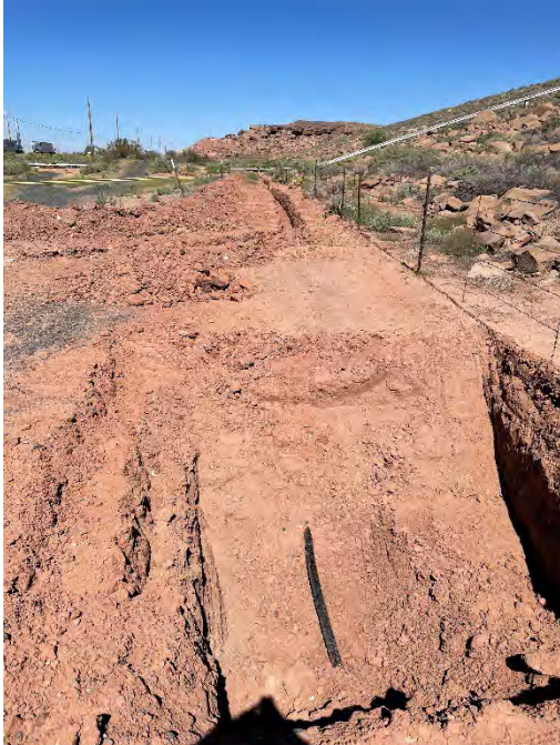
Located HDPE feed line
