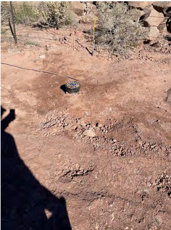
Valve cap/boxes that will need concrete collars
