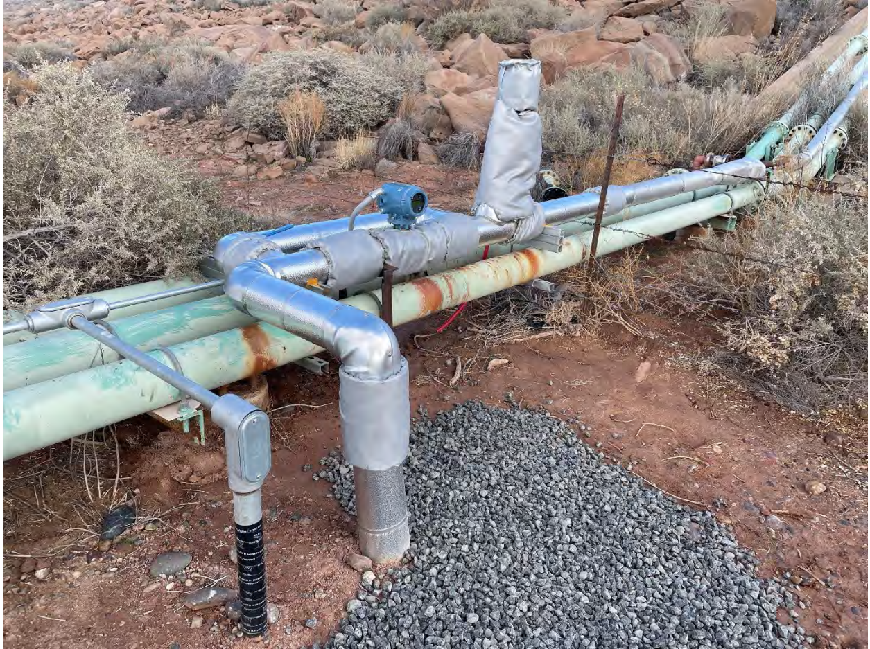
Figure 17: Combined Hunt-Geronimo Flowmeter completed
