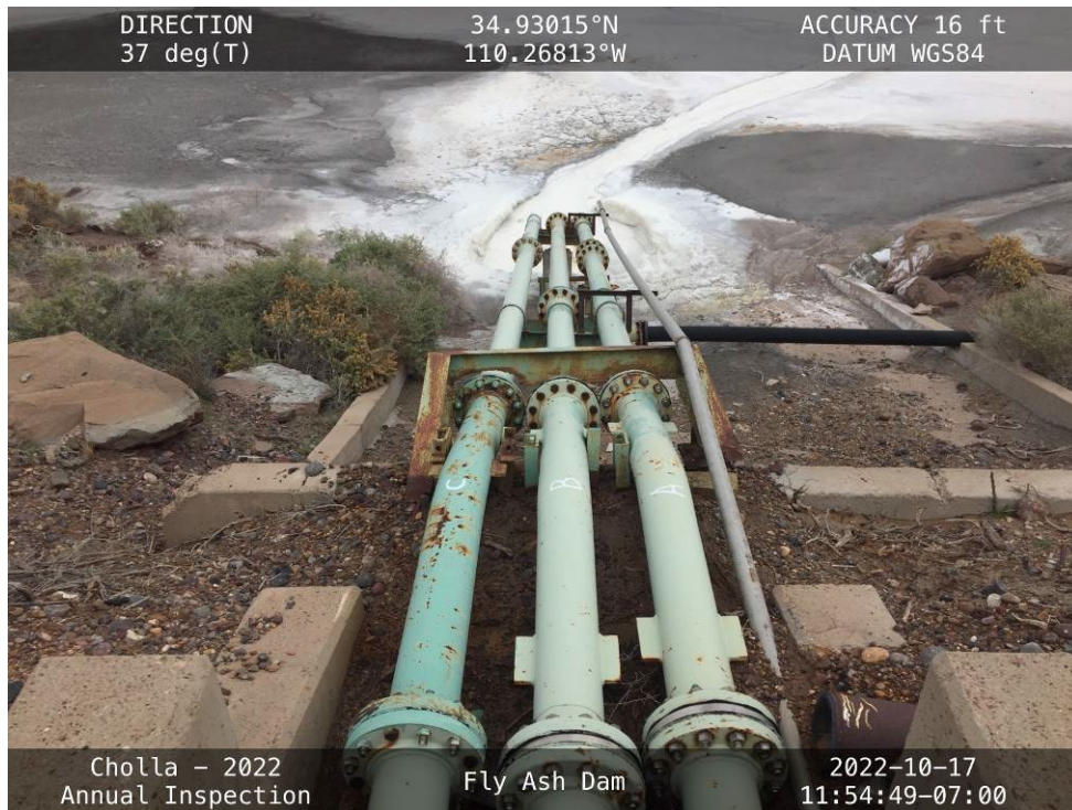
20221017 – IMG_3431 The inlet pipes along the upstream slope.
