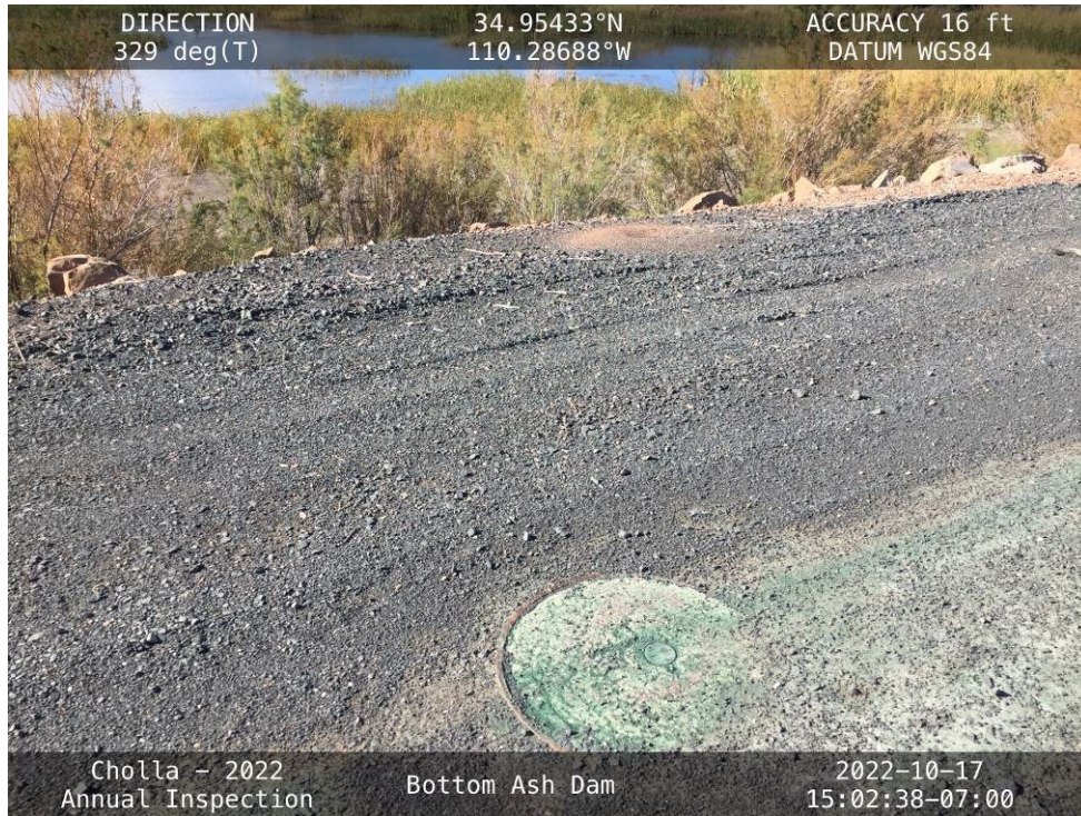
20221017 – IMG_3627 An ant hill on the upstream shoulder near Monument PI.
