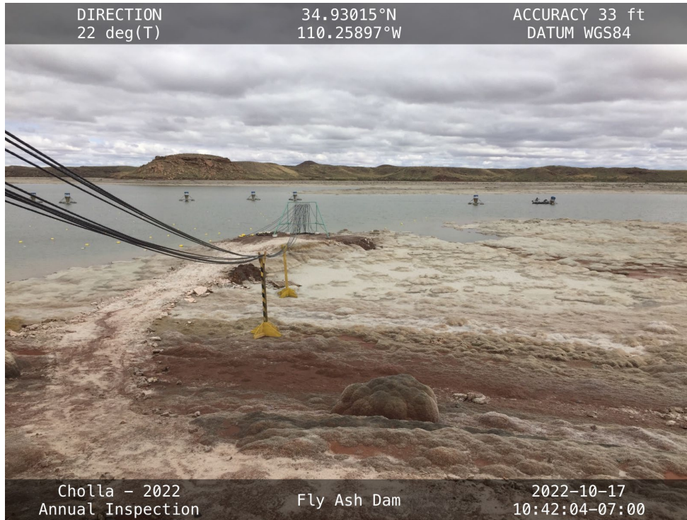
Downdraft evaporators in the Fly Ash Pond. One evaporator being removed for repairs.
