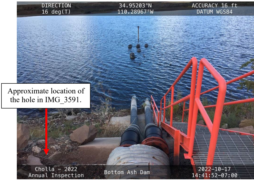
The central siphon lines along the upstream slope of the South Embankment.
