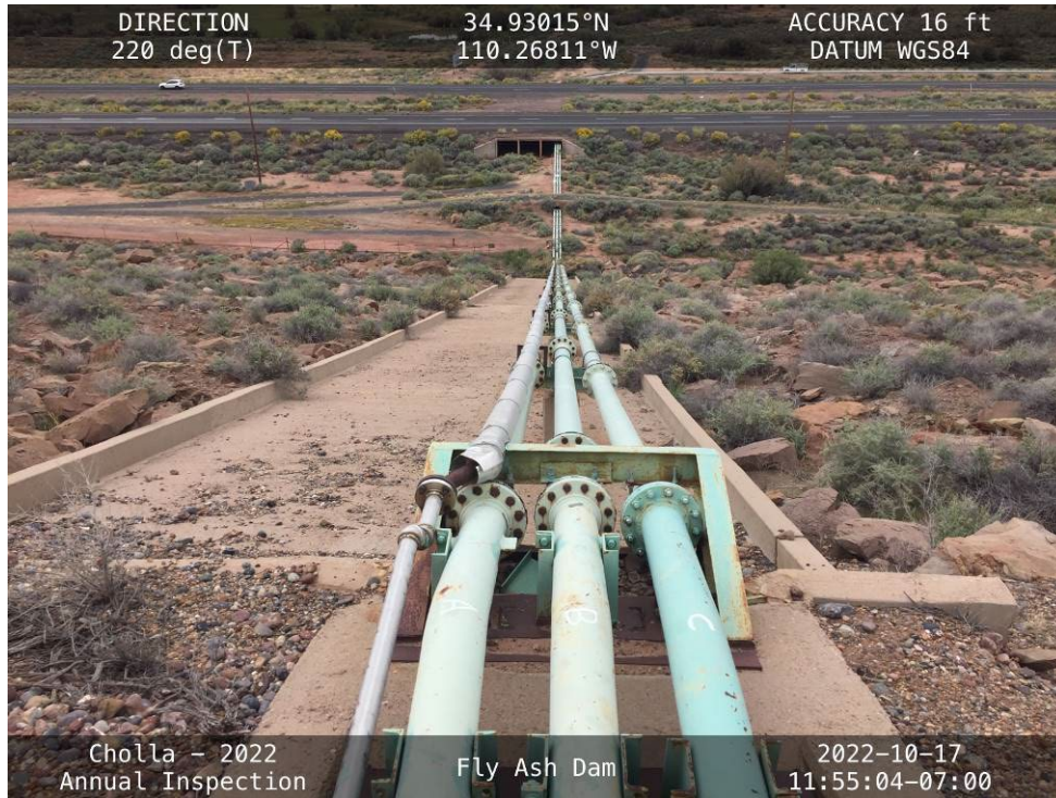
20221017 – IMG_3435 The inlet pipes along the downstream slope.
