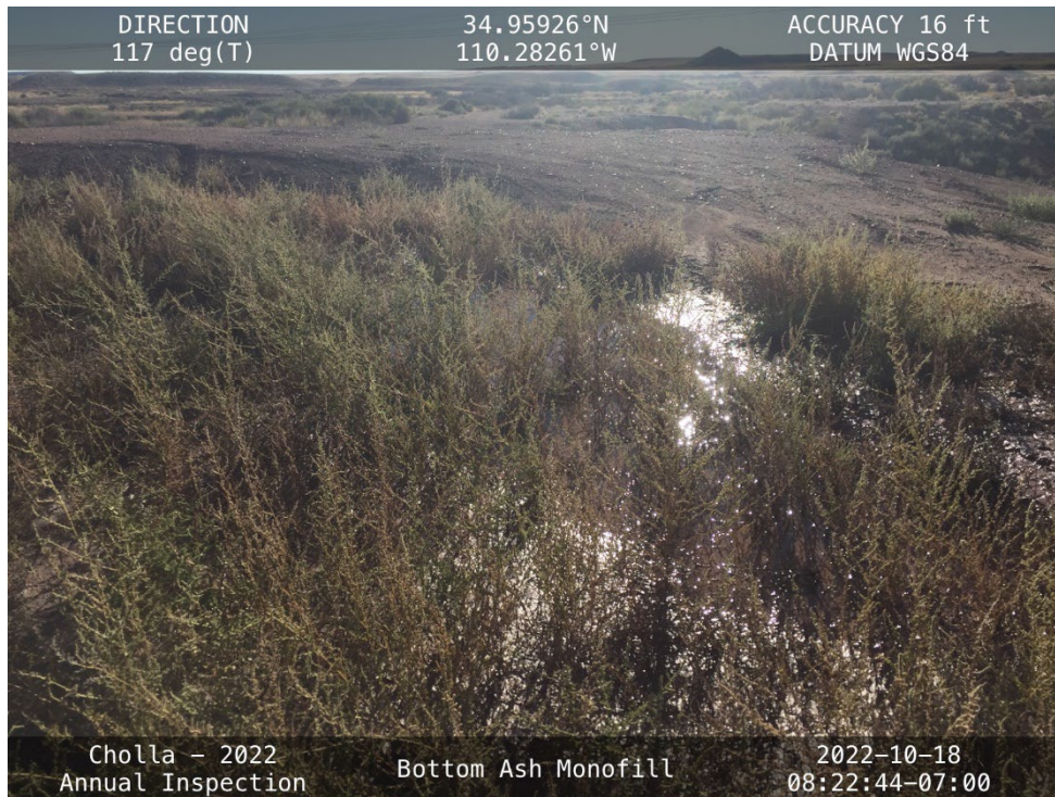
Standing water in the perimeter drainage channel on the north side of the BAM.
