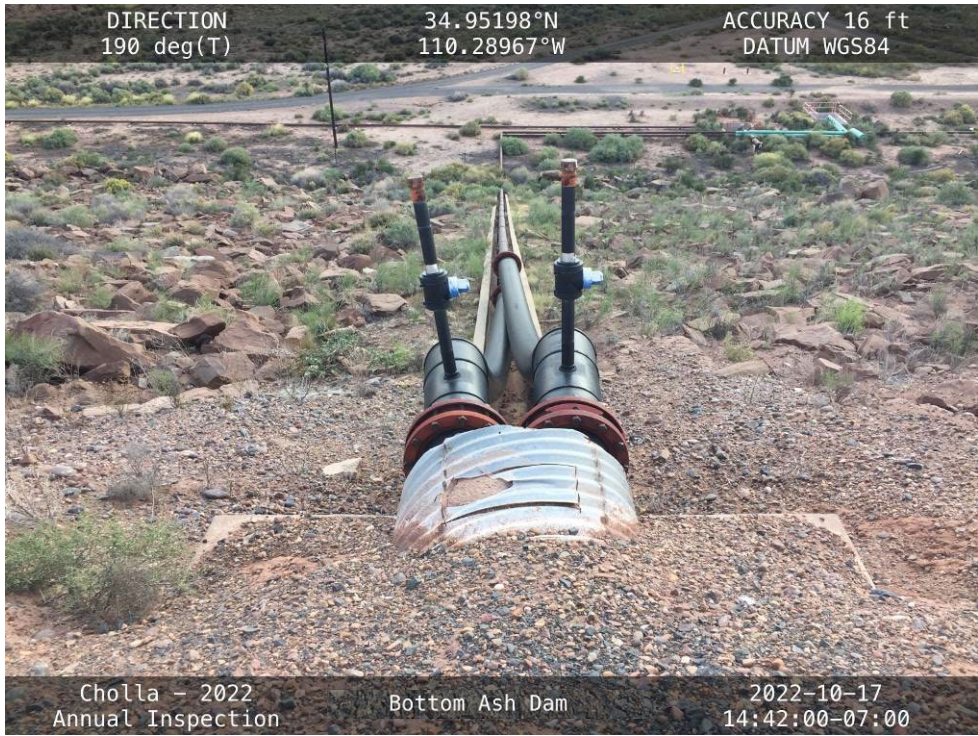
The central siphon lines along the upstream slope of the South Embankment.
