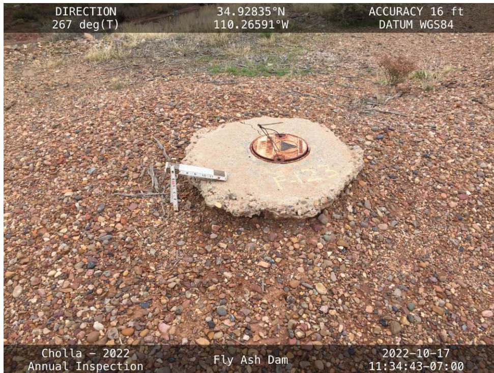
Erosion around piezometer F-123 on the downstream shoulder of the West Embankment crest.
