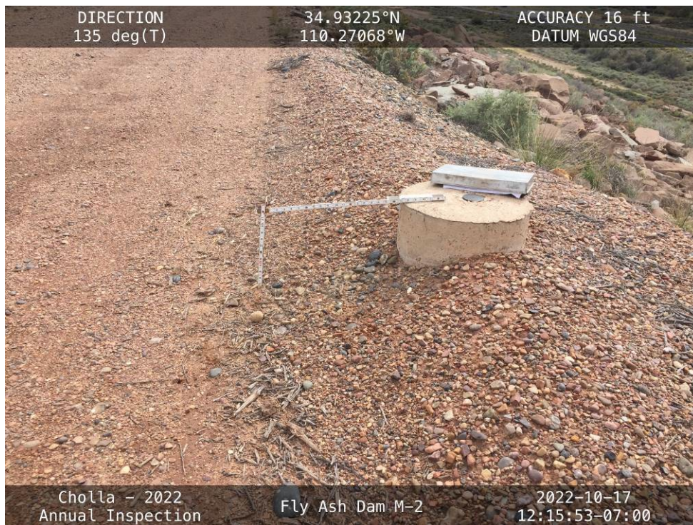
20221017 – IMG_3458 Settlement monument M-2 on the crest of the West Embankment.
