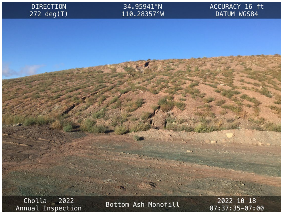
20221018 – IMG_3730 An erosion gully at the top and east side of the BAM with sediment at the toe.
