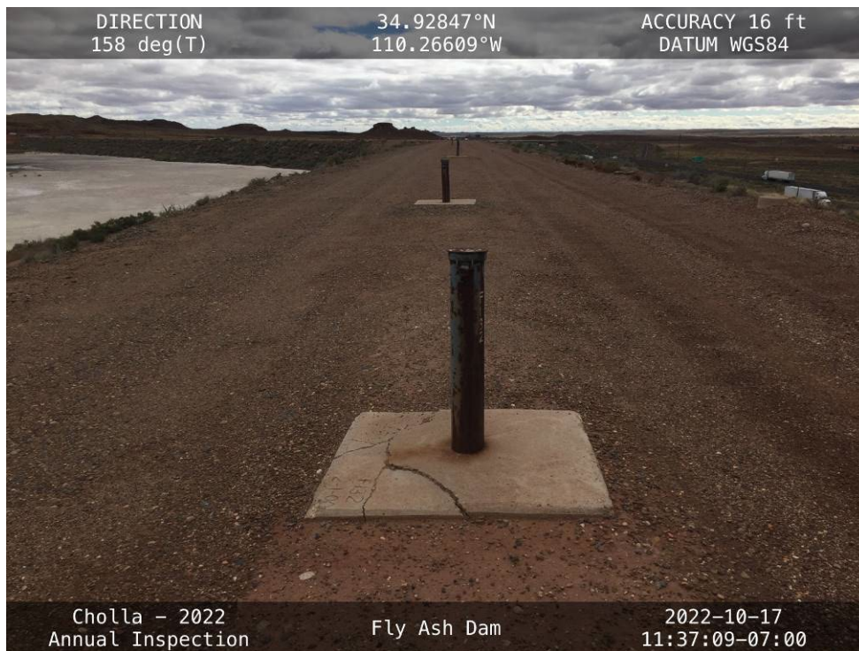
Erosion around piezometer F-123 on the downstream shoulder of the West Embankment crest.
