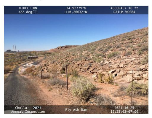
$20211025-IMG\_6874$  Area of historic erosion along the downstream toe of the West Embankment.
