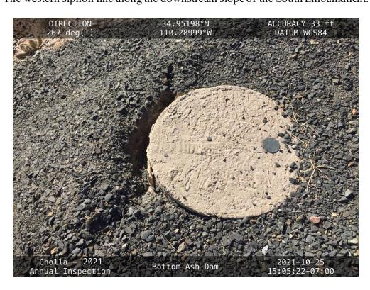
${\bf 20211025-IMG\_7006}$  The support material on the downstream side of M-13 starting to separate from the concrete.
