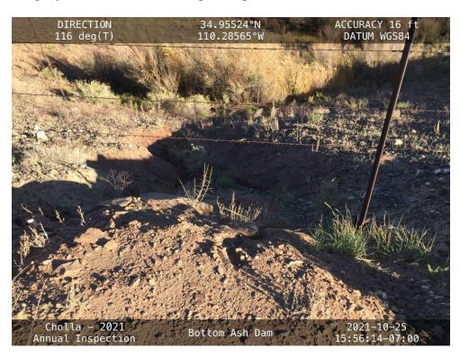
$20211025-IMG\_7127$  An erosion gully on the downstream slope along the northern half of the East Embankment.
