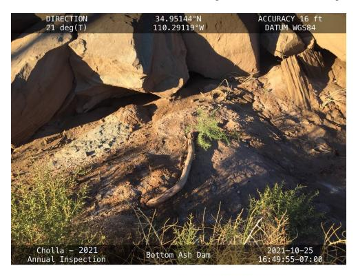
20211025 – IMG\_7191 Riprap deterioration along the South Embankment toe.
