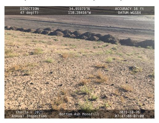
$20211026-IMG\_7283$  An incipient erosion rill on the eastern slope near the top of the BAM.
