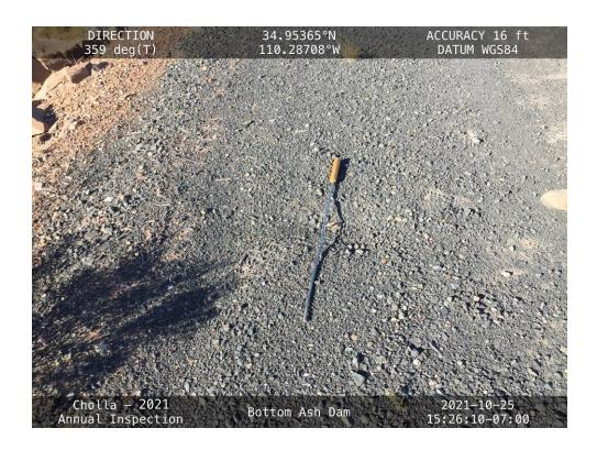
${\bf 20211025-IMG\_7052} \\ {\rm A~2.5-inch-deep~depression~along~the~upstream~shoulder~of~the~East~Embankment.}$
