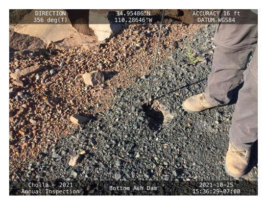
$\label{eq:continuous} 20211025-IMG\_7073$  A hole on the downstream shoulder of the East Embankment crest.
