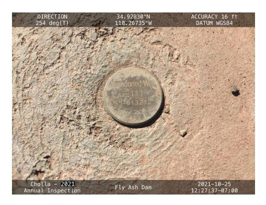
20211025 – IMG\_6885 The well abandonment marker for piezometer F-111 set in May 2021.
