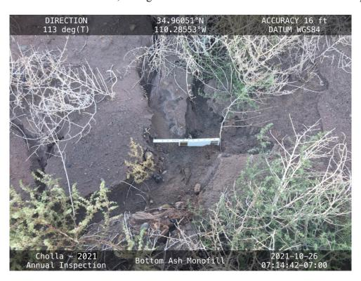
$20211026-IMG\_7223$  Erosion gullies along the western toe of the BAM. The ruler is 13 inches long.
