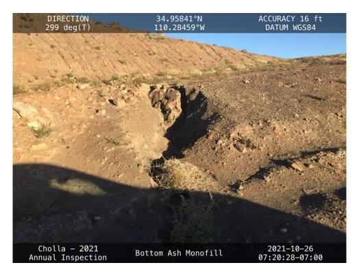
20211026 – IMG\_7229 An erosion gully on the southeast side of the BAM requiring repair.
