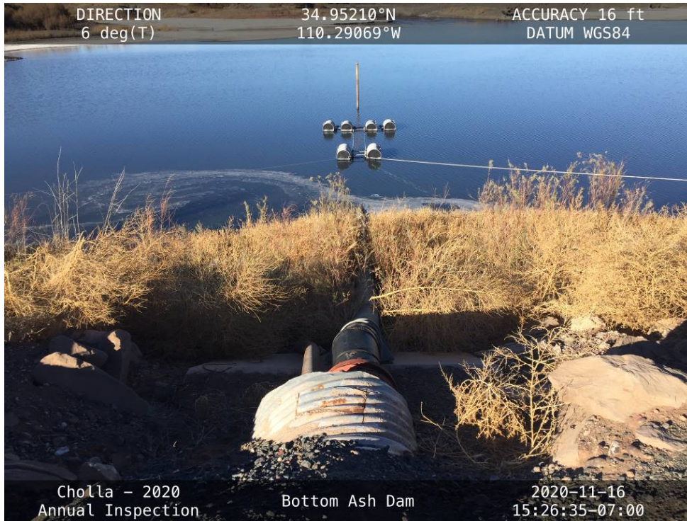
The western siphon line along the upstream slope of the South Embankment.
