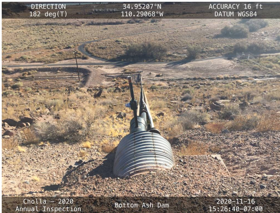
The western siphon line along the upstream slope of the South Embankment.
