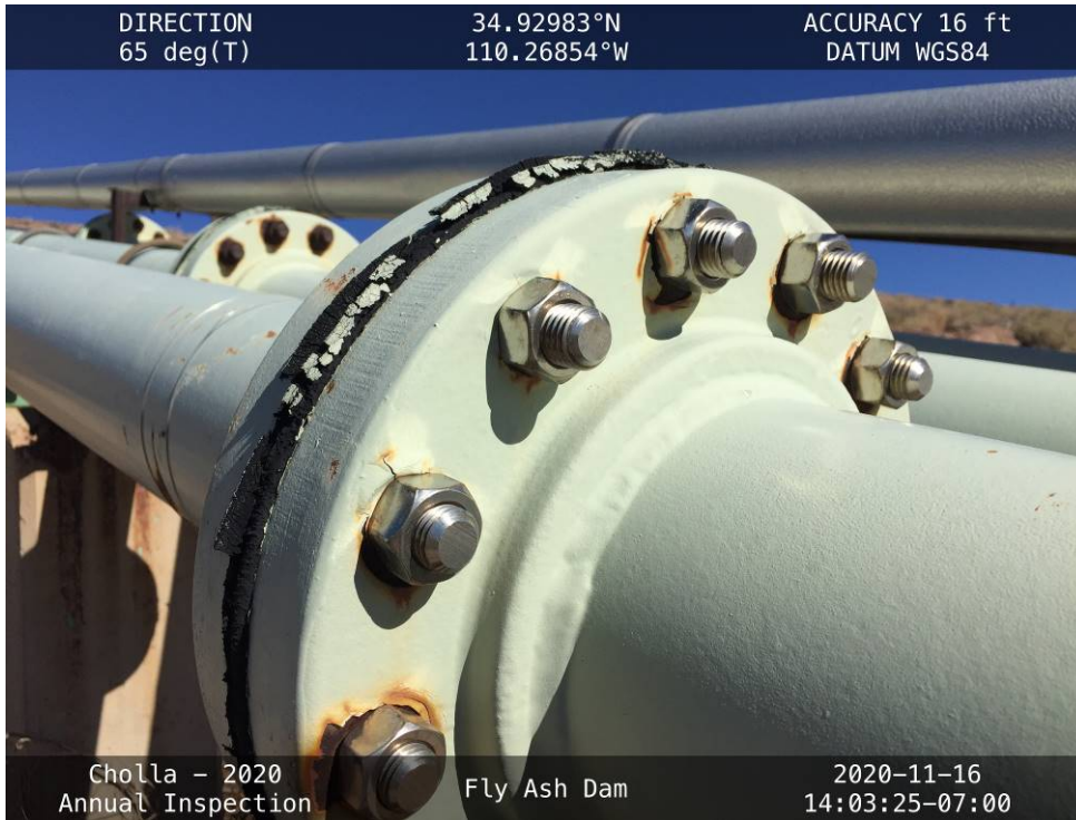
20201116 – IMG_2556 New bolts installed on the return water line pipe.
