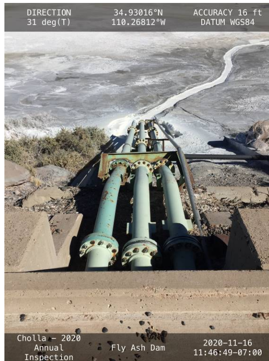
20201116 – IMG_2284 The inlet pipes along the upstream slope.
