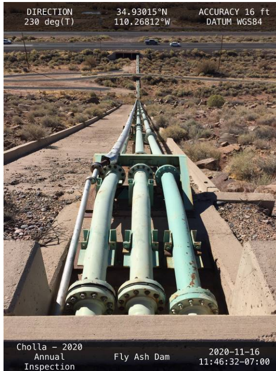
20201116 – IMG_2282 The inlet pipes along the downstream slope.
