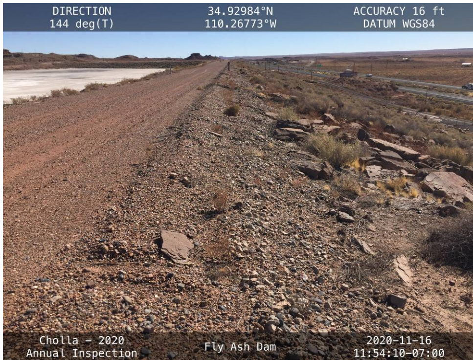
20201116 – IMG_2303 The downstream slope, facing southeast from the Northwest Abutment.
