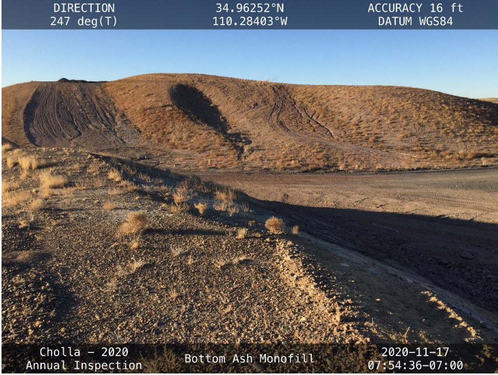
20201117 – IMG_2850 The north side of the Bottom Ash Monofill.
