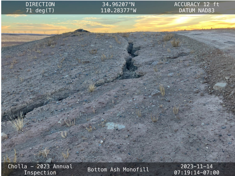
20231114 – IMG_1840 An erosion gully on north side of the BAM, facing south.
