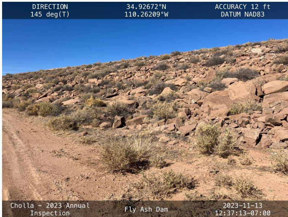
20231113 – IMG_1510 The downstream slope and toe of the South Embankment.
