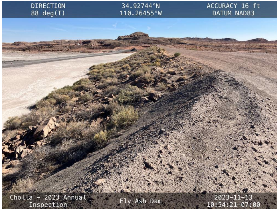
20231113 – IMG_1401 The upstream slope of the South Embankment, facing east.
