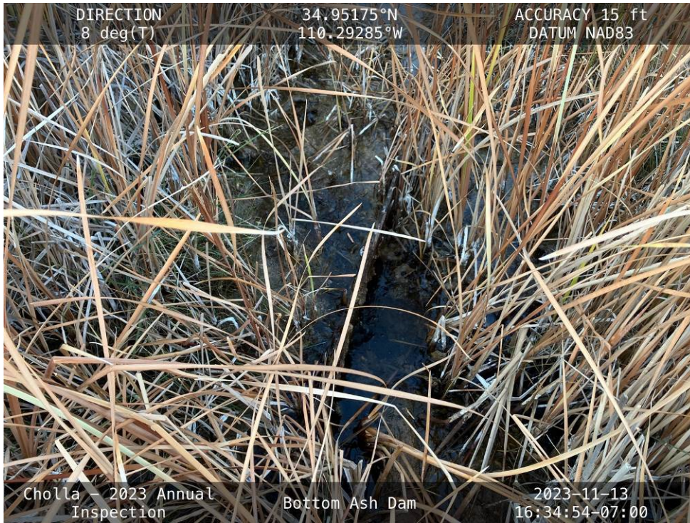
20231113 – IMG_1800 The West Abutment Weir, flowing at approximately 1.72 gpm.
