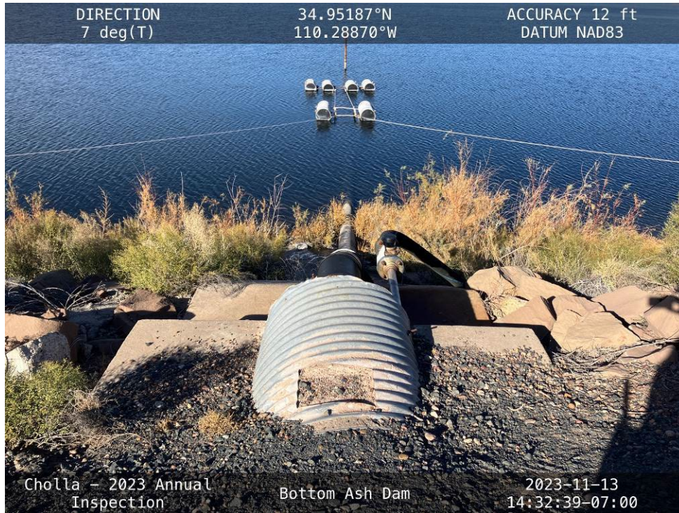
The eastern siphon line along the upstream slope of the South Embankment.
