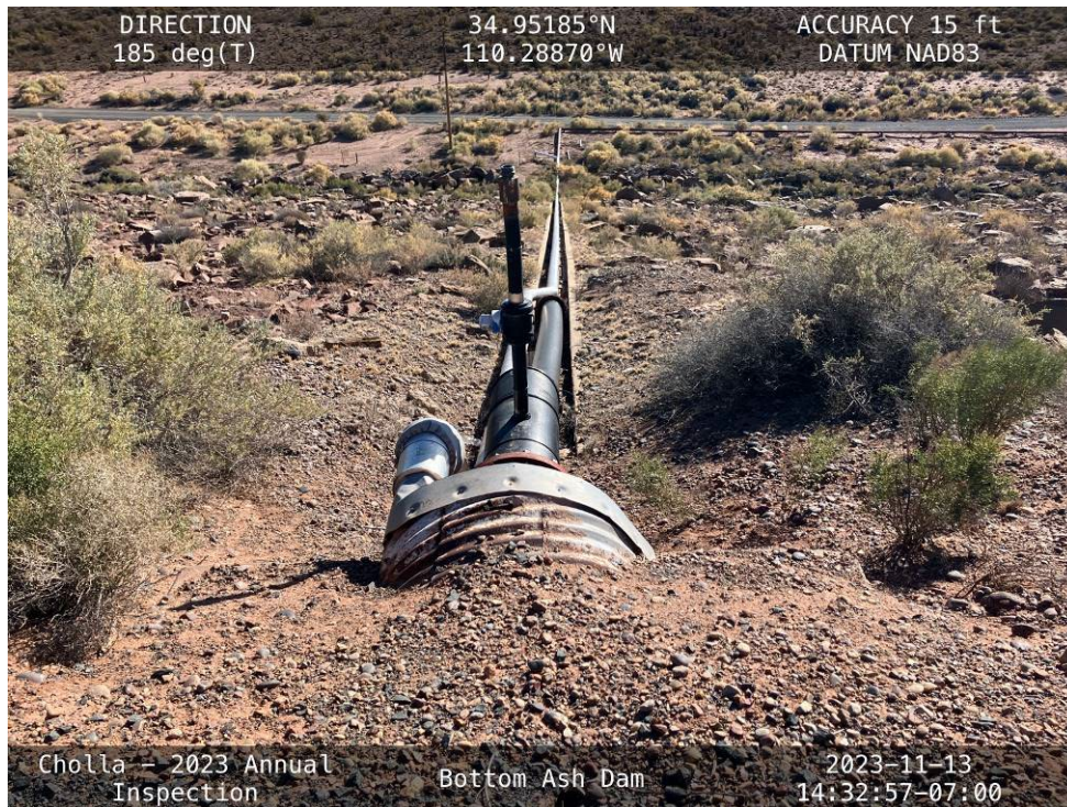
The eastern siphon line along the upstream slope of the South Embankment.
