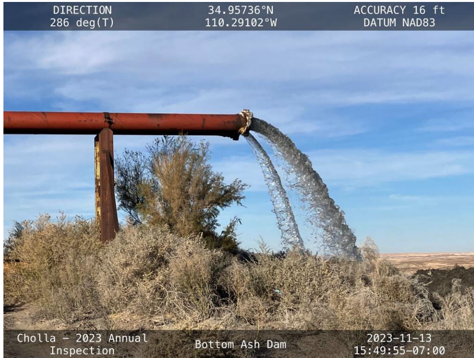
20231113 – IMG_1744 Ash and water being deposited into the Bottom Ash Pond.
