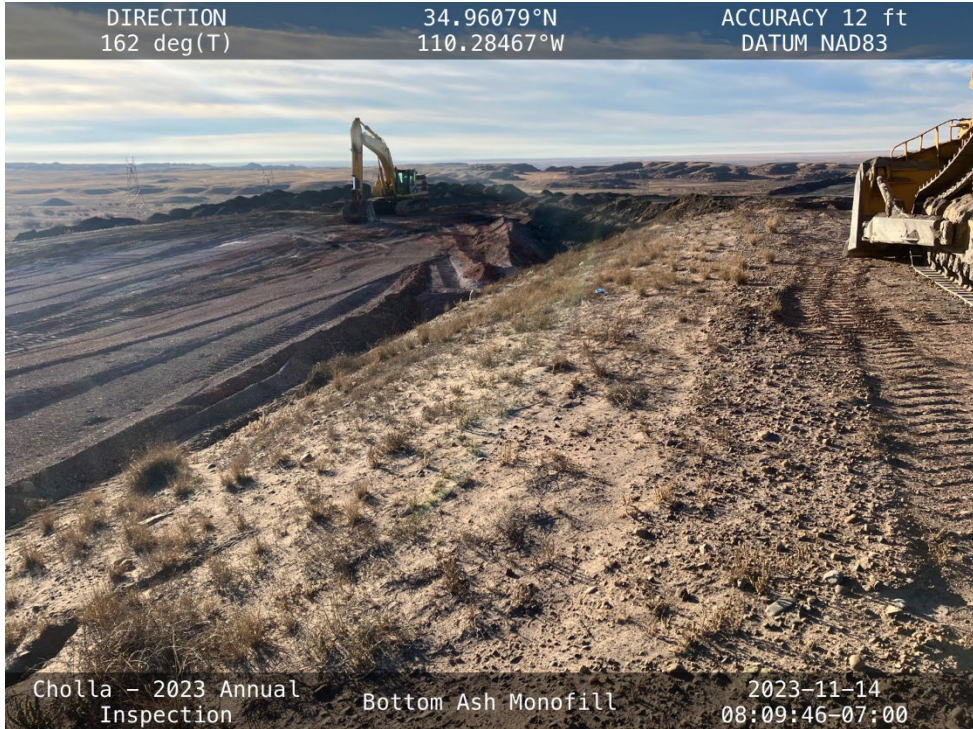
20231114 – IMG_1915 The CCR excavation area on top of the BAM.
