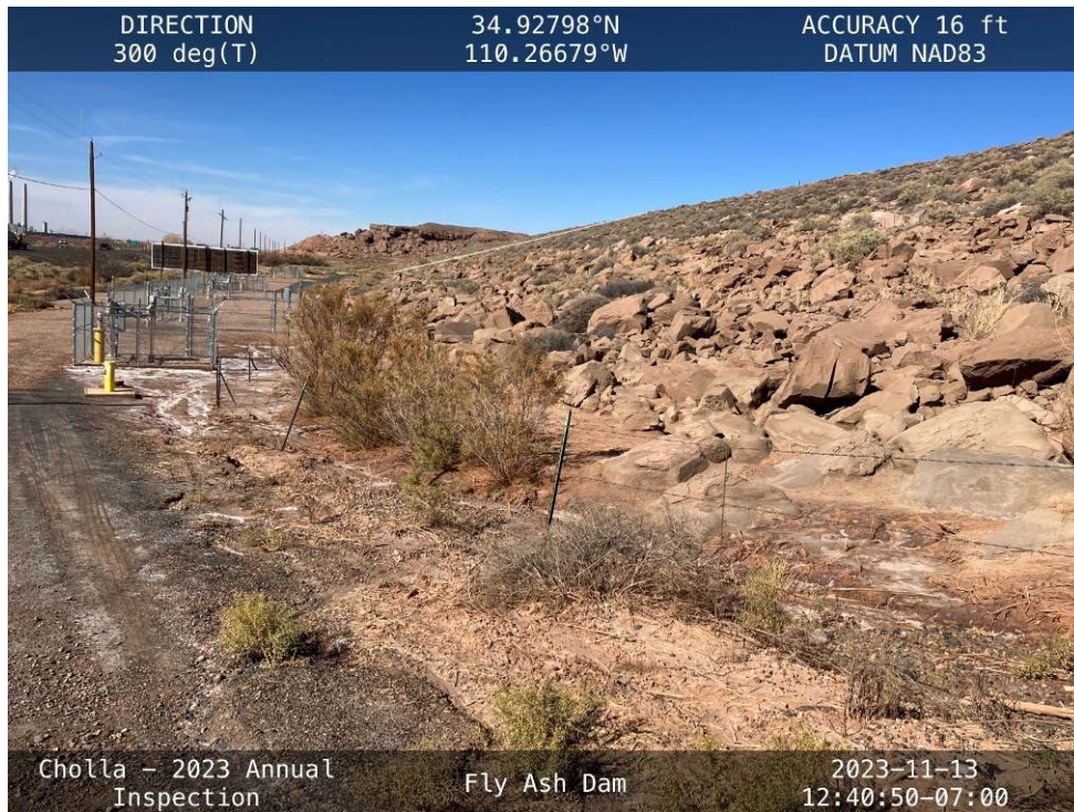
20231113 – IMG_1519 The Geronimo Seep area, with new monitoring wells, fencing, and extraction wells.
