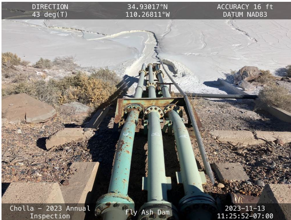
20231113 – IMG_1444 The inlet pipes along the upstream slope.
