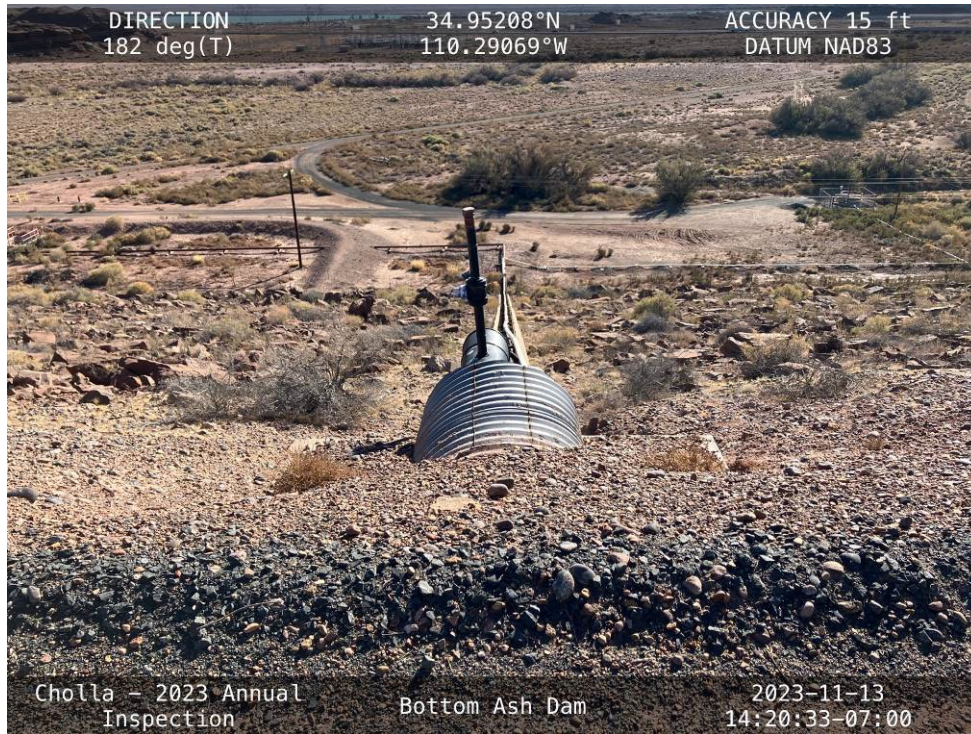
The western siphon line along the downstream slope of the South Embankment.
