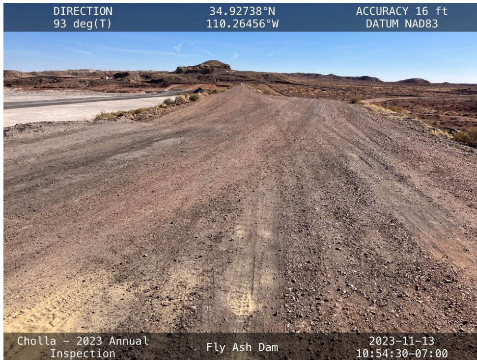
20231113 – IMG_1402 The crest of the South Embankment, facing east.
