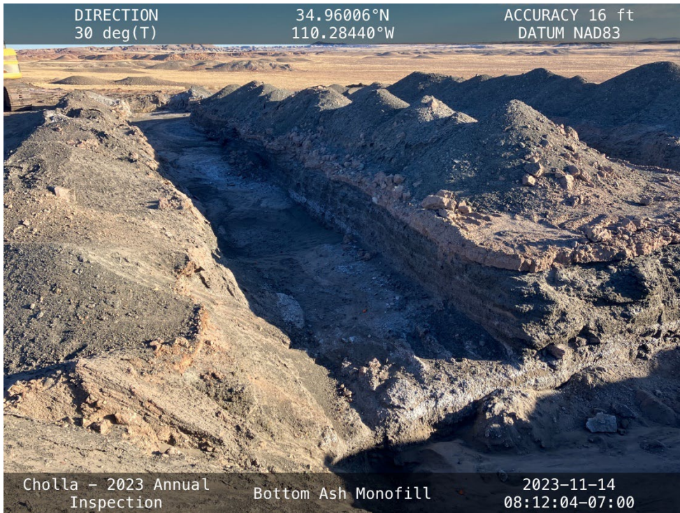
20231114 – IMG_1924 The CCR excavation area on top of the BAM.
