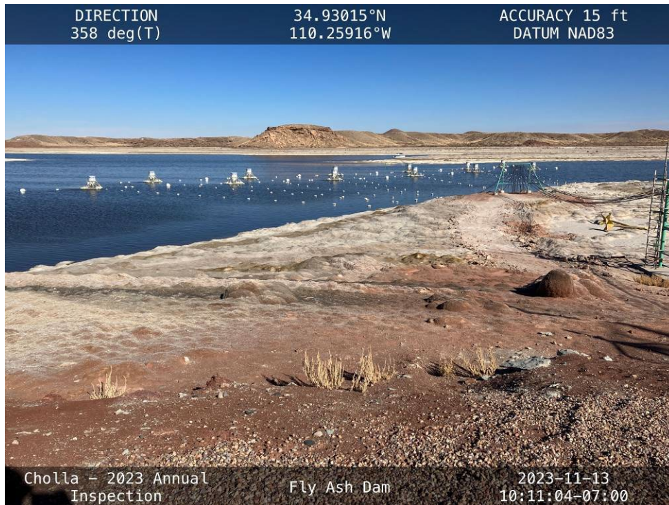
20231113 – IMG_1365 Downdraft evaporators in the Fly Ash Pond.
