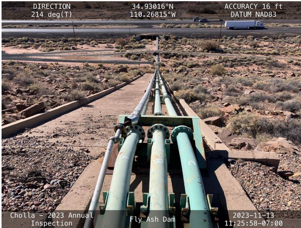
20231113 – IMG_1445 The inlet pipes along the downstream slope.
