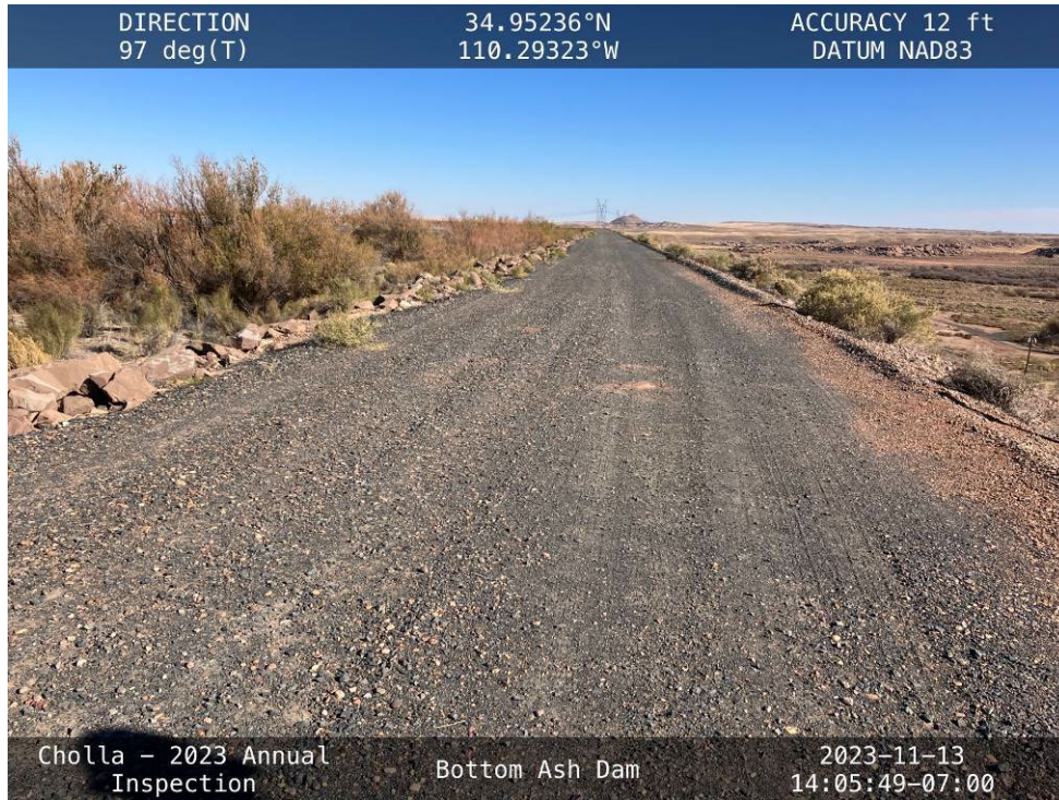
20231113 – IMG_1608 The South Embankment crest, facing east from the Right Abutment.
