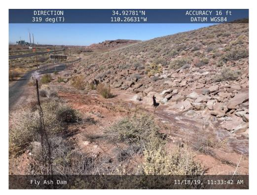
**20191118 – IMG\_5790** Area of historic erosion along the downstream toe of the West Embankment.
