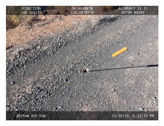
An erosion hole in the crest along the southern half of the East Embankment.
