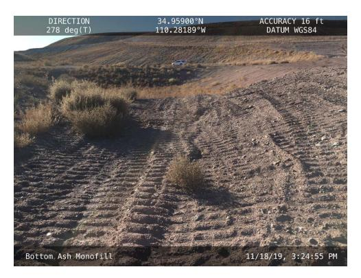
Area of repaired headcutting on the east side of the Stormwater Detention Basin.
