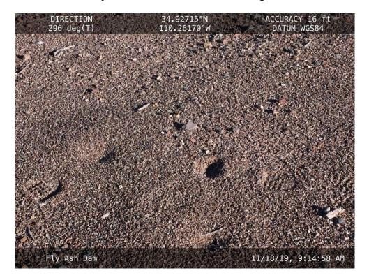
**20191118 – IMG\_5705** Ant hill in the crest of the South Embankment.
