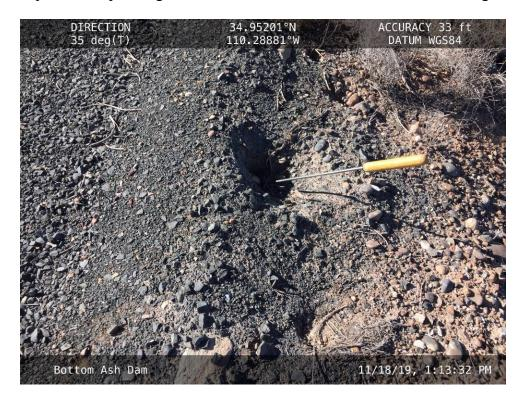
**20191118 – IMG\_5857** An erosion hole on the upstream side of the South Embankment crest.
