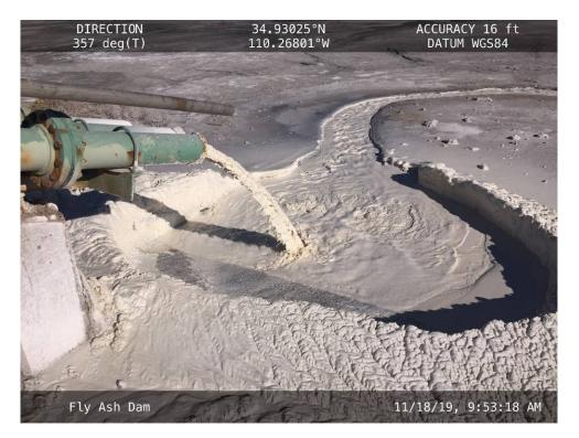
**20191118 – IMG\_5742** The inlet pipe depositing CCR into the impoundment.
