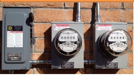
Customer's shall apply NEC 300.3(B): All conductors of the same circuit (including the neutral and ground) shall be contained within the same raceway, conduit, gutter, cable tray, etc..
