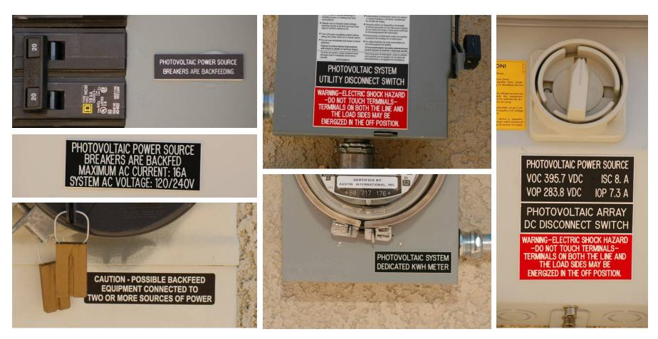
*NOTE:* Typical APS Equipment Labels Handout is located at <u>www.aps.com/dg</u>. ANSI color standards may be used, but is not required by NEC or APS.
