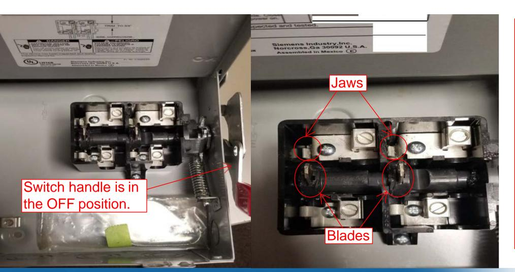
The photographs above depict the switch in the OFF (open) position. The blades and the jaws are not in contact with each other and are separated by an air gap prohibiting the flow of current through the switch.
