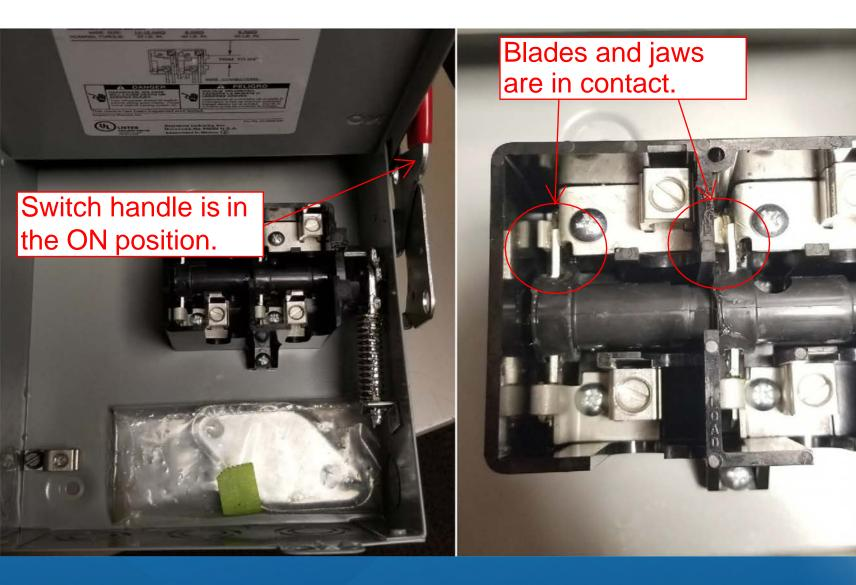
The photograph depicts the switch in the ON (closed) position. The blades and the jaws are in contact with each other and current can flow through.
