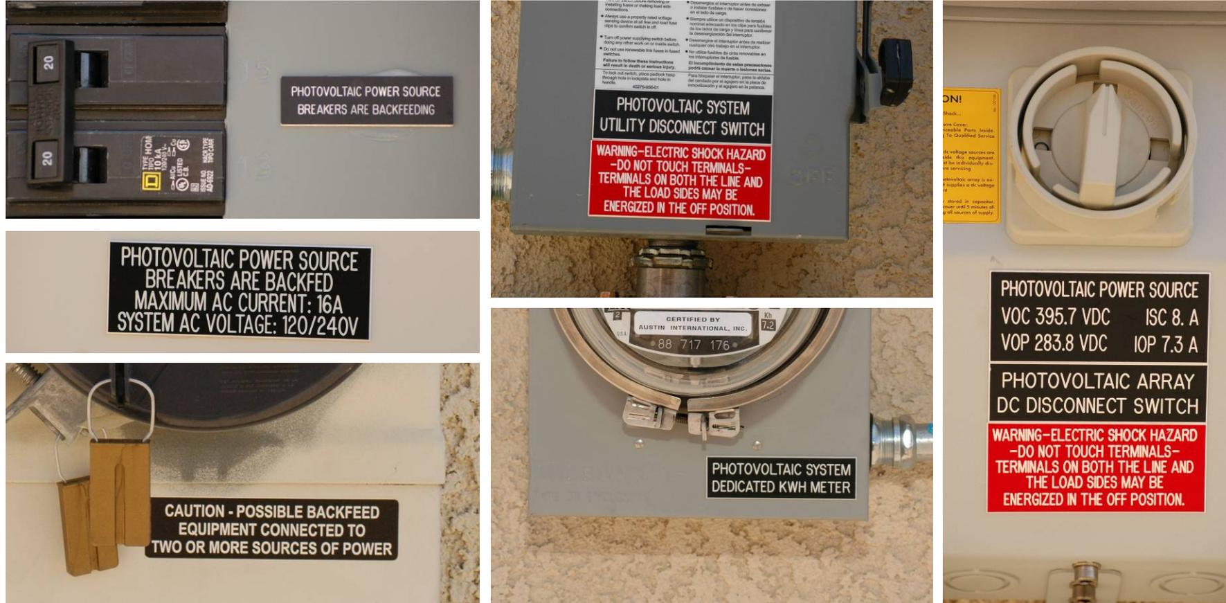
**NOTE:** Typical APS Equipment Labels Handout is located at [www.aps.com/dg](http://www.aps.com/dg). ANSI color standards may be used, but is not required by NEC or APS.
