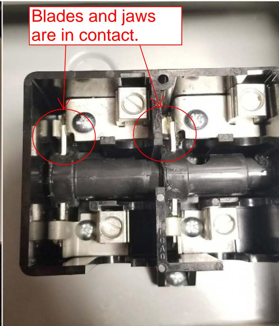
The photograph depicts the switch in the ON (closed) position. The blades and the jaws are in contact with each other and current can flow through.
