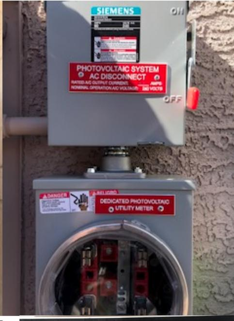
**PHOTOVOLTAIC SYSTEM DEDICATED KWH METER**
