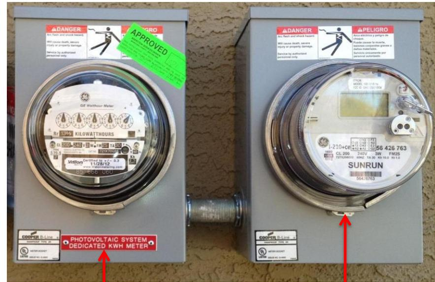
APS Production Meter labeled "Photovoltaic System Meter" or "Photovoltaic System Dedicated kWh Meter."
