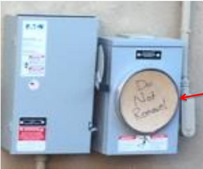
**NOTE: Cardboard is not an acceptable cover material.** Cover material shall be fiberglass, plastic, glass or Plexiglas.
