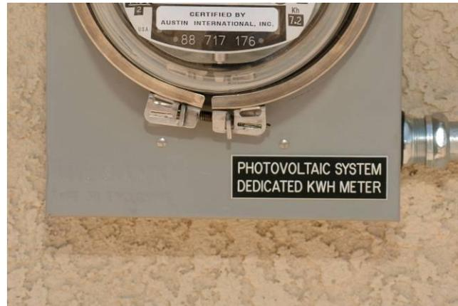
**NOTE:** Typical APS Equipment Labels Handout is located at [www.aps.com/dq](http://www.aps.com/dq). ANSI color standards may be used, but isn't required by NEC or APS.
