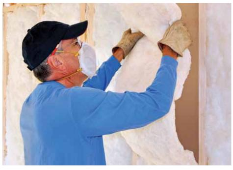
Installers take care to ensure insulation fits correctly with no gaps or voids.
