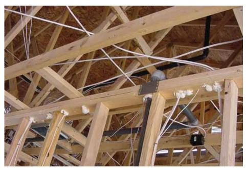
In an ENERGY STAR home, holes created for wiring or plumbing are tightly sealed.
