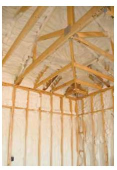
Insulation completely blankets the home and is inspected before the drywall goes up.
