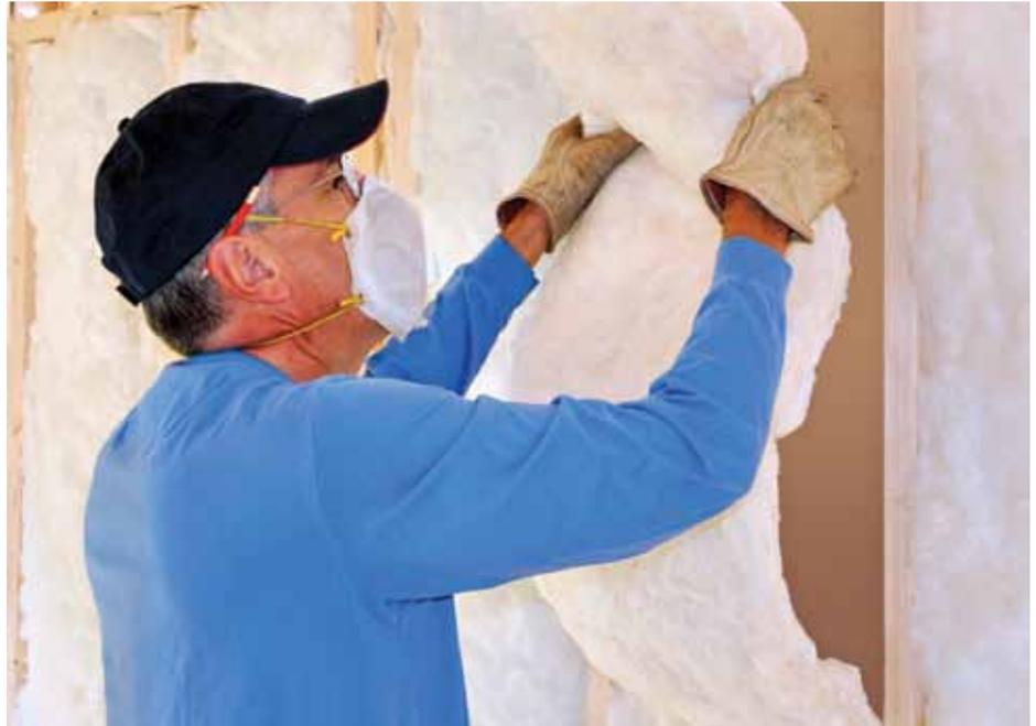
Installers take care to ensure insulation fits correctly with no gaps or voids.
