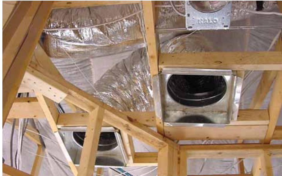
"Jump ducts" ensure adequate air flow from room to room.
