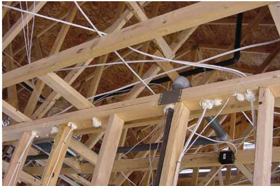
In an ENERGY STAR home, holes created for wiring or plumbing are tightly sealed.
