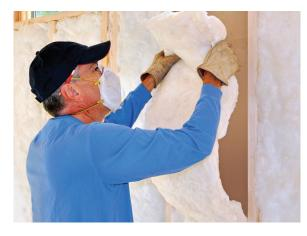
Insulation completely blankets the home, making full contact with the air barrier and filling every void, so air cannot leak through.
