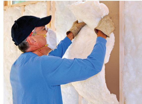
Insulation completely blankets the home, making full contact with the air barrier and filling every void, so air cannot leak through.
