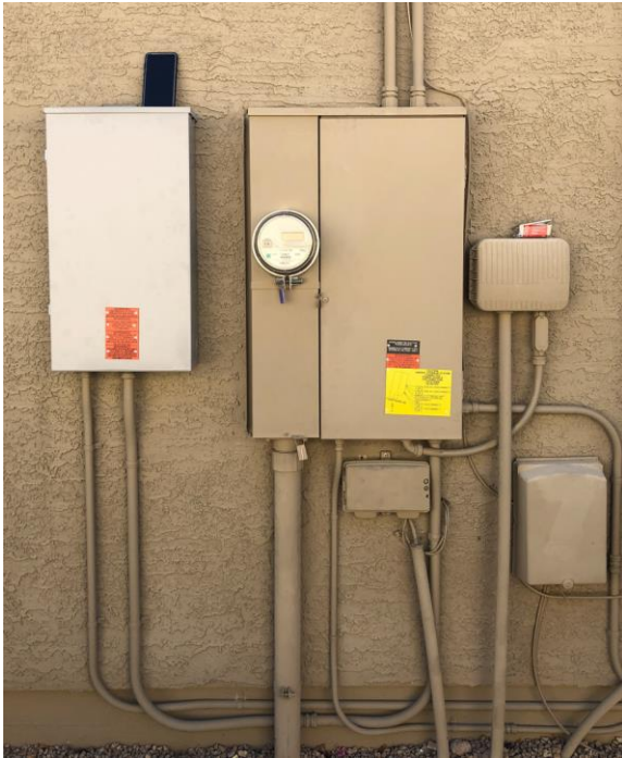
Figure 1 – Location of Backup Load Panel
