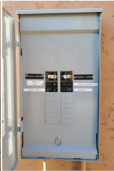
Figure 2 –Backup Load Panel
