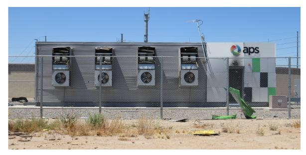
Figure 7 The side door to the McMicken BESS was ejected in the explosion and can be seen laying against the fence in the foreground
