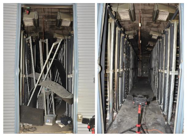
Figure 9 Interior damage to the energy storage system with the condition after the explosion (left), and condition after debris was removed to gain access to the interior and begin the forensics analysis (right)
