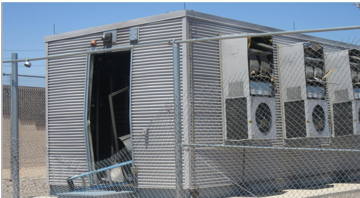
**Figure 6 Damage to the rear door and HVAC systems of the McMicken BESS**
