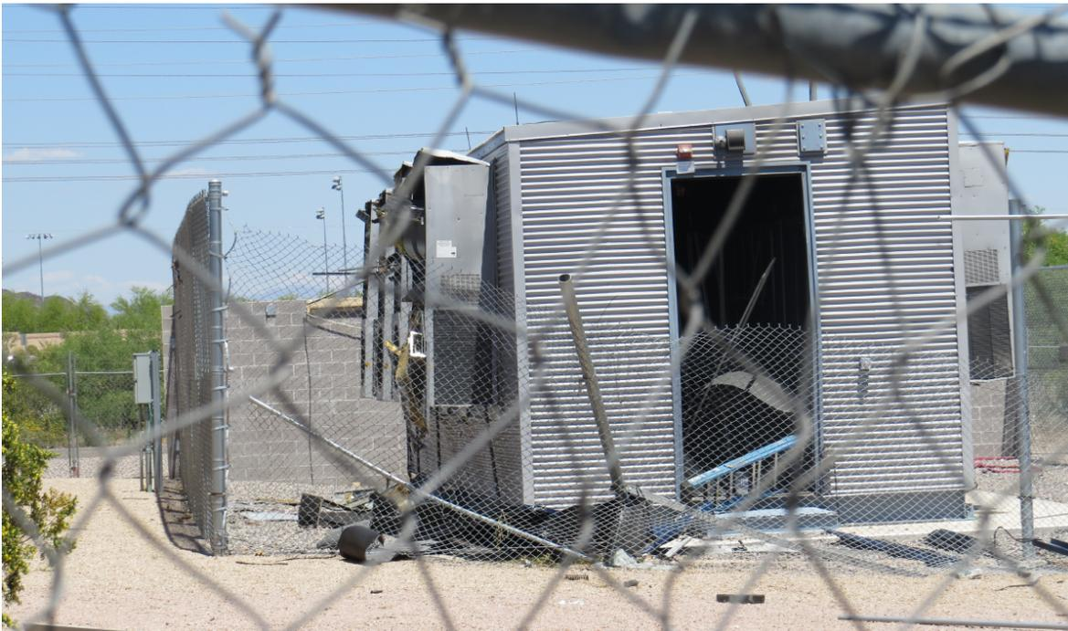
**Figure 8 Additional view of debris and damage to the rear door, HVAC systems, and the container**
