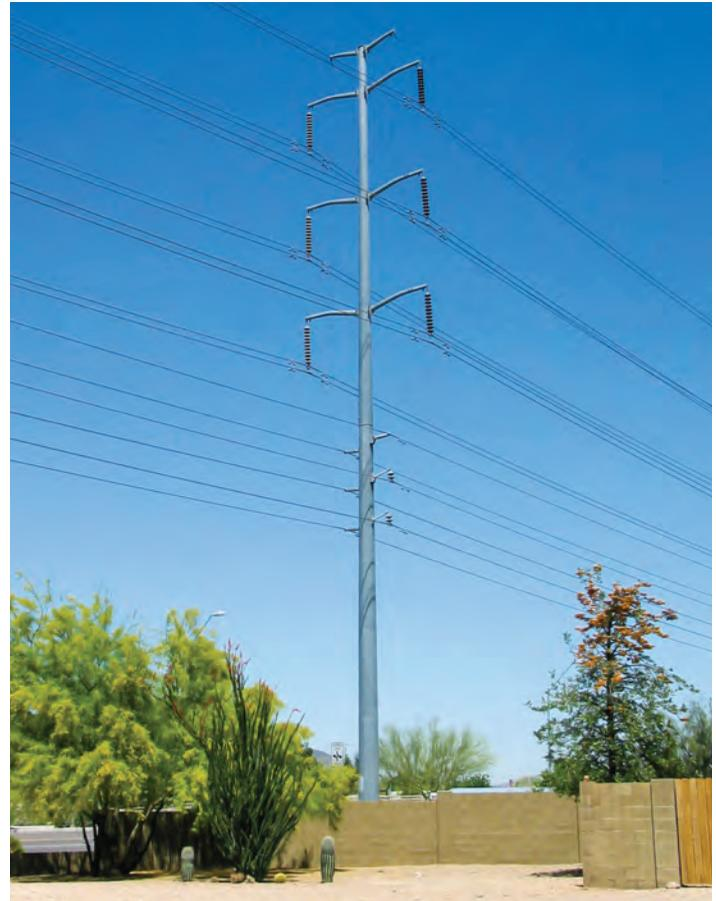
230kV transmission line pole example
