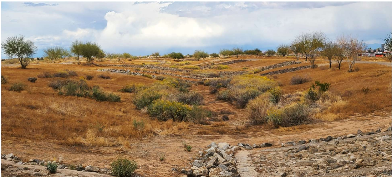
Class B – Reems Road Channel Flood Control Facility
