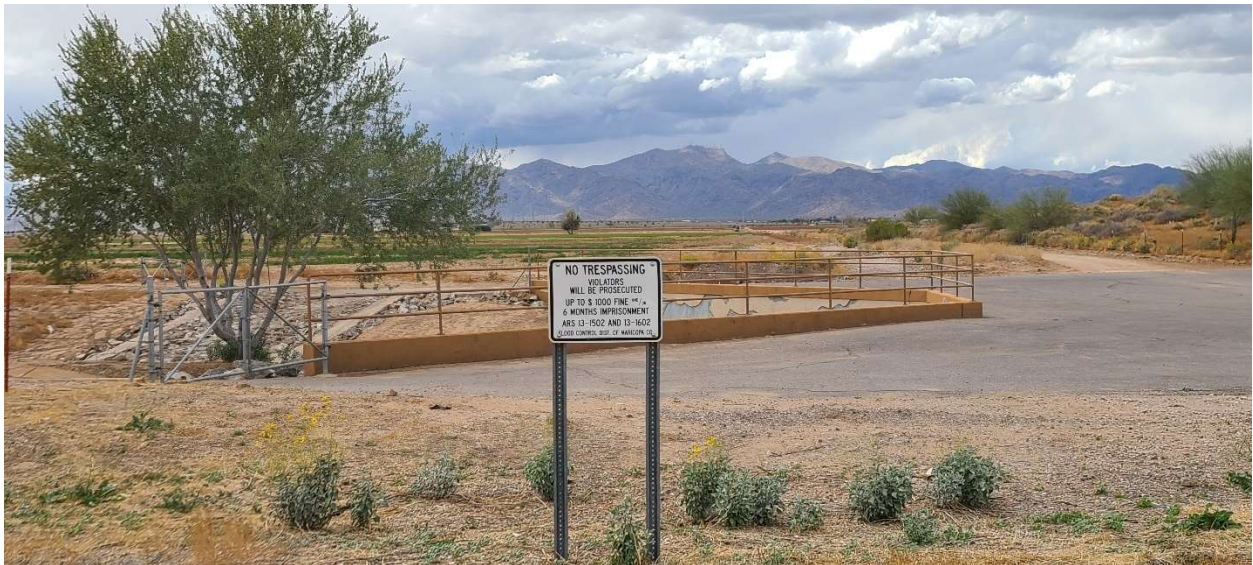
Reems Road Flood Control District Facility
