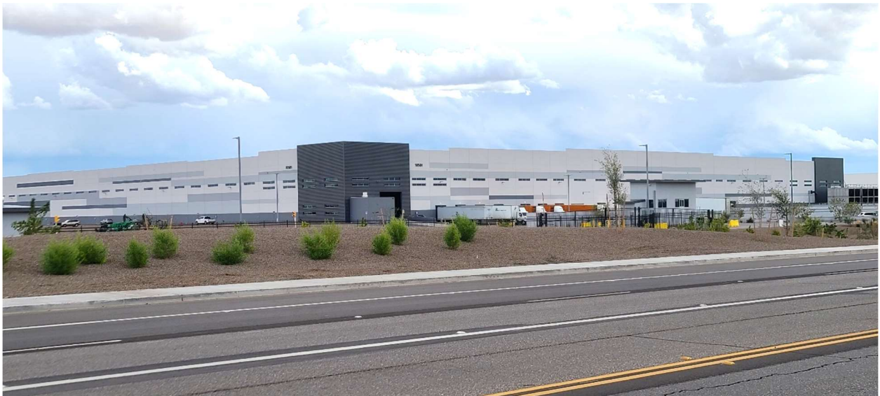
Light Industrial Development
