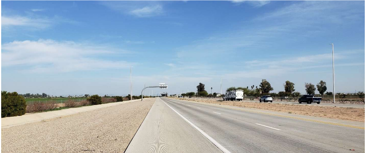
Northern Parkway Freeway
