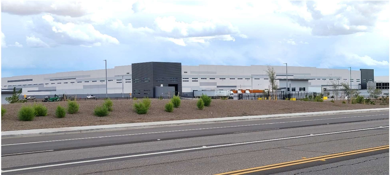
Light Industrial Development
