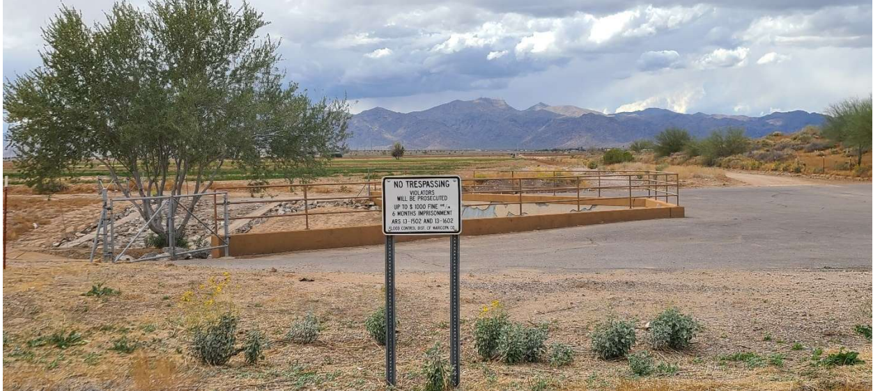
Reems Road Flood Control District Facility
