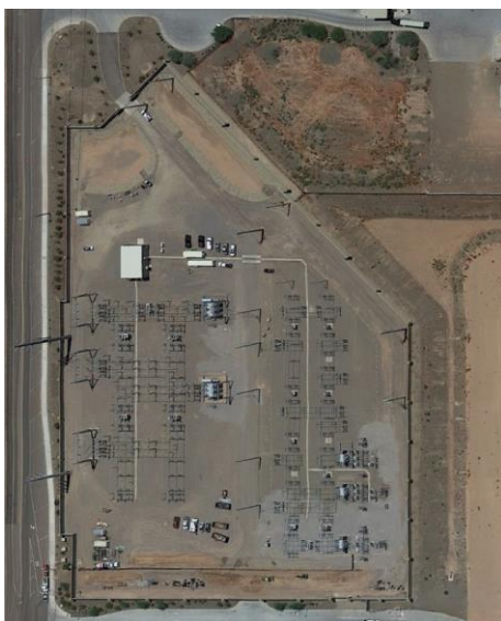
230/69kV Substation – Aerial View
