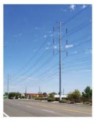
230kV Double Circuit with 69kV Double Circuit Underbuild
