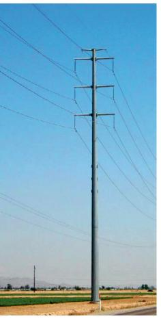
Typical 230kV pole with future 69kV capability
