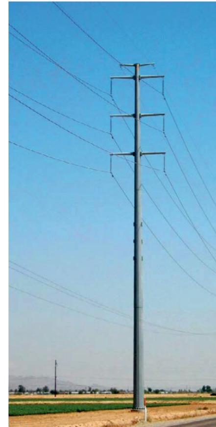
Typical 230kV pole with future 69kV capability
