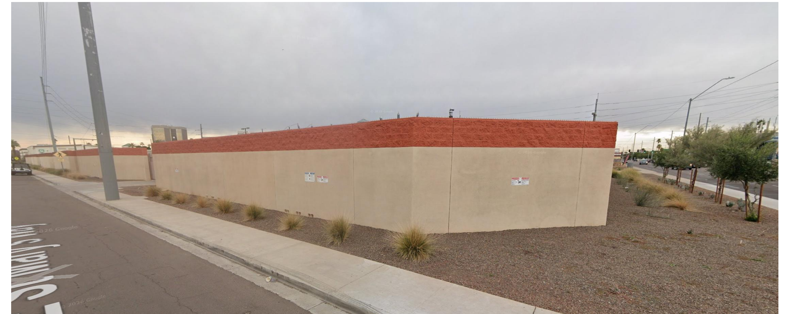
Sample of Substation Block Wall (future Helios)
