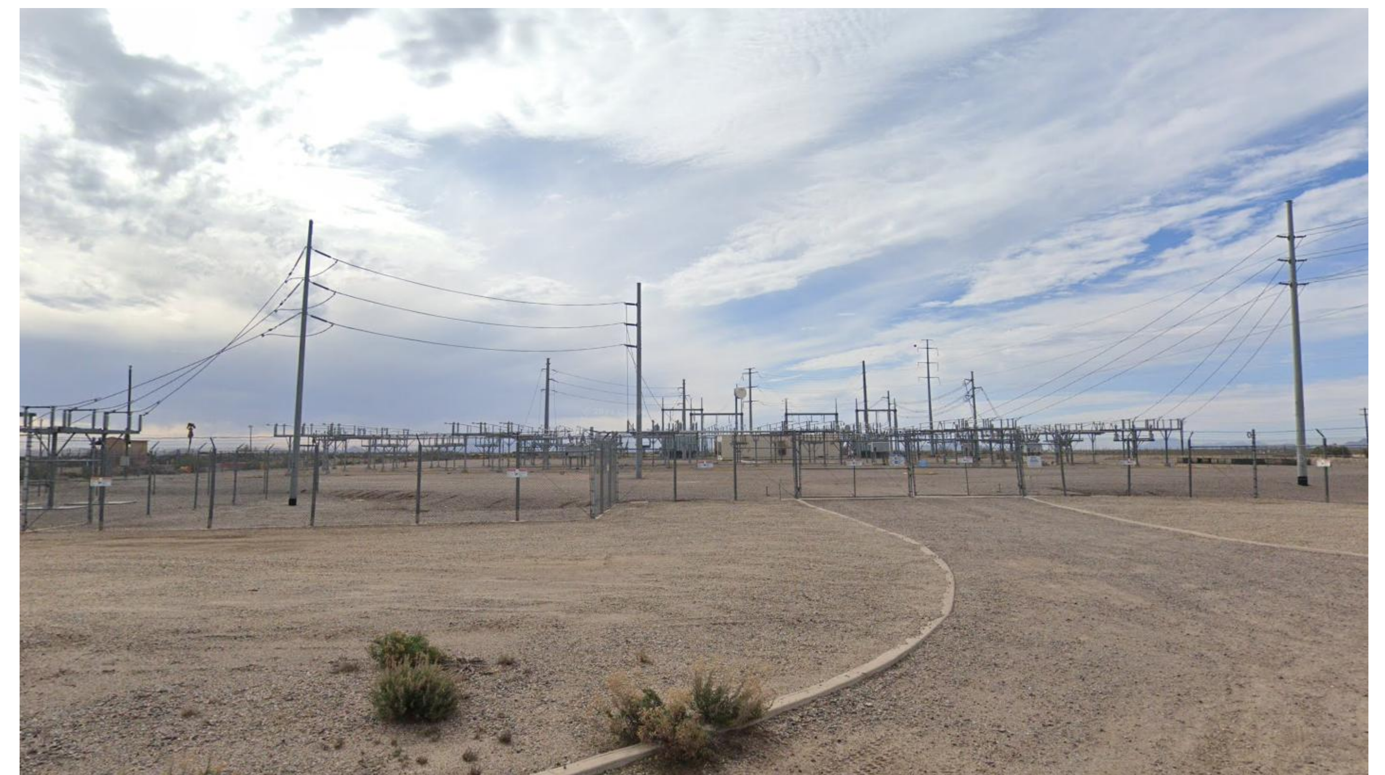
Milligan Substation (existing)
