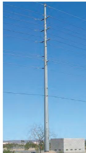
Typical 69kV double-circuit pole (left) and typical 69kV double-circuit pole with 12kV underbuild (right)
