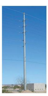
Typical 69kV double-circuit pole (left) and typical 69kV double-circuit pole with 12kV underbuild (right)
