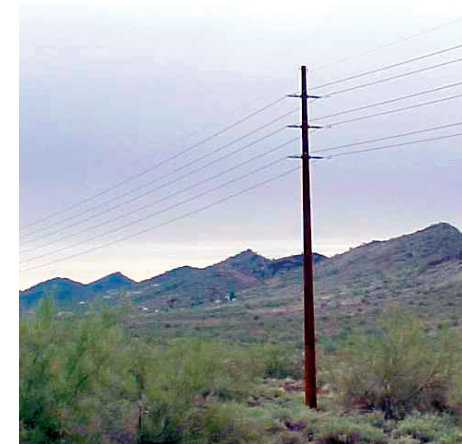
Double Circuit 69-kV Self-Weathering Steel Pole Structure
