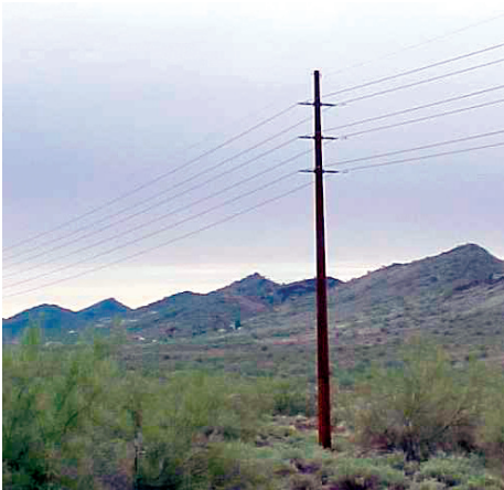
Double Circuit 69kV Self-Weathering Steel Pole Structure
