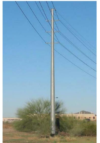
Typical 69kV double-circuit poles
