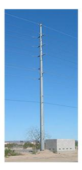
69kV Double-Circuit Monopole with 12kV Underbuild
