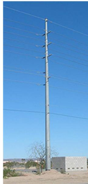
69kV Double-Circuit Monopole with 12kV Underbuild
