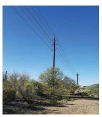
Typical 69kV double-circuit pole
